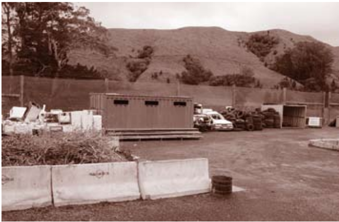
Above: Matawai transfer station has areas for greenwaste, recyclable materials, whiteware and tyres.
