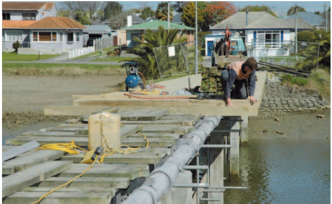
As strengthening work takes place underneath the Hall St footbridge, James Kissling (Fulton Hogan) builds the new deck on top.
