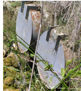
Floodgates on culvert
