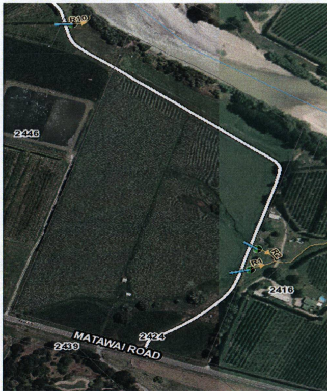
Image 2 – Aerial photograph showing the location of the stop bank (Identified with a white line).
