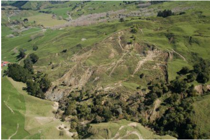
Figure 9 Isolated slump with stream undercutting along the toe slope contributing a small amount of sediment to the stream channel with most of the displaced material remaining on-slope.
