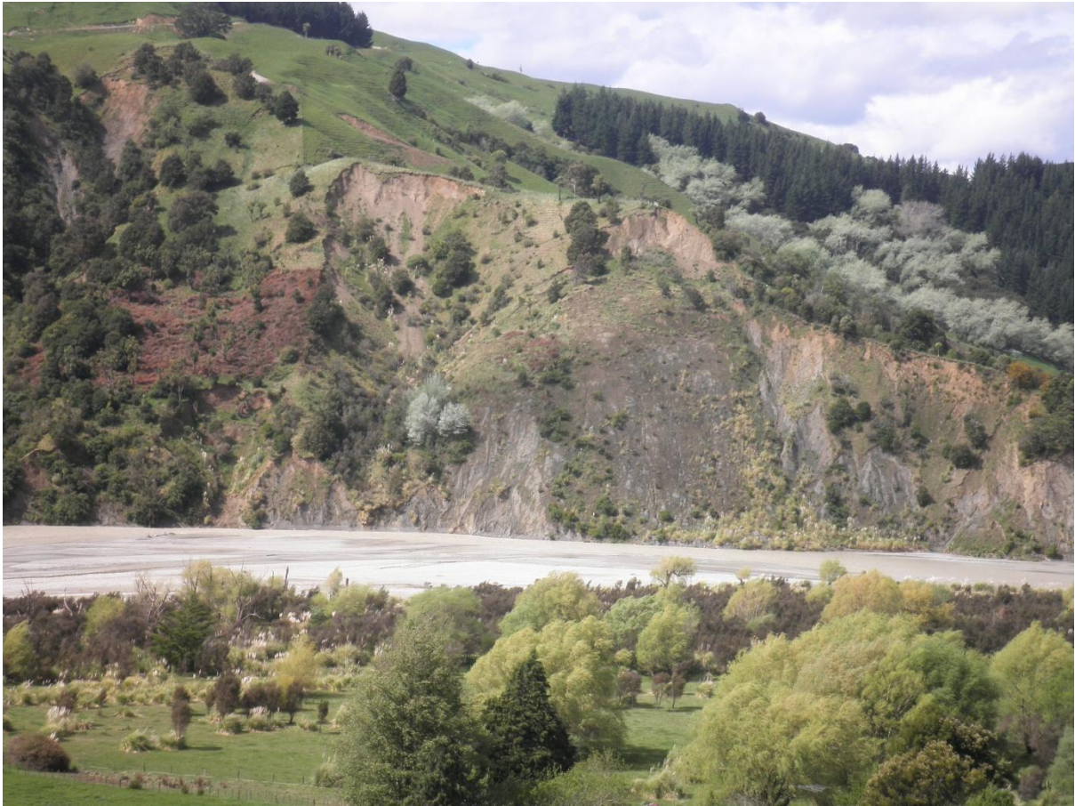
Figure 6 Undercut bedrock cliff resulting in the slumping of sediment directly to the channel (photograph courtesy of Gisborne District Council).
