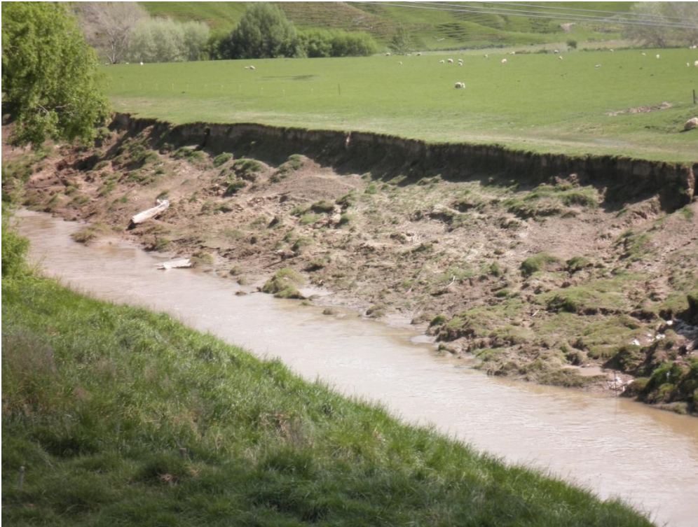
Figure 7 Bank consisting of unconsolidated alluvium that likely failed after flood waters receded (photograph courtesy of Gisborne District Council).
