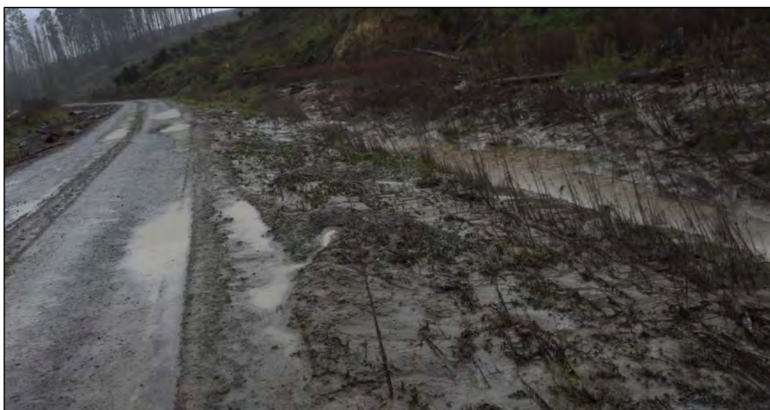
Image_0116. Mangatoitoi forestry road showing silt deposition from flooding and scattered logs.
