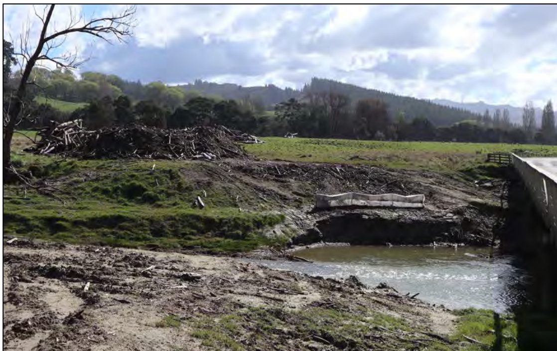
Poorly configured silt fence installed at Wigan Bridge.
