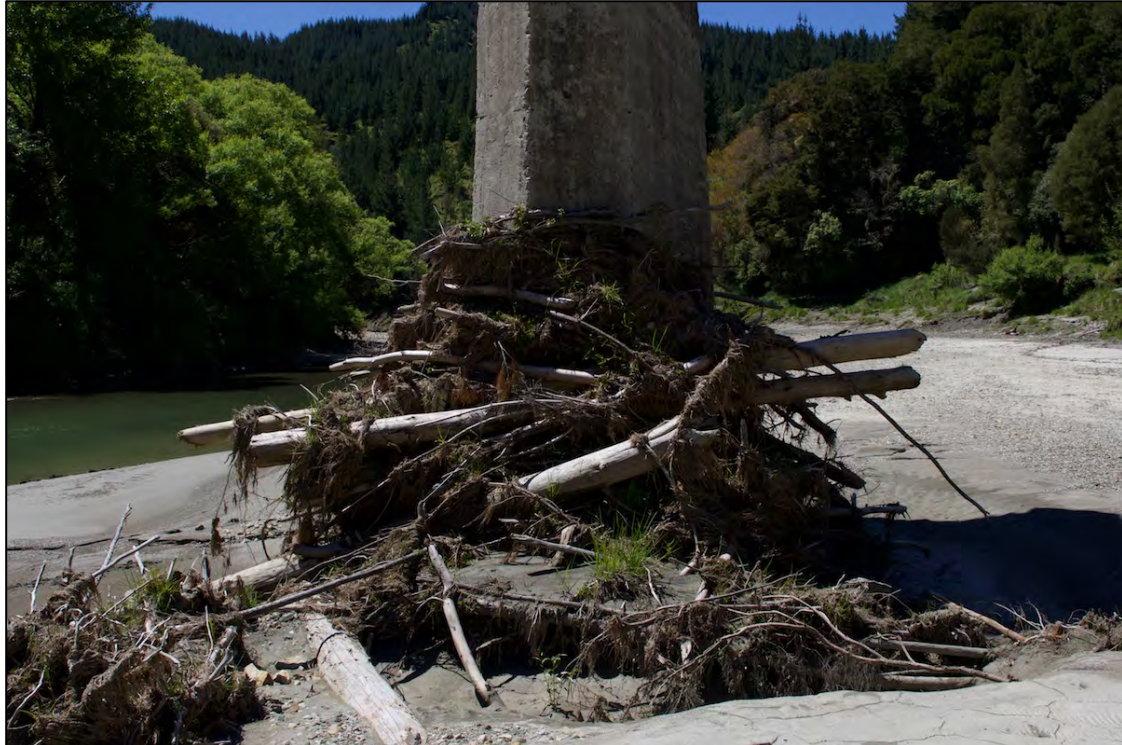
Image 1D1A4221. View of pine and cross woody debris caught up in old bridge pile Ihungia.
