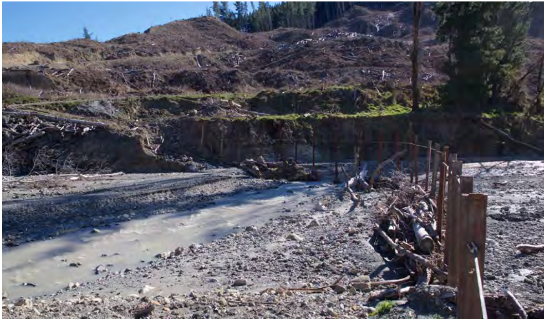
New slash catcher installed at Whakoau Stream showing new logs including cut logs caught against catcher
