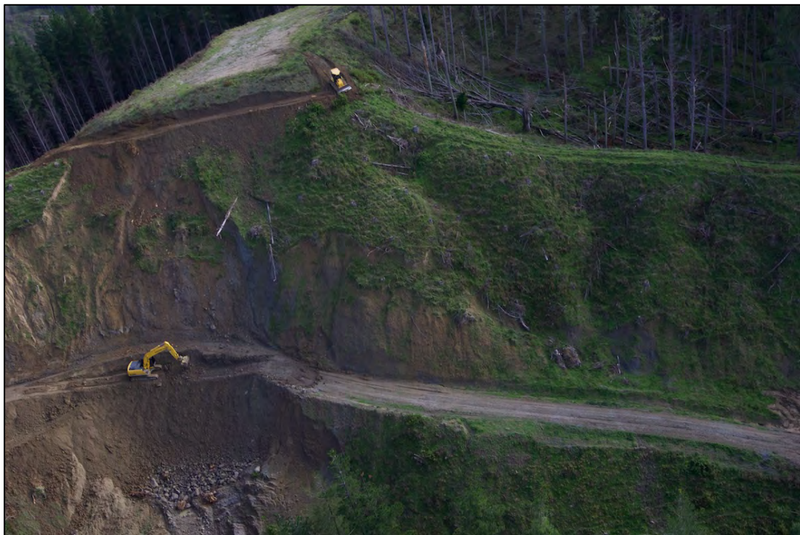
Image 1D1A0983. Forestry roadworks and slip clearing between Mangateao and Mangatoitoi streams, Tauwhareparae Road.
