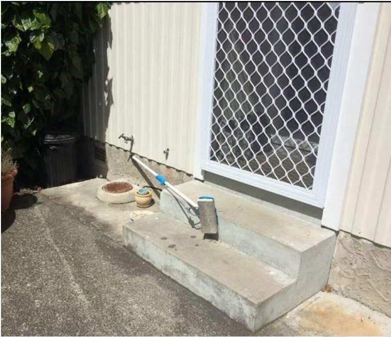
Figure 3-3 Height of Flooding During the Same Event (indicated by the mop)
