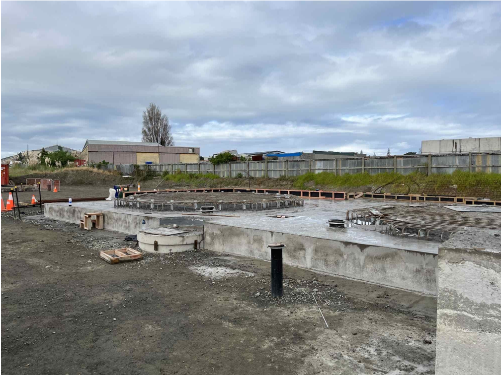
Sludge storage tank slab initial pour completed.
