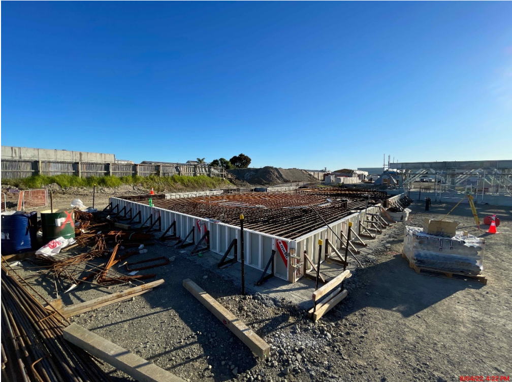
Sludge storage tank slab being constructed.
