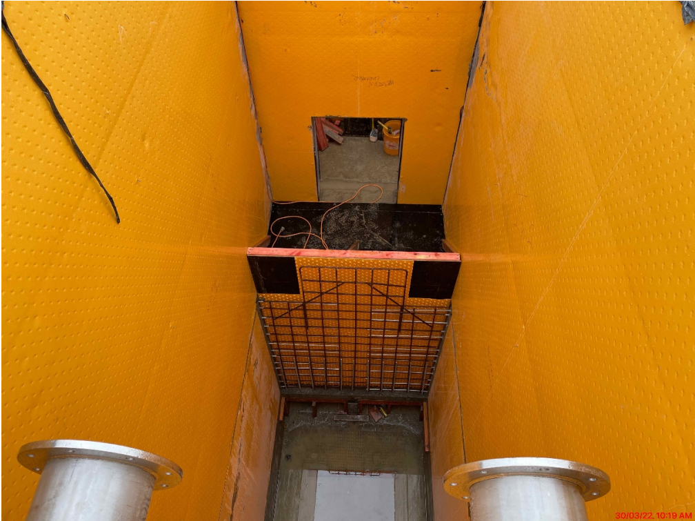
Reinforcing steel for internal wall within clarifier pump station.
