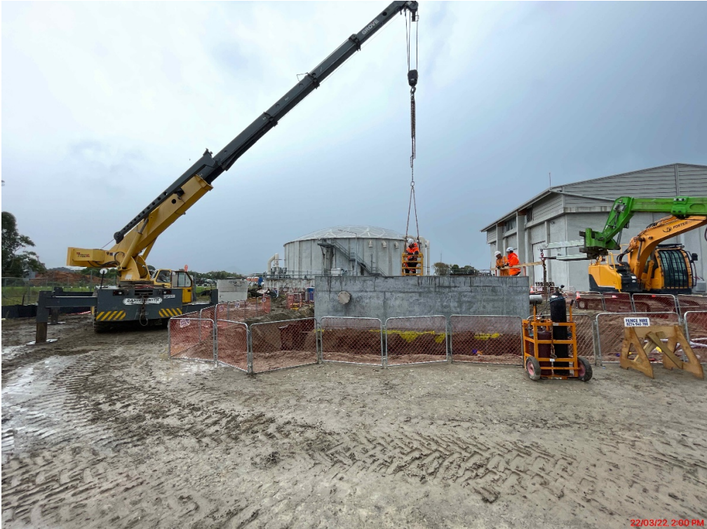
Crane access for inspections of clarifier pump station internal walls work.
