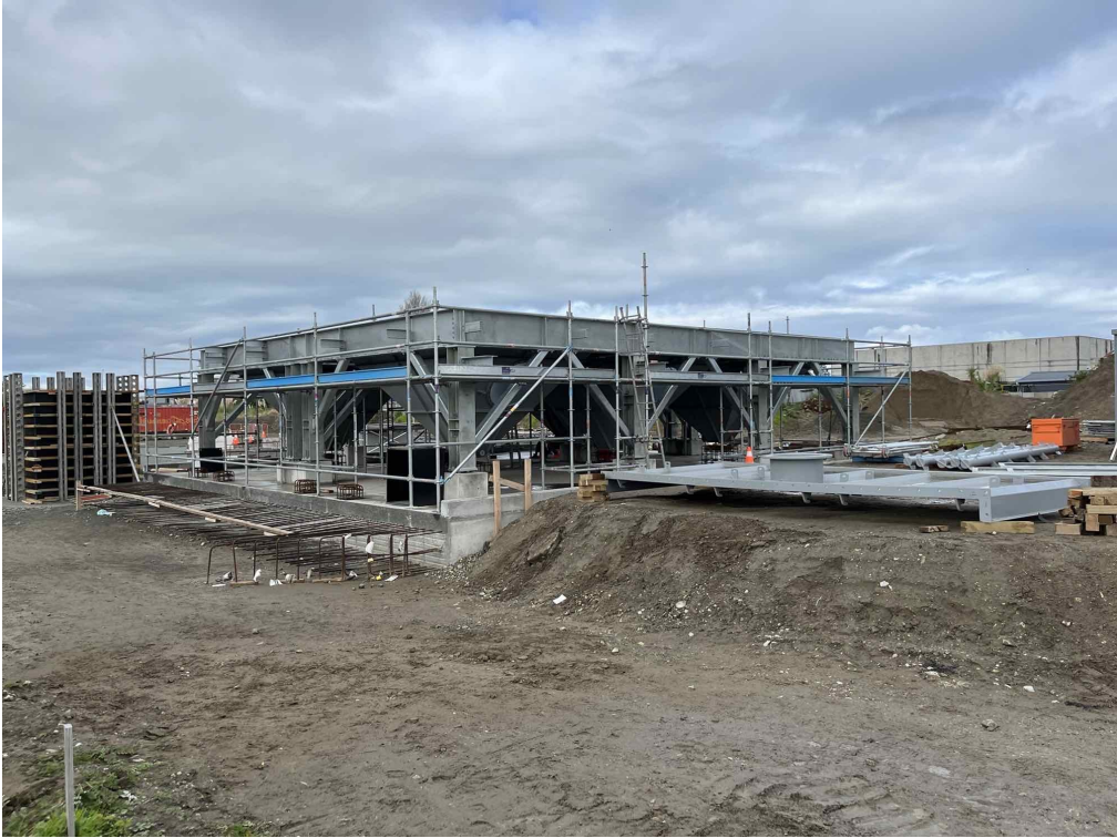
Lamella clarifier hopper bases installed into frame.
