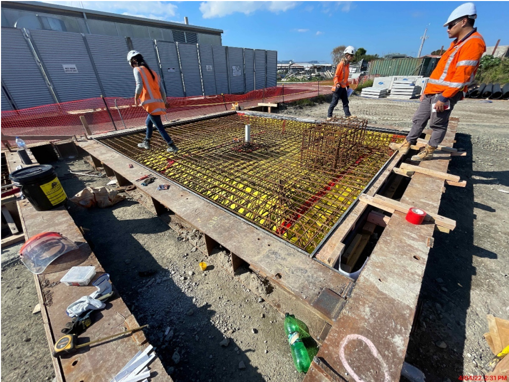
Reinforcing steel for pump shed slab in place.
