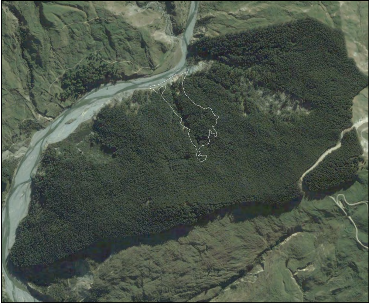
Figure Forty Four. Satellite image of the site of the landing failure that occurred in the Waitahaia River between 21 st May 2020 and 8 th of August 2020. This shows the outline of the slope failure that occurred during the storms of July 2020 with signs of the earlier slope failure marked by an area of poor growth. Other areas of instability with poor pine cover are evident on either side of the 2020 failure.
