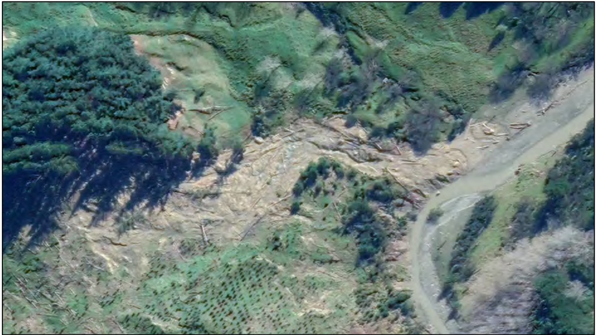
Figure Sixty Four. Satellite image dated 8 th August 2020 showing a large slope failure on recently replanted slope that has shed a large volume of logs to the Whakoau Stream at Bremnar bridge.
