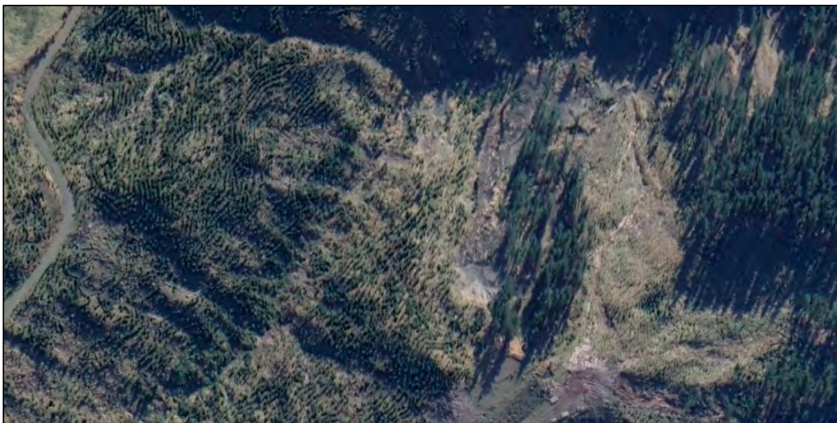
Figure Forty Seven. Satellite image dated 13 th of July 2018 showing a recently activated landslide on the lefthand side of the landing and a debris flow on the righthand side. Note mature pine left standing below the landing.
