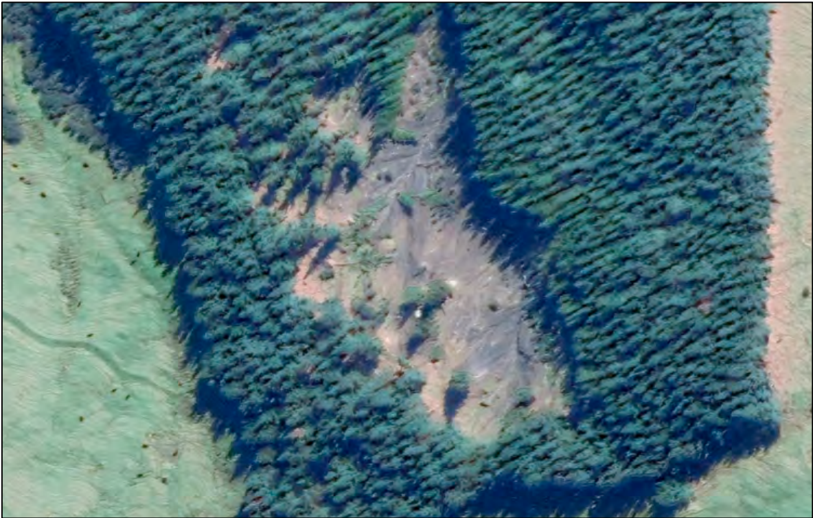
Figure Sixty One. Satellite image of gully WTR3 in the Waitahaia River dated 8 th of August 2020 showing trees that have collapsed from the eroding headscarp on the left of the gully.
