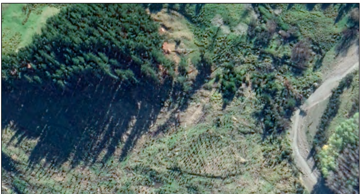
Figure Sixty Five. Satellite image of the Whakoau Stream immediately downstream of the Bremnar Bridge dated 21 st May 2020 showing the pre-failure presence of harvest residues on the slope.
