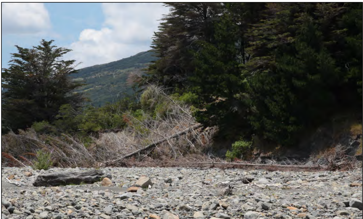
(Figure Seventy) Photograph of collapsed pine tree resulting from river bank scour (toe failure). Tapuaeroa River immediately upstream of Pakihiroa Bridge (6 th January 2021).
