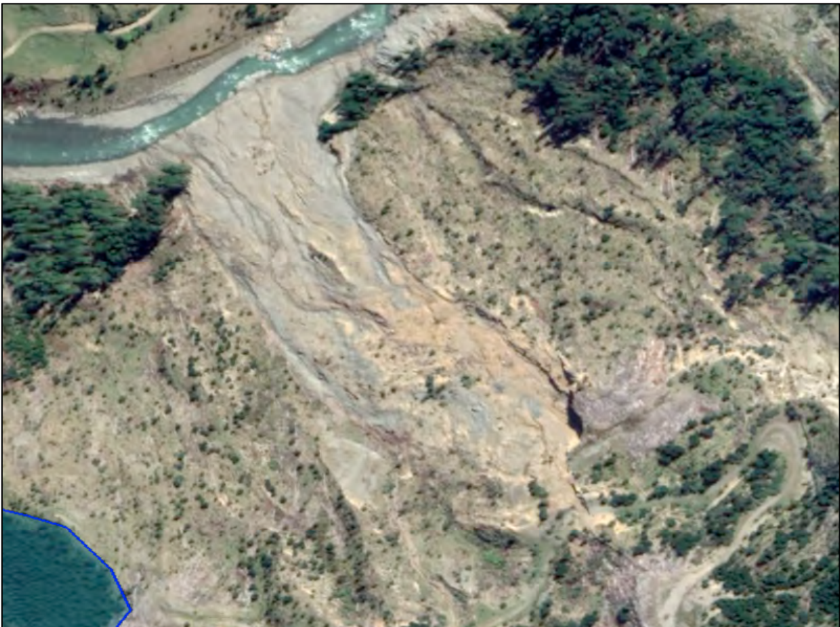
Figure Forty Three. Satellite image of the same landing in the Waitahaia River dated 8 th August 2020 showing the collapse of the landing with a significant slope failure to river level.
