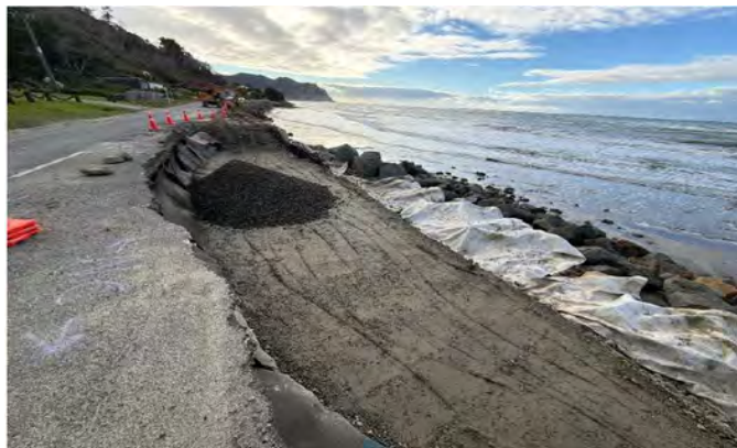
COUNCIL - 25 June 2026 Tokomaru Bay sea wall site 4 (after digout)
