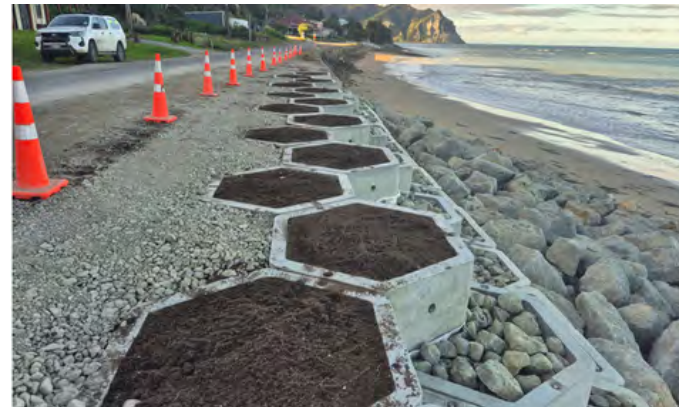
Tokomaru Bay sea wall site 4 (complete)
