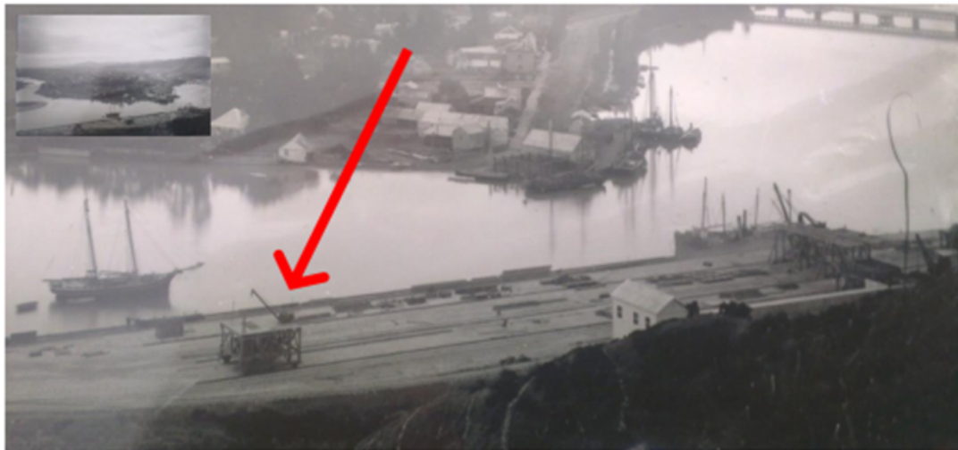
Fig. 7 Extract image of blockyard in 1887 showing the one of the two crane structures on rails (indicated) and the larger gantry crane under construction at the right (full image inset) (‘Gisborne from Kaiti Hill’, WFC 102.2/59, Tairāwhiti Museum)
