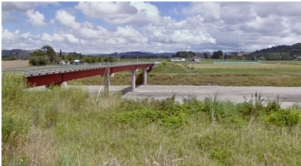
Figure 8. Kanakanaia bridge over the Waipaoa River looking west towards Te Karaka (2010).
