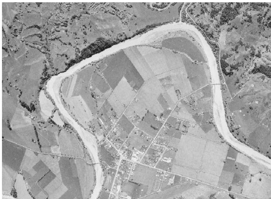
Te Karaka in 1969 after flood scheme built.
