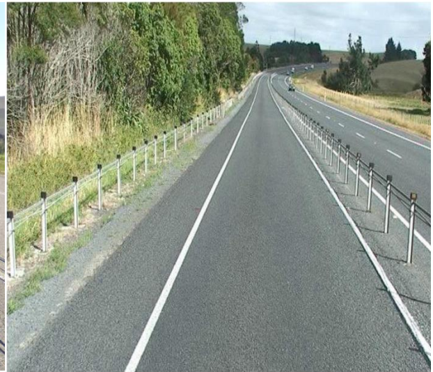
Figure 3-11: Median and roadside barriers on State Highway 1 (Source: NZTA)
