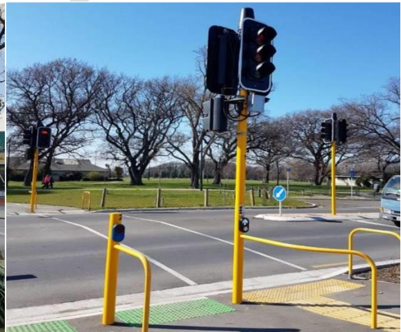
Figure 3-9: An example of safe pedestrian and cyclist crossing with signals (Source: NZTA)
