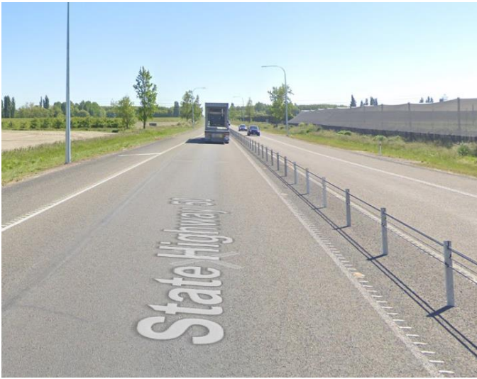
Figure 3-10: Median barriers and white audio tactile markings on State Highway 2 (Source: Google map)
