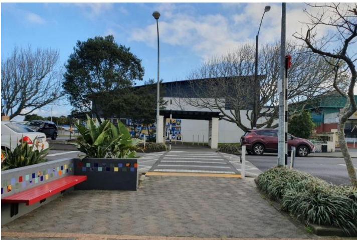
Figure 3-8: An example of raised platform (Source: Auckland Transport)
