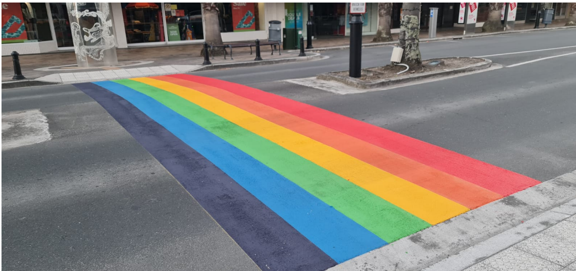
Business as usual maintenance works across the network have been progressing. Below is an example of footpath maintenance undertaken on Patrick St.
