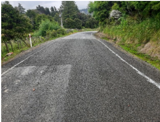
Waipiro Road stabilising work sealed
