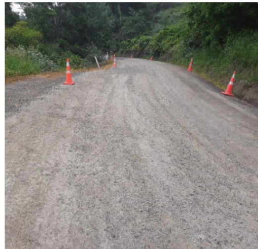
Waipiro Road stabilising work ready for sealing
