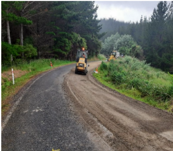
Waipiro Road stabilising prep work
