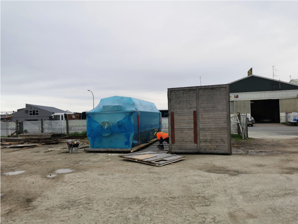
Arrival and unboxing of tertiary filters on site.
