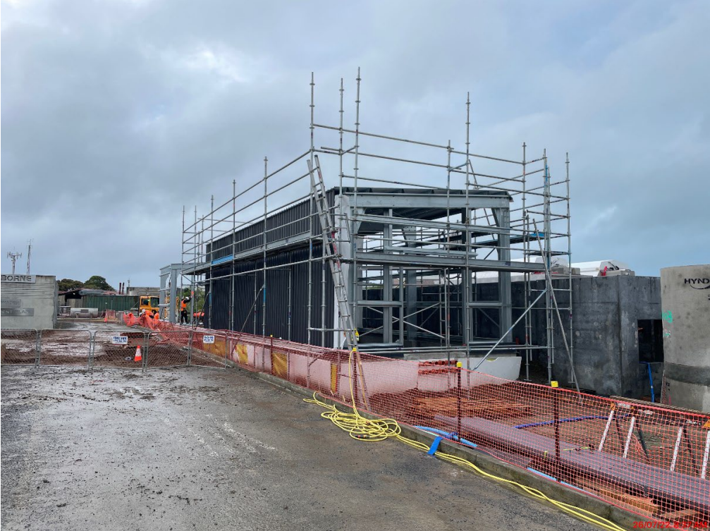
Electrical building construction.
