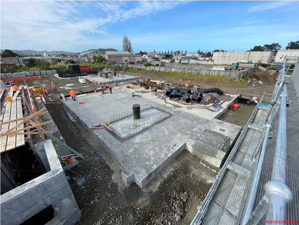
Progress of the tertiary filtration slab construction.
