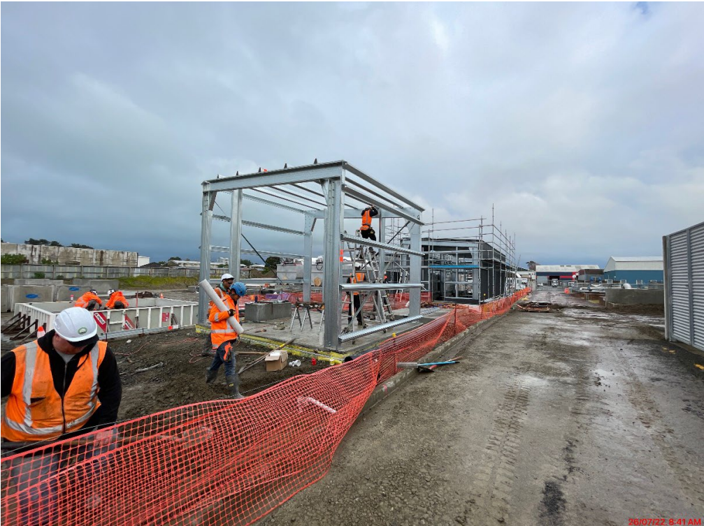
Pump shed building construction.
