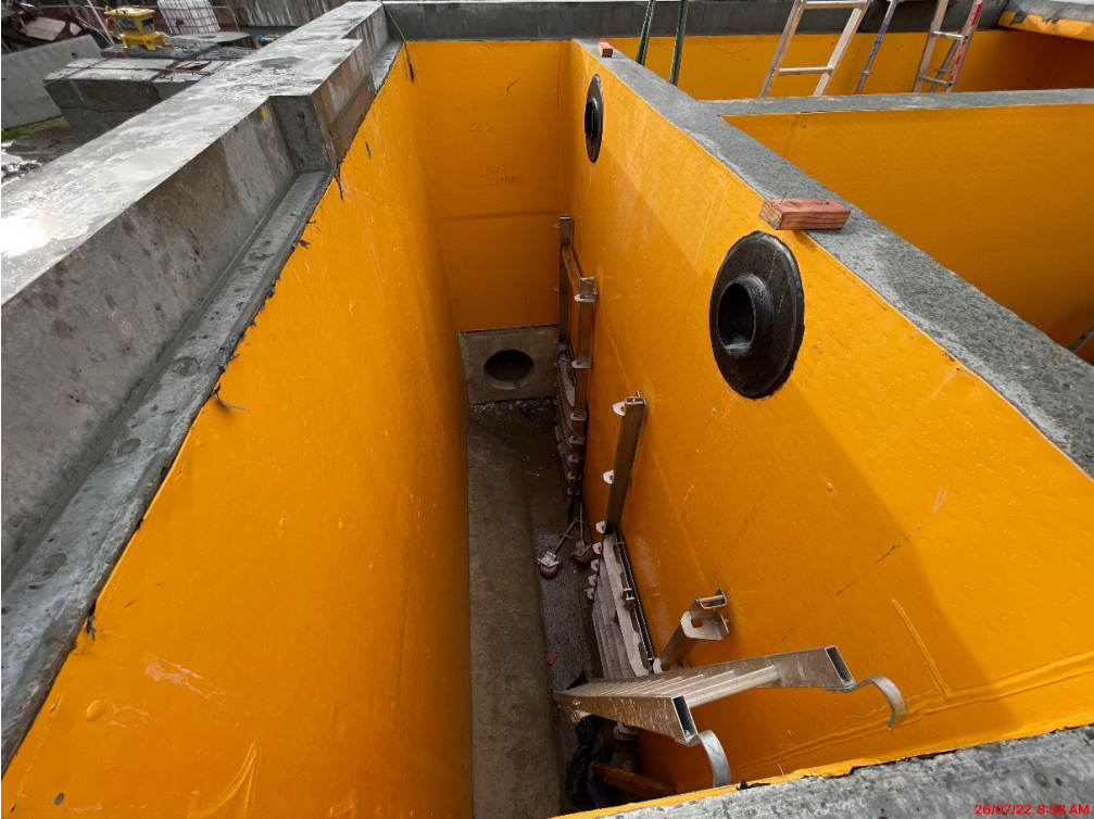
Penstock installation in clarifier pump station inlet chamber.
