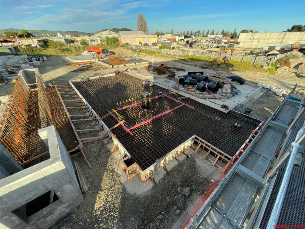
Progress of the tertiary filtration slab construction.
