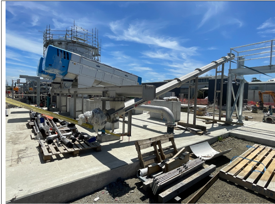
Screw conveyors installation from the screw presses.
