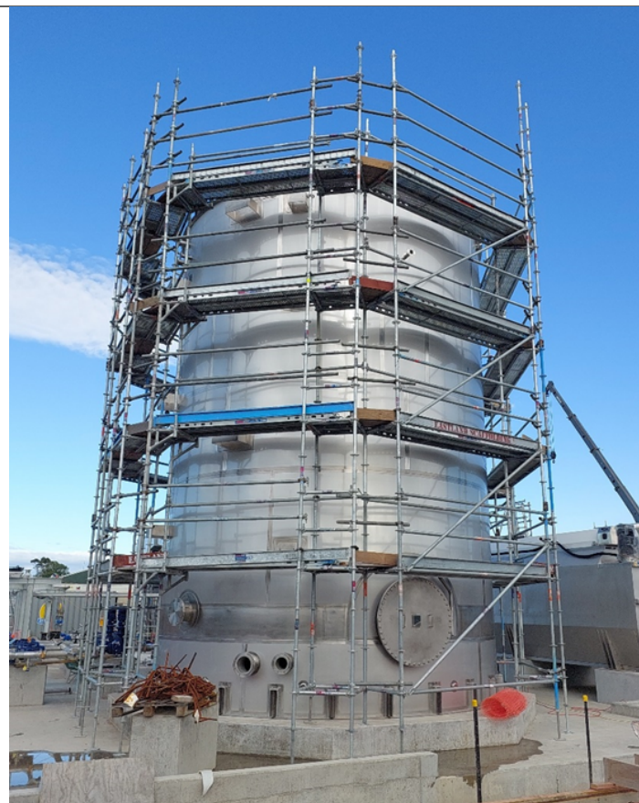
Scaffolding erected around sludge storage tank
