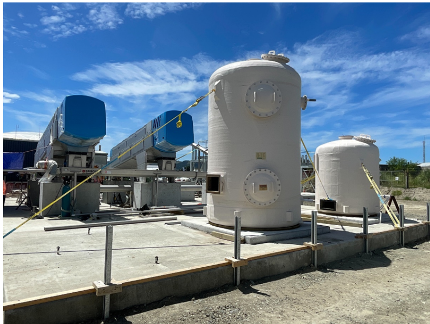
Placement of the odour control vessels
