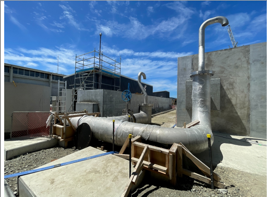
Large stainless-steel pipework fabrication at the flow splitter/UV
