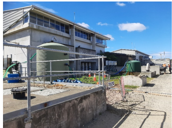
Smaller green tank fed from dewatering spears
