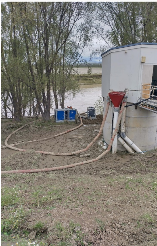
Overland pumping water for treatment
