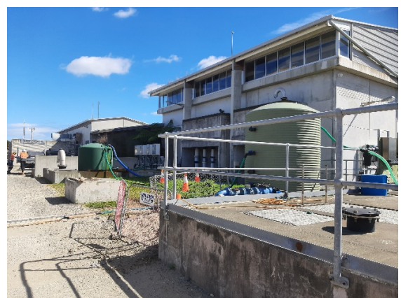
Feed tank 1 and 2 with hose to the screen room water tank
