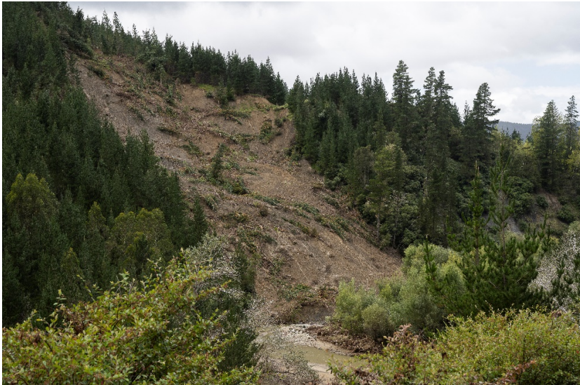
Example of a slip across the road
