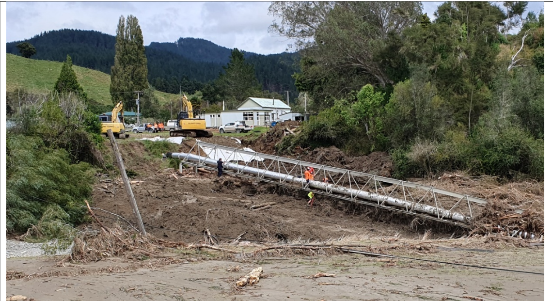
TW Pipe Bridge 4 – Waingake School
