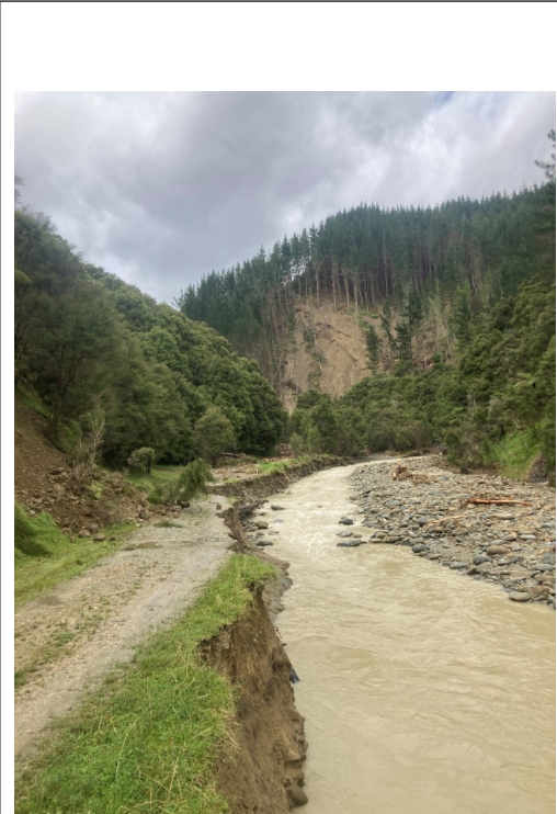
RW Pipe Reinstatement
