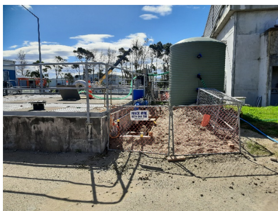
Pump in outfall pump station and feed tank 1
