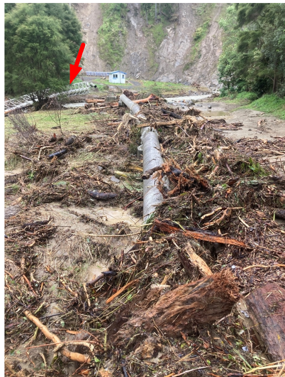
After RW Pipe Bridge 1
