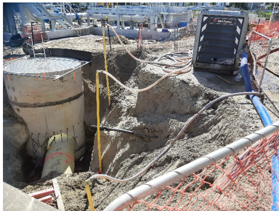
Dewatering spears and pump spears
