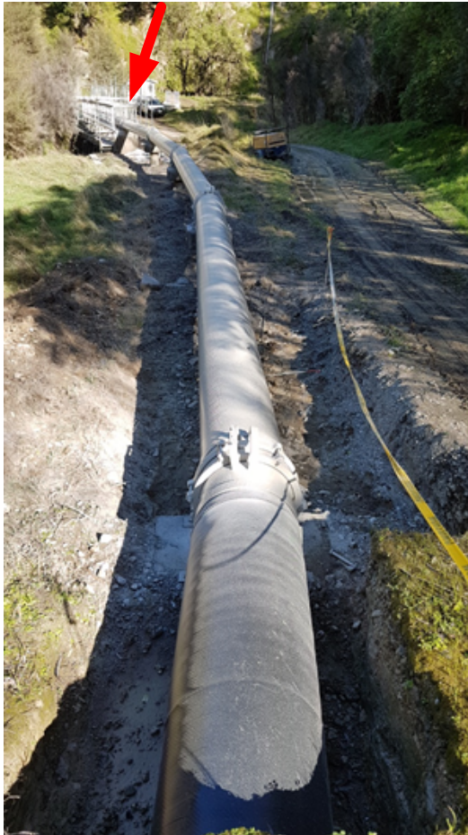
Before RW Pipe Bridge 1
