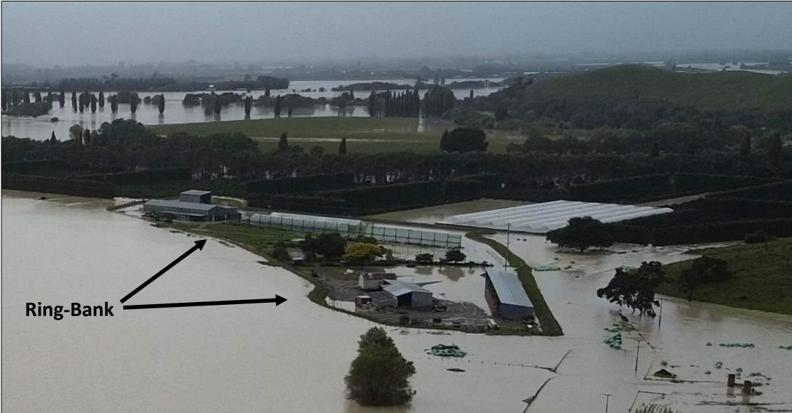
Photo 5 - Wi Pere Trust Ring-bank in operation during Gabrielle.
