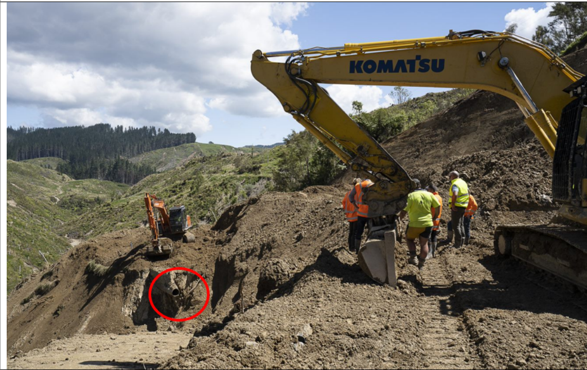
Pipe Reinstatement Rabbit Road
