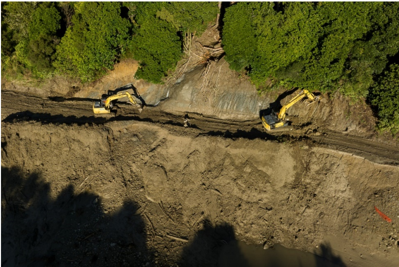
Reinstating road access
