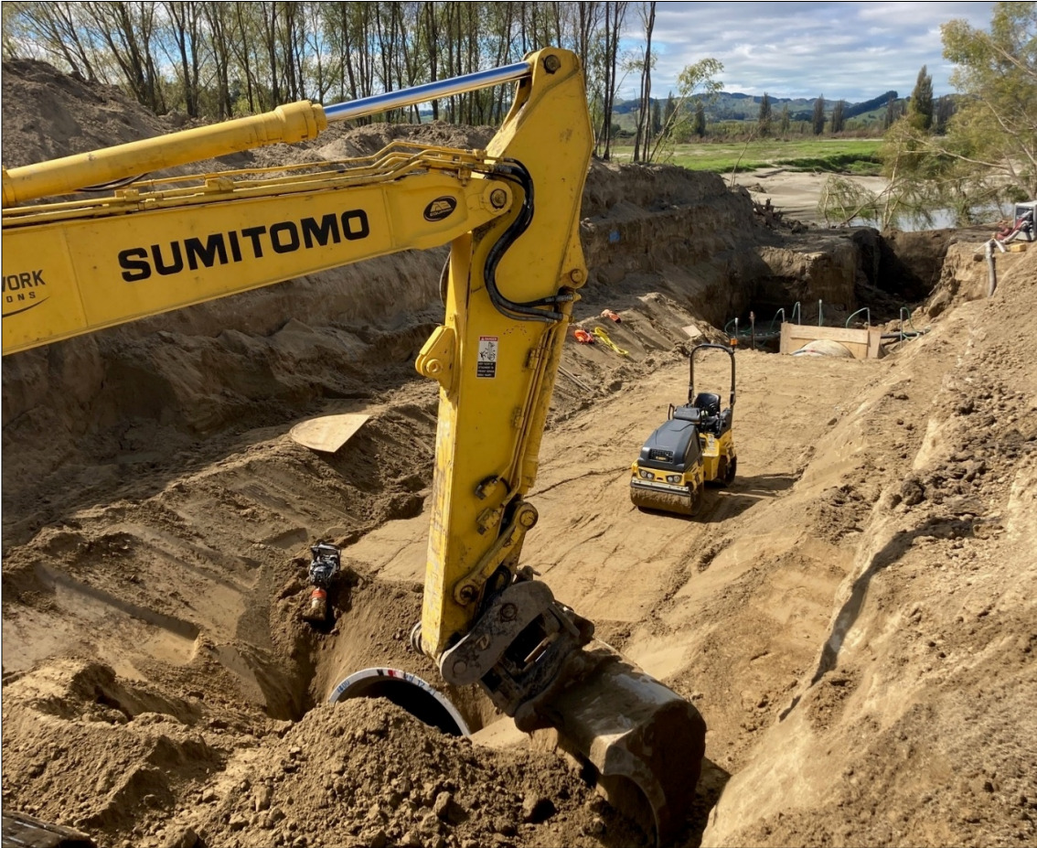
Photo 3 - Lavenham Road – 1800mm dia pipe install works underway, 30 March 2023.
