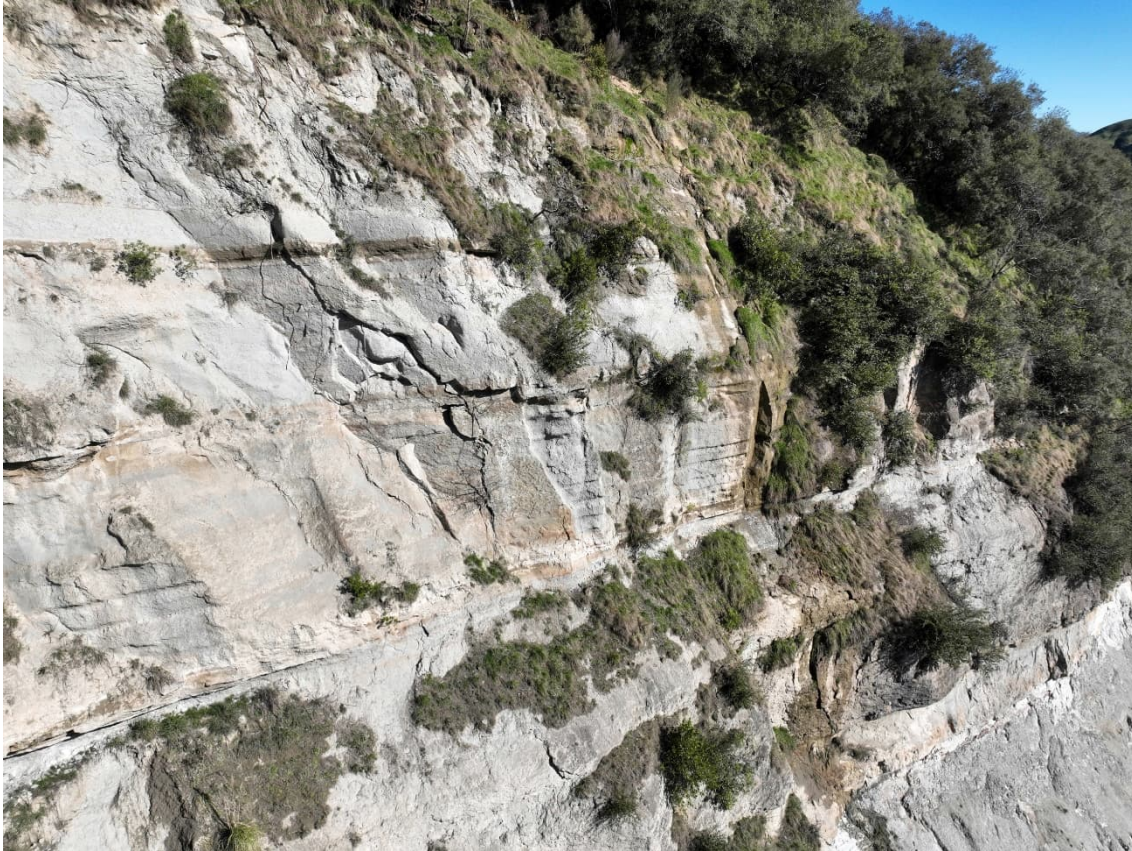
Figure 6: Dilated cracks and defects through and surrounding an unstable block.
