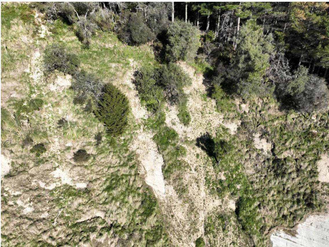
Figure 3: Soil overburden in the upper slopes.
