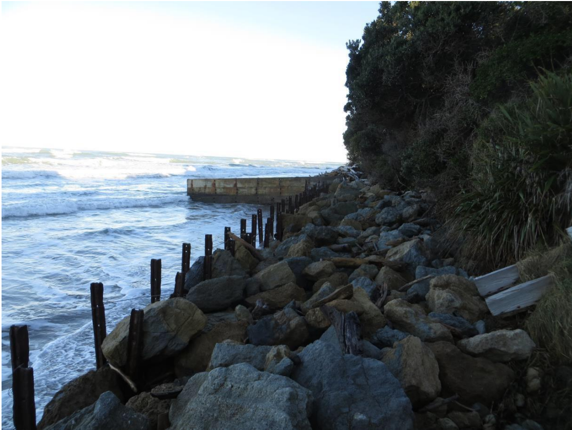
Figure 5 Tuahine Crescent 26 June 201
