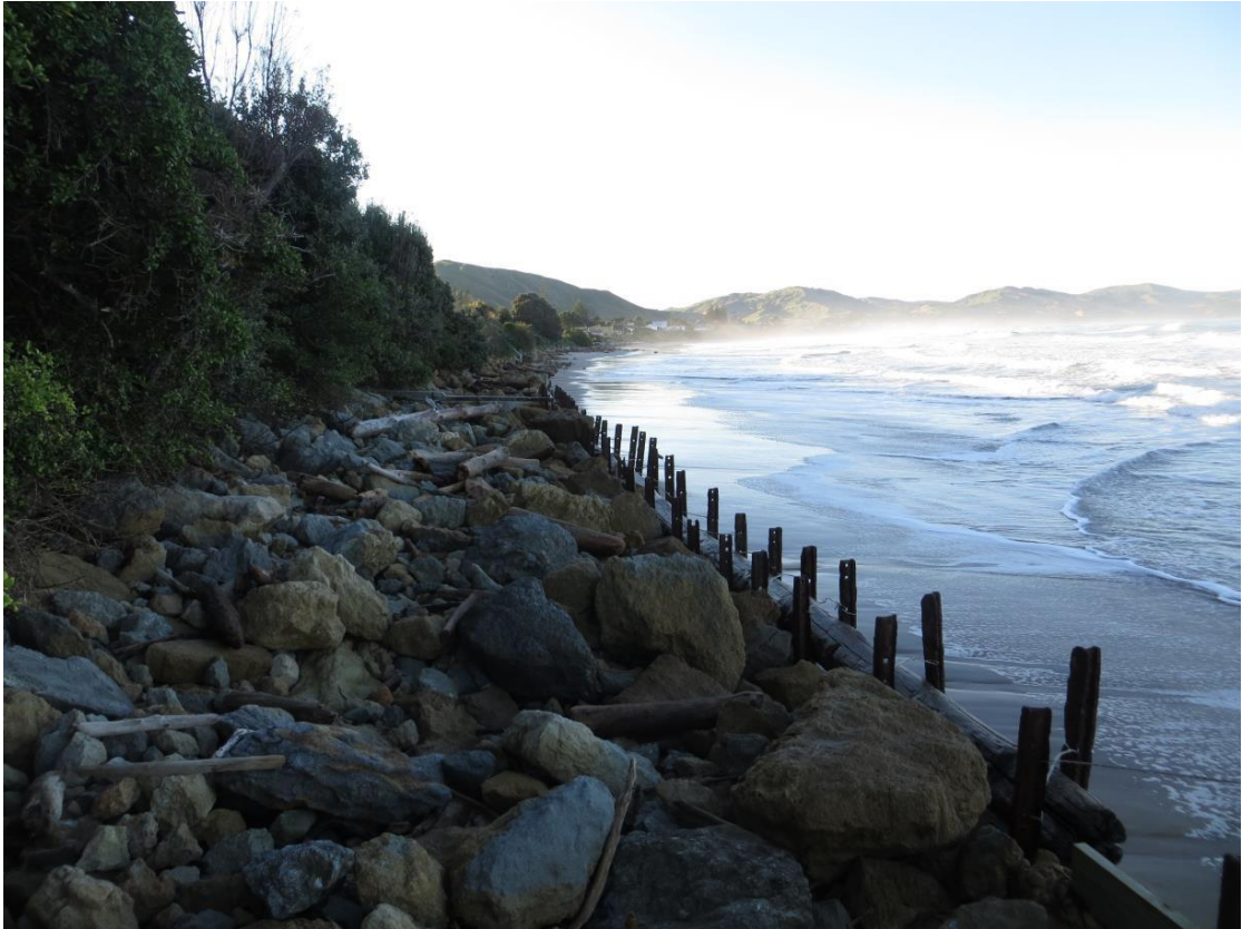
Figure 4 Tuahine Crescent 26 June 2015
