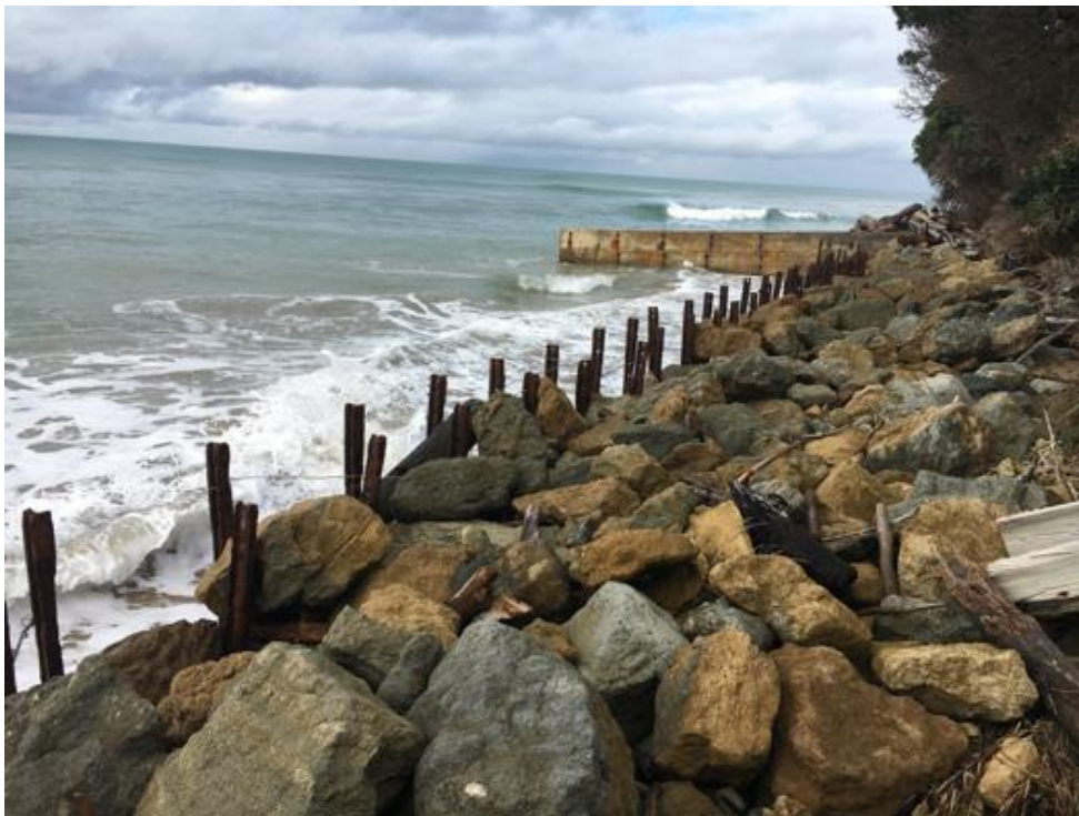
Figure 2: Existing sea wall from public access steps
