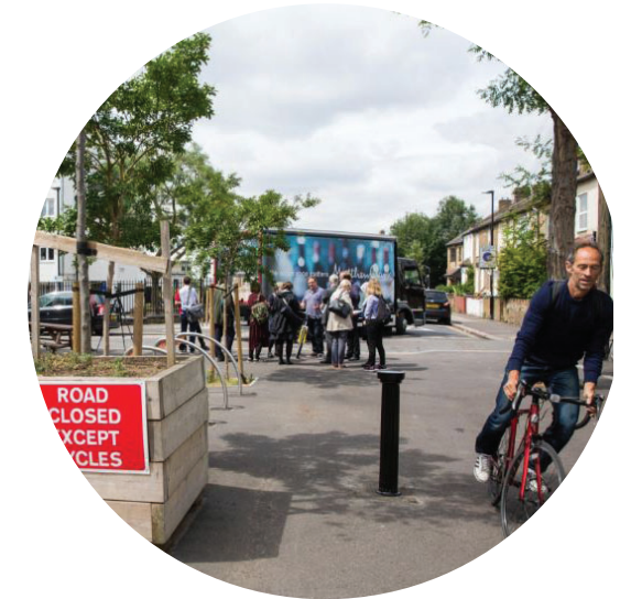
LOW-COST MODAL FILTER (PLANTER & BOLLARD), WALTHAMSTOW, ENG.
