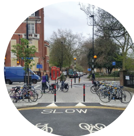
MODAL FILTER COMBINED WITH A RAISED CROSSING AND STREETScape UPGRADE, HACKNEY, ENG.
