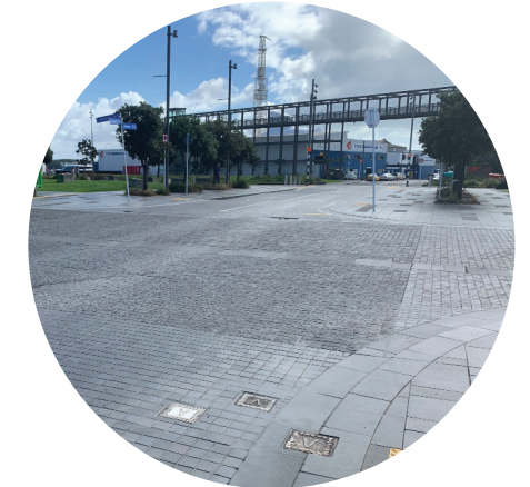
2. RAISED CARRIAGEWAY BETWEEN PARK SPACES
