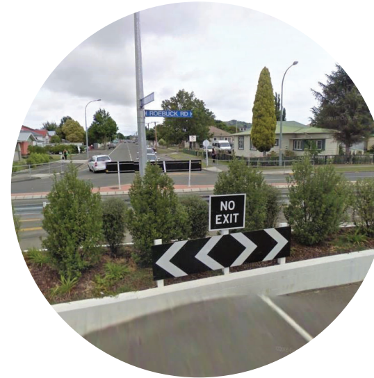
EXISTING MODAL FILTER, PALMERSTON ROAD, GISBORNE.
