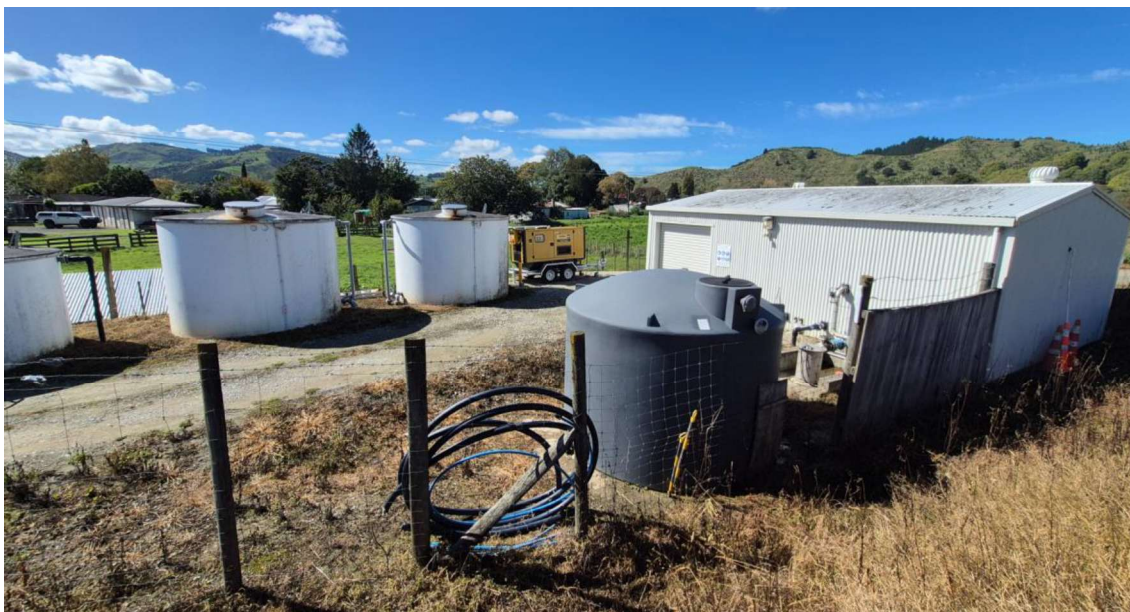
Figure 20 - Existing potable water treatment facility.
