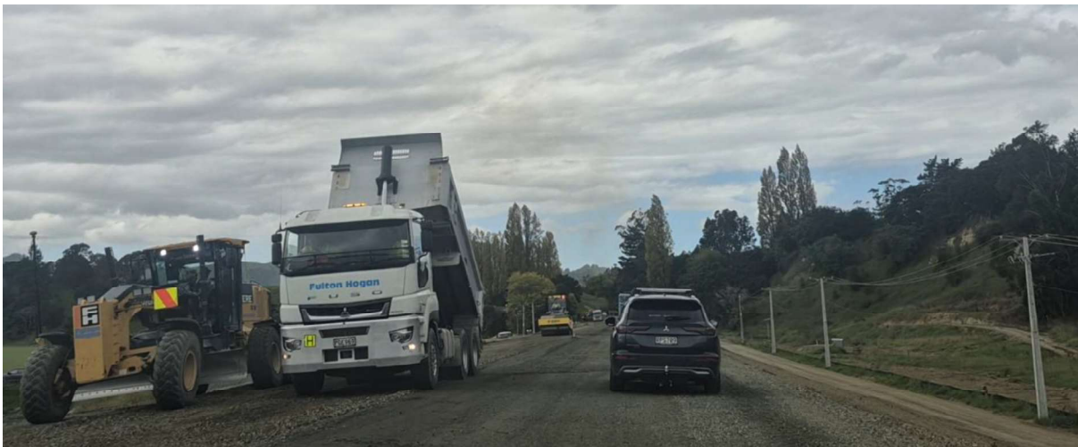
Figure 33 – Further example of temporary single lane road diversion along the Hakanui Straight road raising project.
