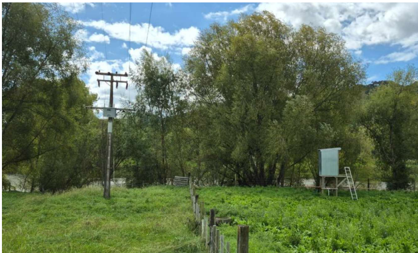
Figure 14 - Photo showing the existing terminal pole for the powerlines running adjacent to the oxidation pond.
