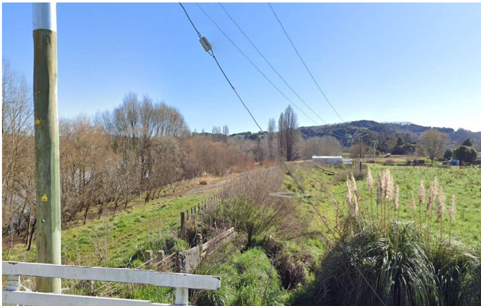
Figure 10 - Photo of existing overhead power lines between Rangatira Road and the potable water treatment facility.
