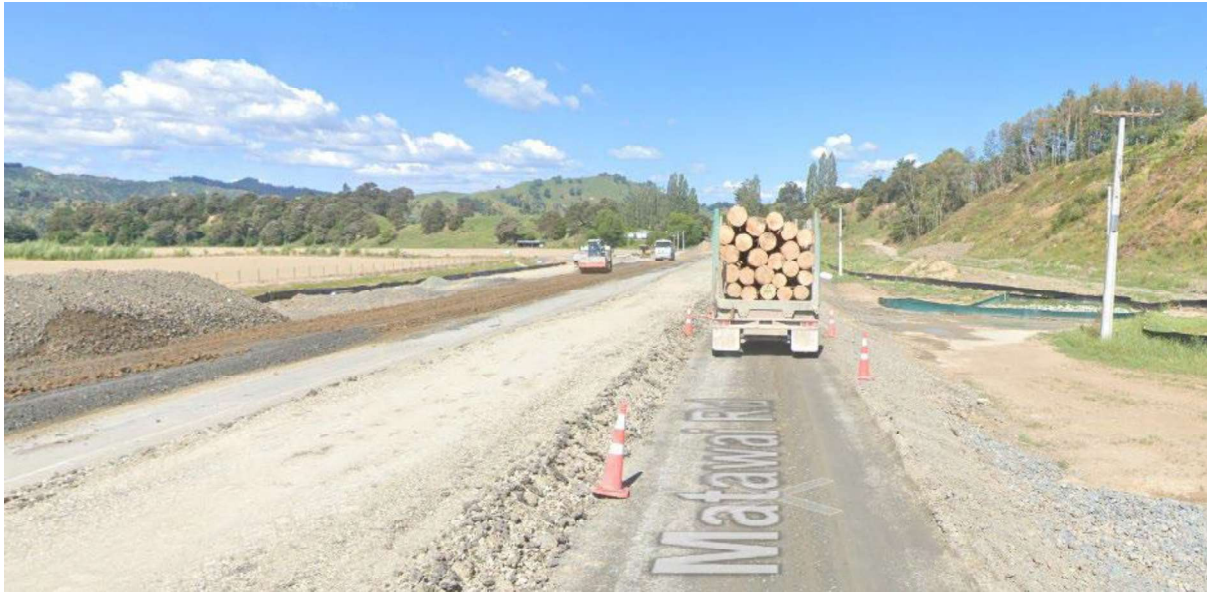
Figure 32 - Example temporary single lane road diversion along the Hakanui Straight road raising project.
