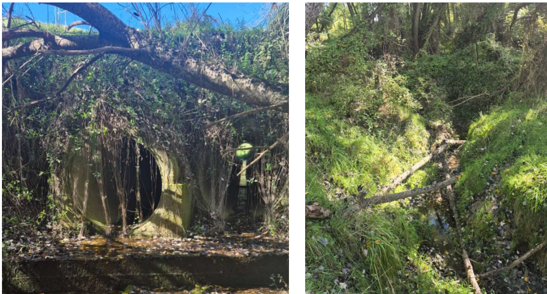
Figure 25 - Photo showing the outlet of the existing culvert and the downstream creek
