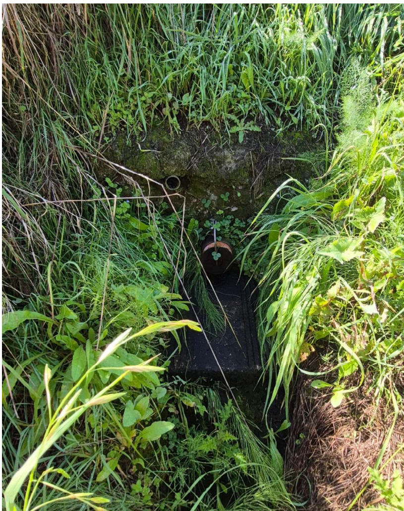
Figure 21 - Existing Water Treatment Plant outlet / scour pipe.
