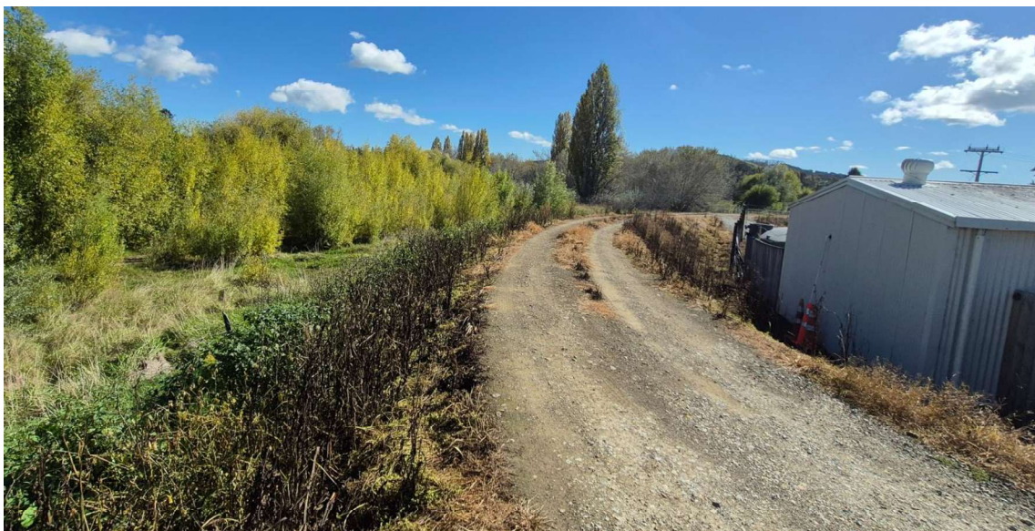
Figure 19 – Photo showing the existing stopbank and the potable water treatment facility.
