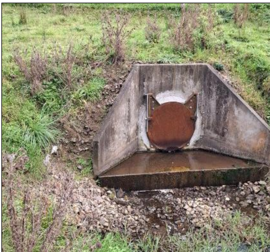
Figure 1: Existing culvert with floodgate at eastern stopbank
