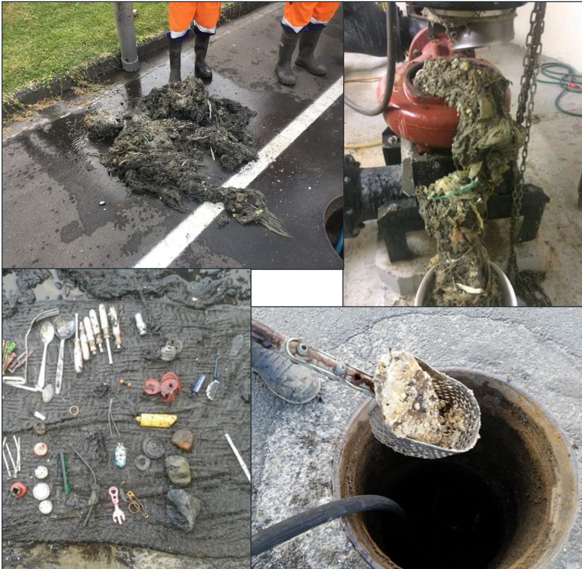
Figure 10: Objects and Material Removed from the Wastewater Network
