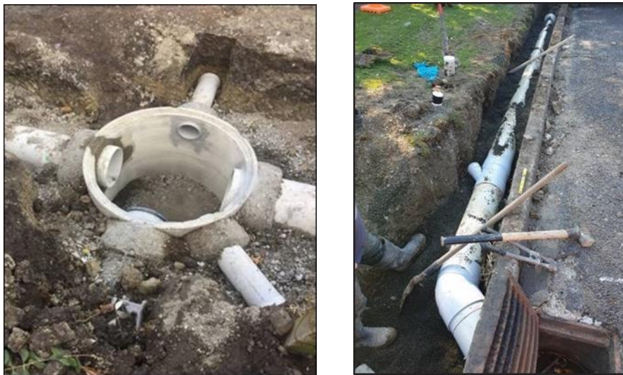
Figure 15: Examples of Drainage Sumps
