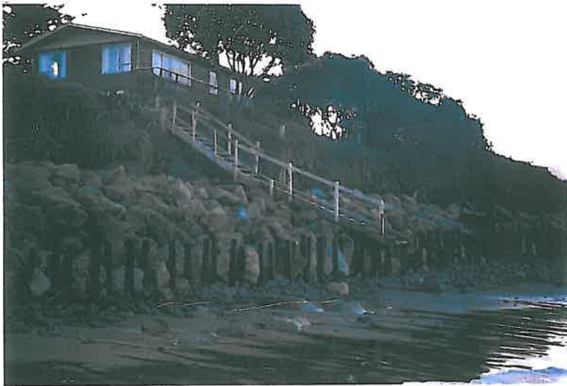
Photo 2: Rock revetment with rail on top, with beach levels low
