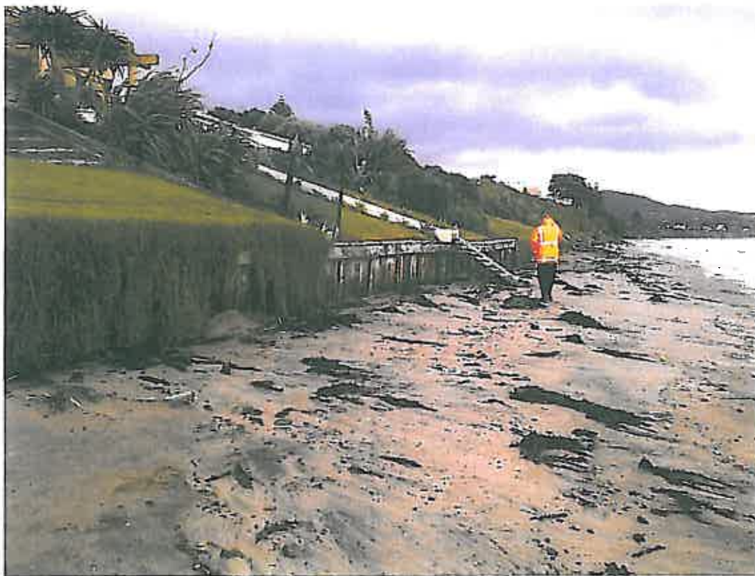
Photo 4: Timber wall with buried gabions toe, with beach levels high
