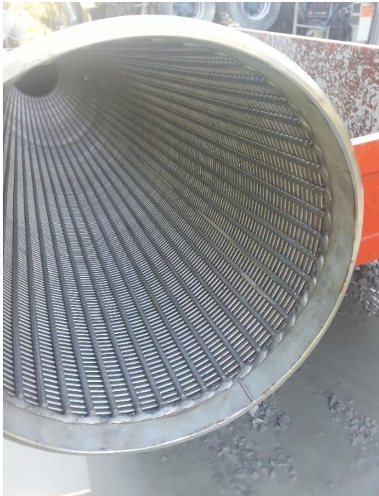
Figure 17: MAR injection well (GPE066) screen shown in left photo; sump and screen leader shown in right photo.
