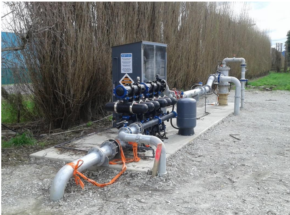
Figure 18: Completed MAR injection well (GPE066), headworks, filter bank and control systems shown in left photo; MAR monitoring well (GPE065) shown in right photo.
