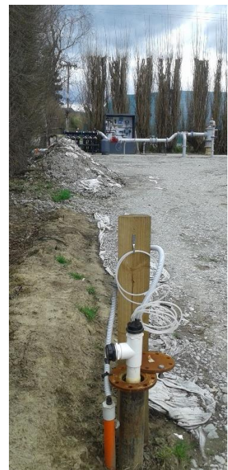
Figure 18: Completed MAR injection well (GPE066), headworks, filter bank and control systems shown in left photo; MAR monitoring well (GPE065) shown in right photo.
