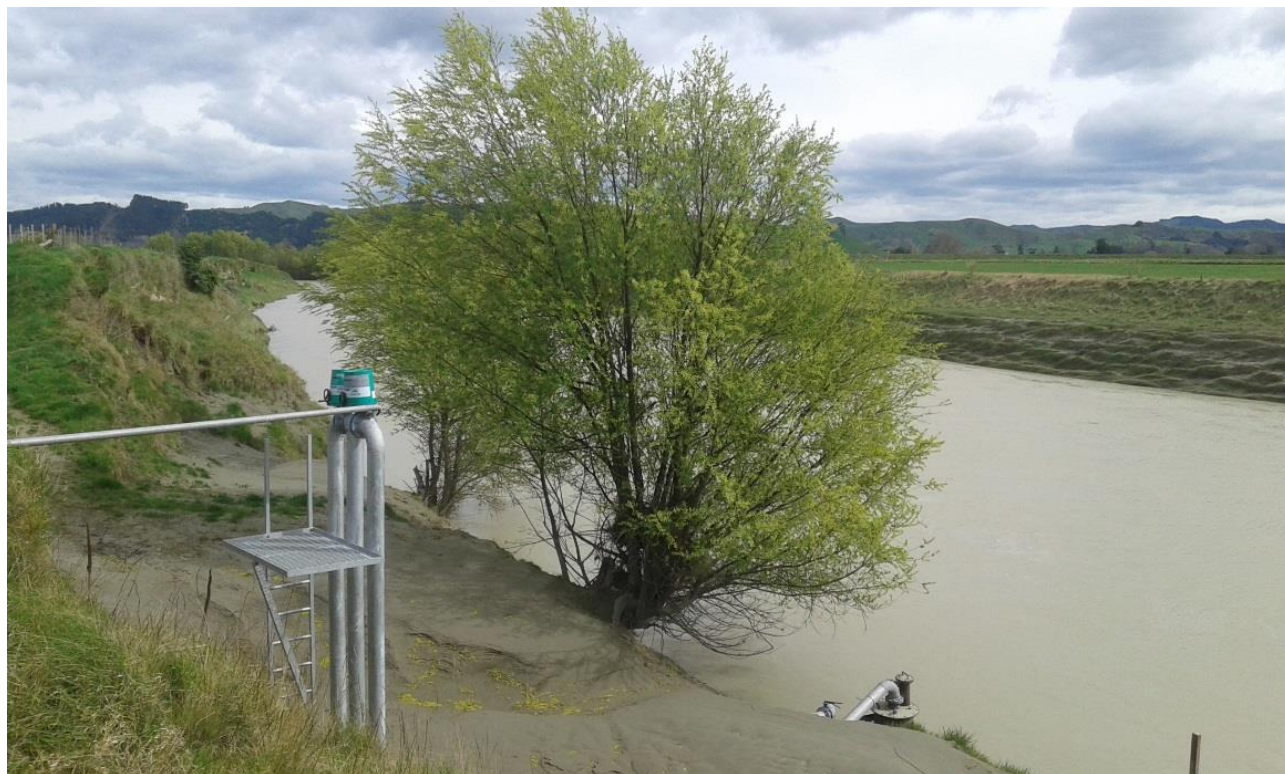
Figure 14: Kaiaponi infiltration gallery for Waipaoa River water abstraction (looking eastwards).
