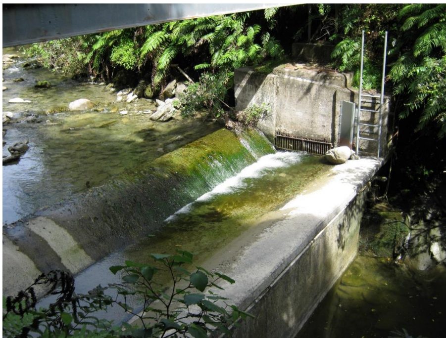
Figure 2-7: Te Arai at Bush Creek intake in April 2010. Source: Doug Booker, NIWA.
