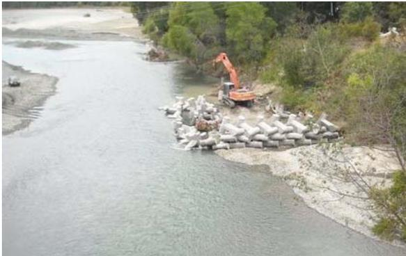
Stage One of the Waiapu River flood control project involves building groynes made of dollasses in the Waiapu River north of the Rotokautuku Bridge to divert fast water back towards the main river channel. The dollasses are doing their job by trapping sediment and creating beaches that can be planted. Stage two of the work to raise the height of the dollasses has funding and is due to start in 2012. Local contractors were used for stage 1 works and this will continue for stage 2.
