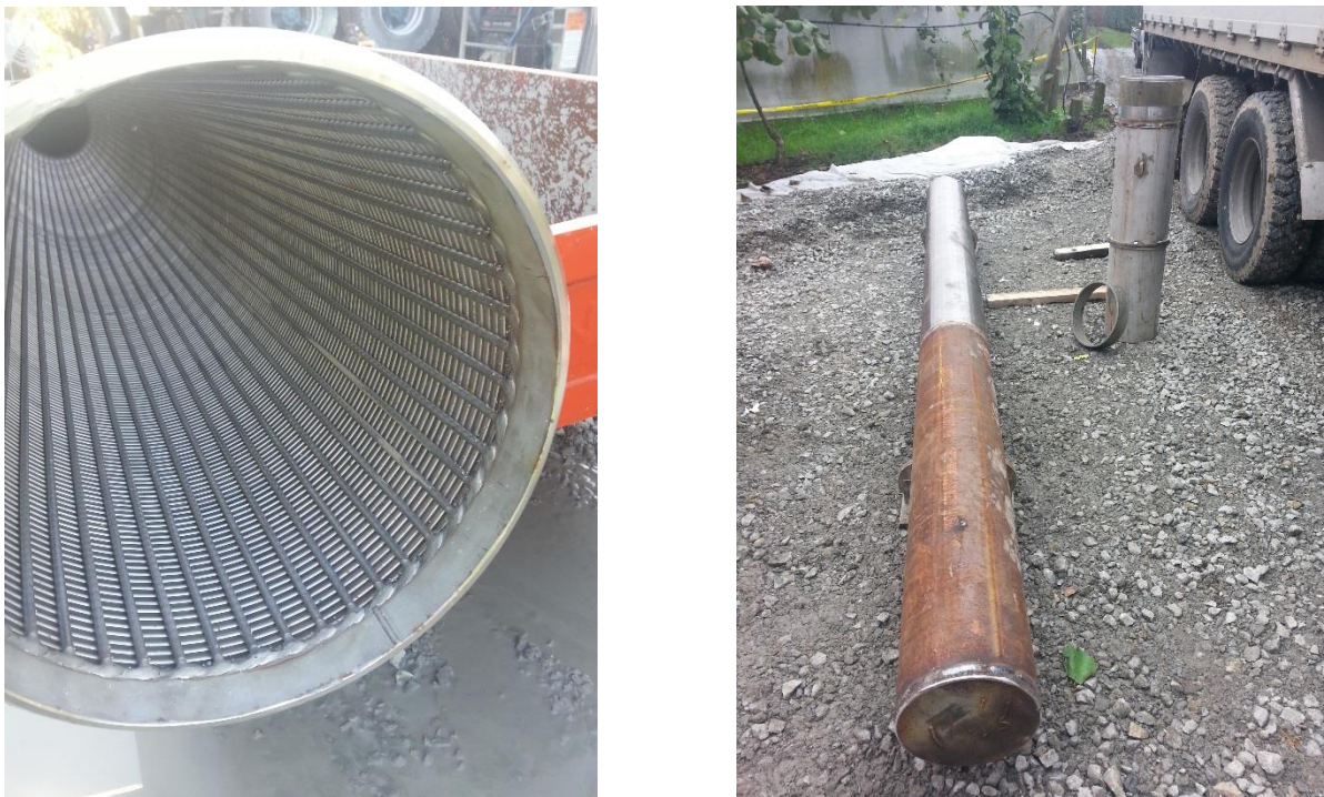
Figure 8: MAR injection well (GPE066) screen shown in left photo; sump and screen leader shown in right photo.
