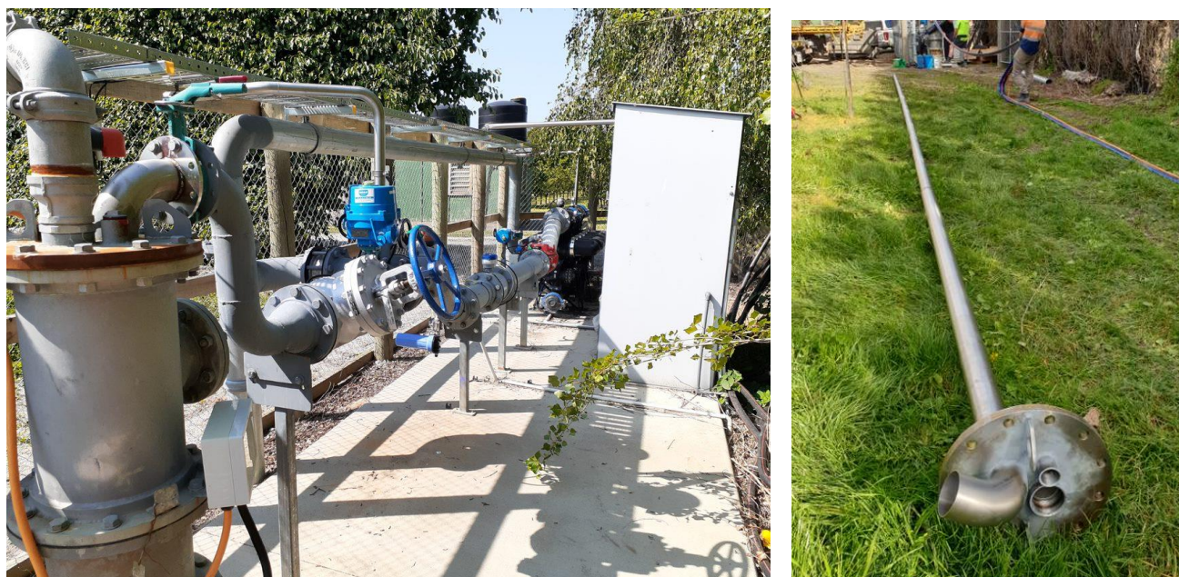
Figure 10: Photo of the Gisborne MAR injection well GPE066 and headworks post-upgrading in 2019 (left photo) and downhole injection pipe (right photo).
