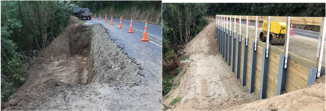
July 2020 -$17.6m - retaining wall structure on Mata Road in progress.
