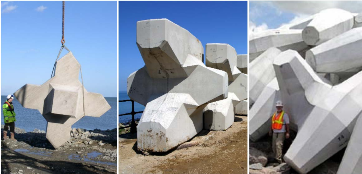
Figure 3-5 – Left – X-bloc® (4 m 3 /9.6 t, Port Oriel, Ireland). Centre – Accropode units (6.2 m 3 /14.9 t, Scarborough UK). Right – Core-loc® (15 m 3 /36 t, Kaunapali Harbor, Hawaii). (Reedjik & Muttray, 2009)
