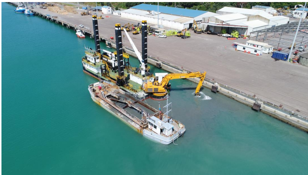
Figure 3-27 Backhoe dredging – the backhoe is placed onto a barge and dispose removed sediment into the Pukunui vessel.
