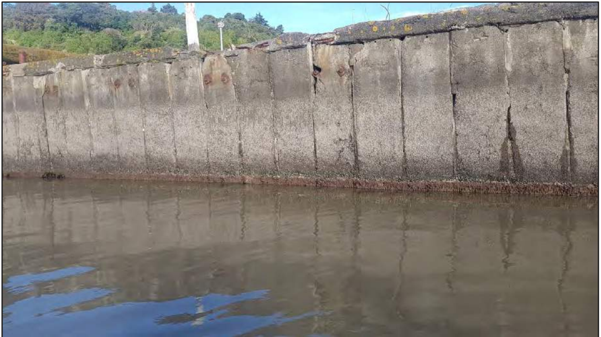
Photo 6: Typical view of the southern concrete sheet pile wall adjacent the marine railway.
