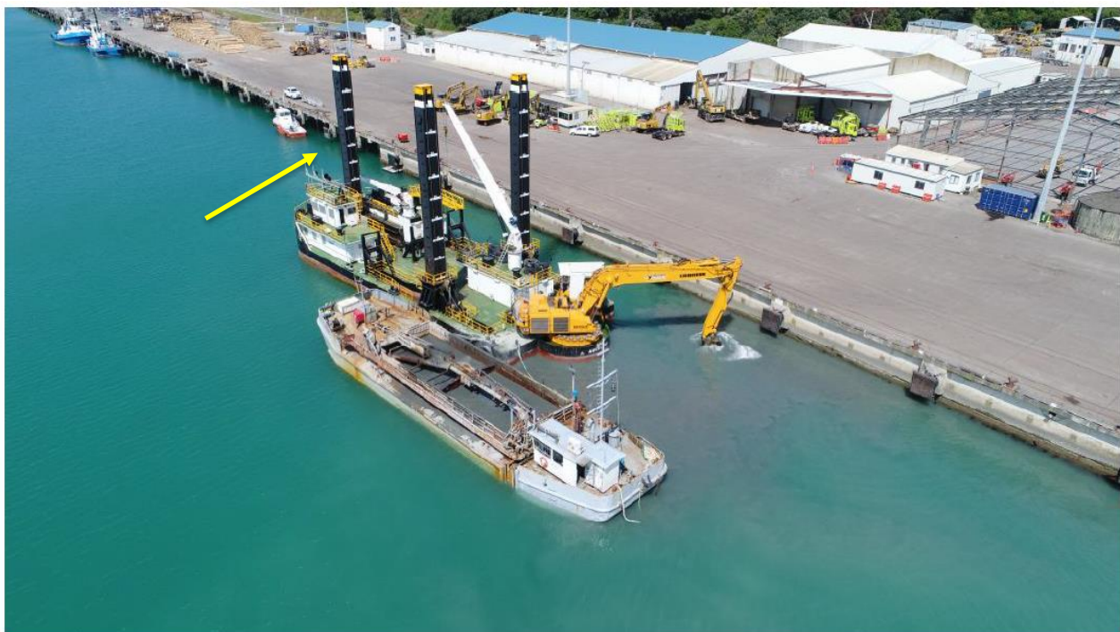
Figure 15: Backhoe loading Pukunui at Port Gisborne (Source MetOcean, April 2018; Figure 3.44).
