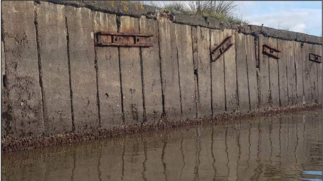
Photo 5: Typical section of northern concrete sheet pile wall adjacent the marine railway.
