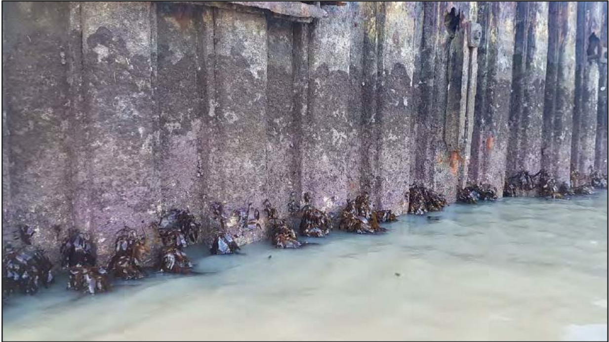
Photo 1: Marine growth on southern steel sheet piles (port side).
