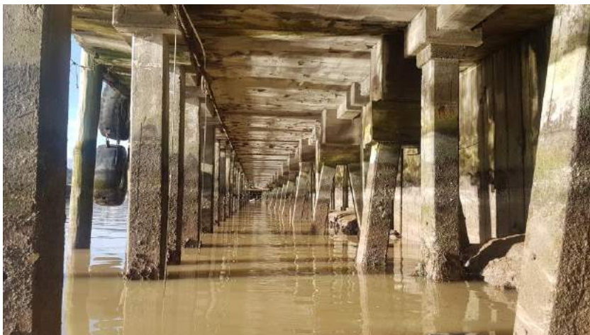
Photo 6: Wharf 6 looking east showing a fender (timber) pile, line of front concrete piles and rear raking piles
