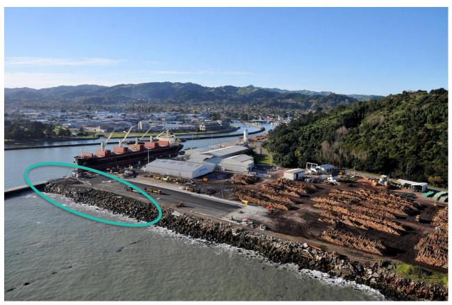
Figure 3: The southern seawall at Eastland Port, looking north towards the Southern Logyard and Gisborne central business district. The area of circled in teal is approximately 130 m of the seawall to be deconstructed as part of the Twin Berths Project (TBP).
