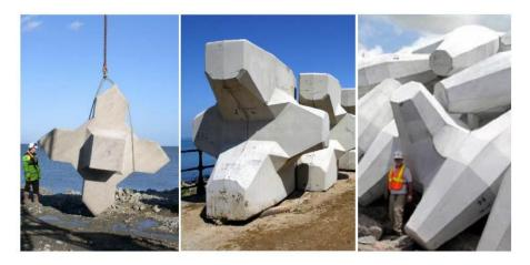
Figure 3-5 – Left – X-bloc<sup>®</sup> (4 m³/9.6 t, Port Oriel, Ireland). Centre – Accropode units (6.2 m³/14.9 t, Scarborough UK). Right – Core-loc<sup>®</sup> (15 m³/36 t, Kaumalapau Harbor, Hawaii). (Reedjik & Muttray, 2009)
