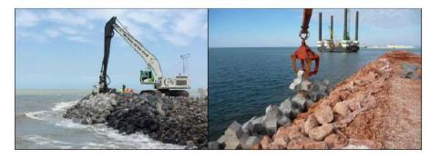
Figure 3-6 – Examples of typical random placement of X-bloc<sup>®</sup> units
