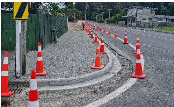
Channel, curbing and new footpath installation along SH 35
