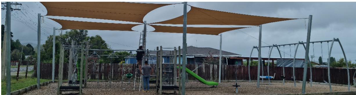
Installation of the Tikitiki Playground shade sails – Sunday 30th October 2022.
