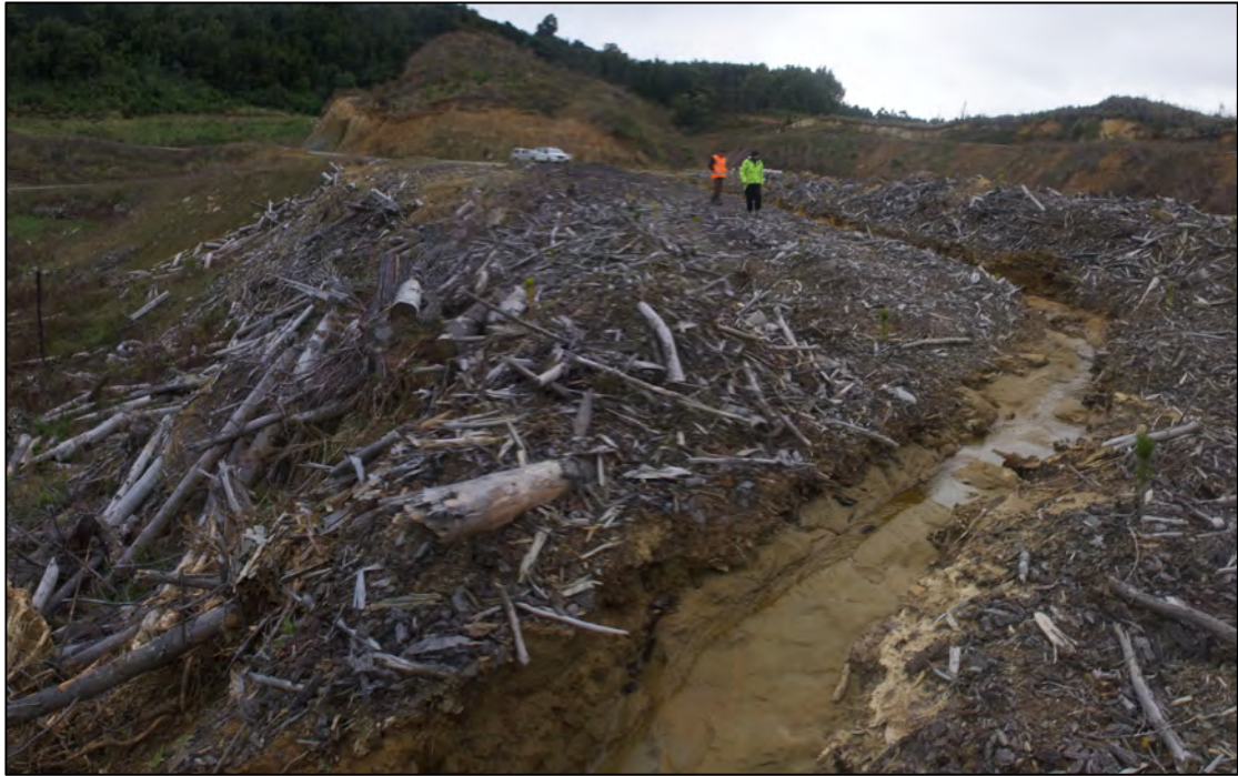
Figure Forty Two. View of the longitudinal drain cut through the middle of Site Eleven showing the deep incising through logging waste material.
