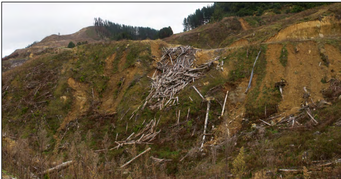
Figure Forty One. Composite Image (1D1A7958-1D1A7959) looking north west from Site Eleven showing a culvert with a sock directing stormwater onto slope materials which have washed away leaving bare rock. Further slope failures in side cast material is evident to the right of the culvert.
