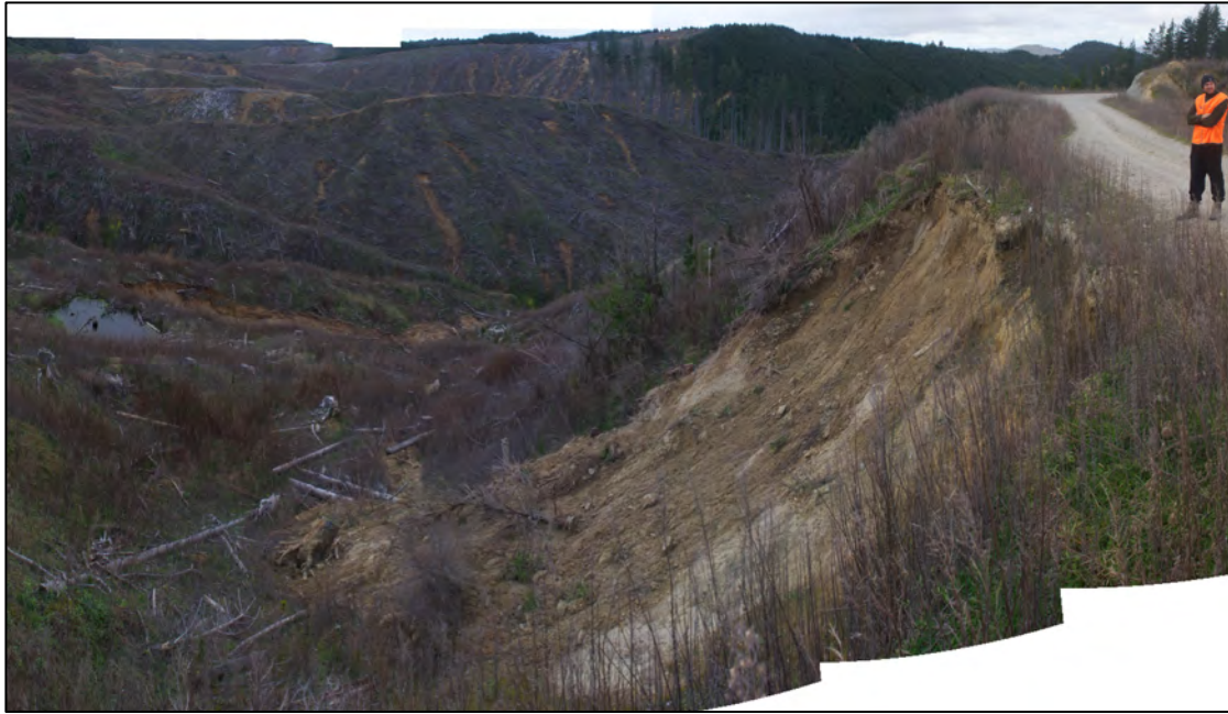
Figure Sixteen. Significant slope failure south east of Site One that has occurred where a cut out has directed water onto side cast material [Image is a stitched together composite of images 1D1A7818 to 1D1A7822].
