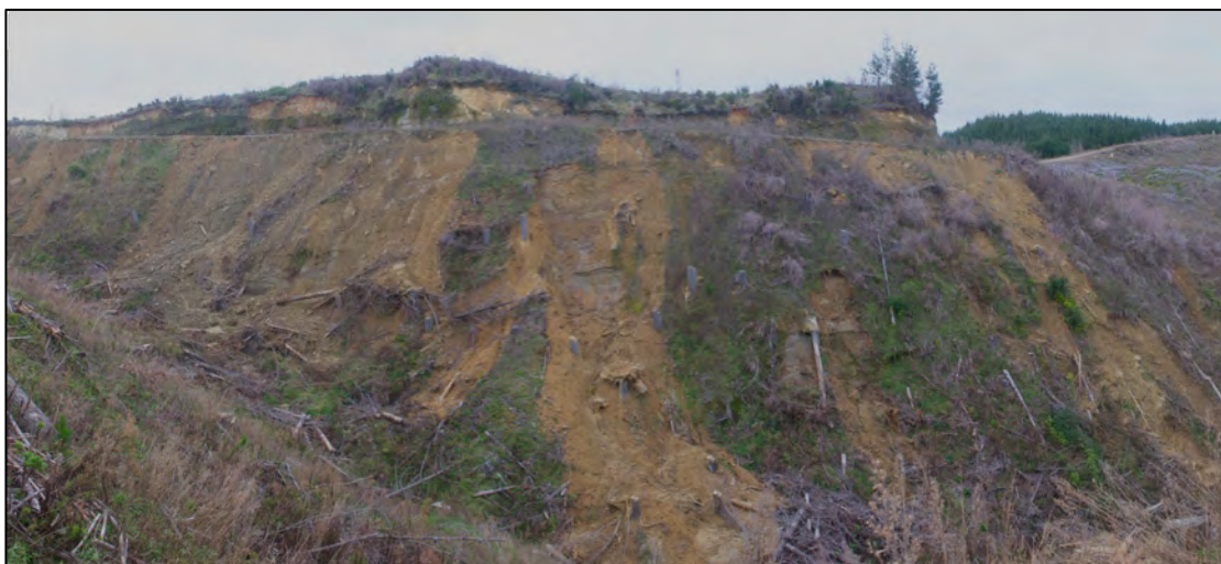
Figure Forty Five. Composite image (1D1A7925 to 1D1A7930) showing the extent of slope failures in side cast material from Bush Road.
