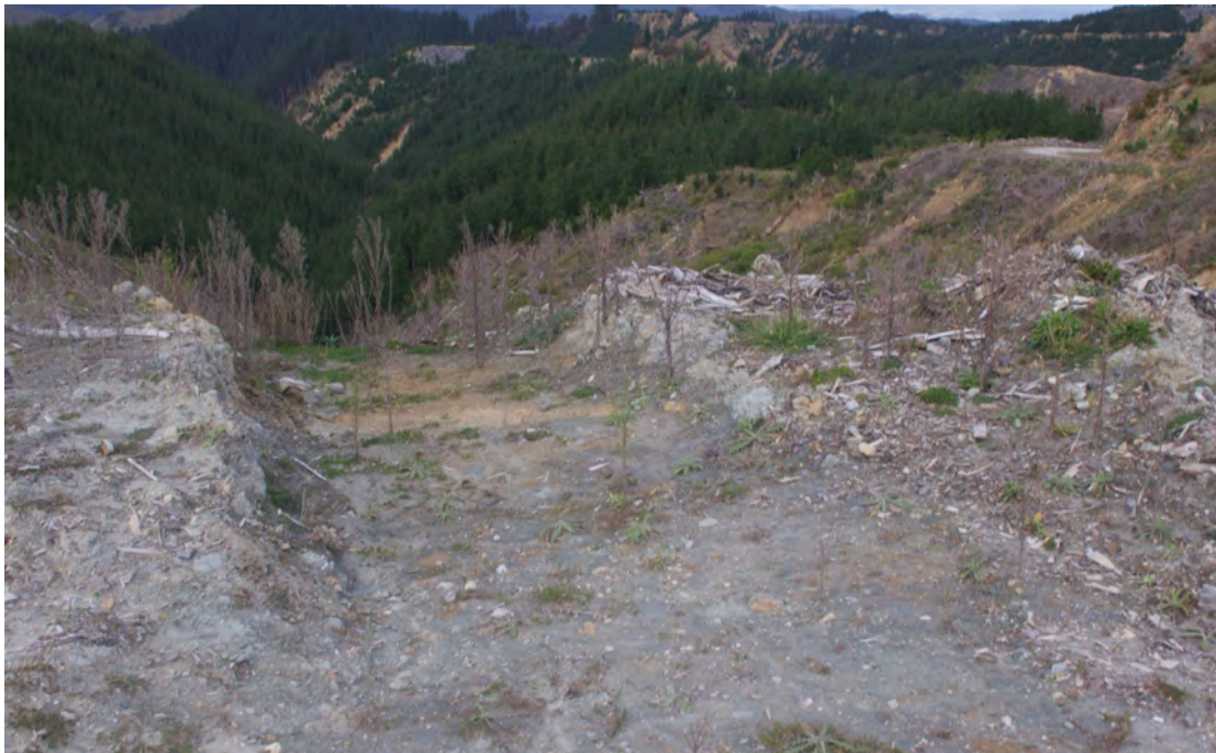
Figure Fourteen. Image 1D1A7816. View of cut out on western side of site one showing cut out directed onto side cast material. In the background (right) several slips originating from Woolshed Road are evident.
