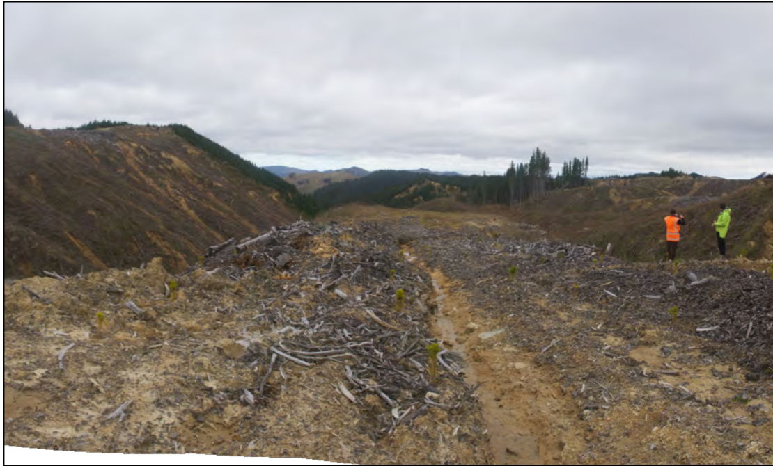
Figure Forty Four. Composite image (1D1A7947 to 1D1A7950) showing the longitudinal drain and the slumped material immediately to the east. Not the indications of standing water in the drain. During storm events this drain would carry significant volumes of water some of which would have been redirected across the skid site saturating the logging waste forming the base of the perched log pile that has slumped on the eastern side.
