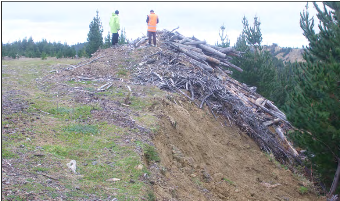
Figure Thirty One. Logging debris stowed on the western edge of Site Three with an obvious drain directing water over the edge of the skid onto side cast material in the foreground.
