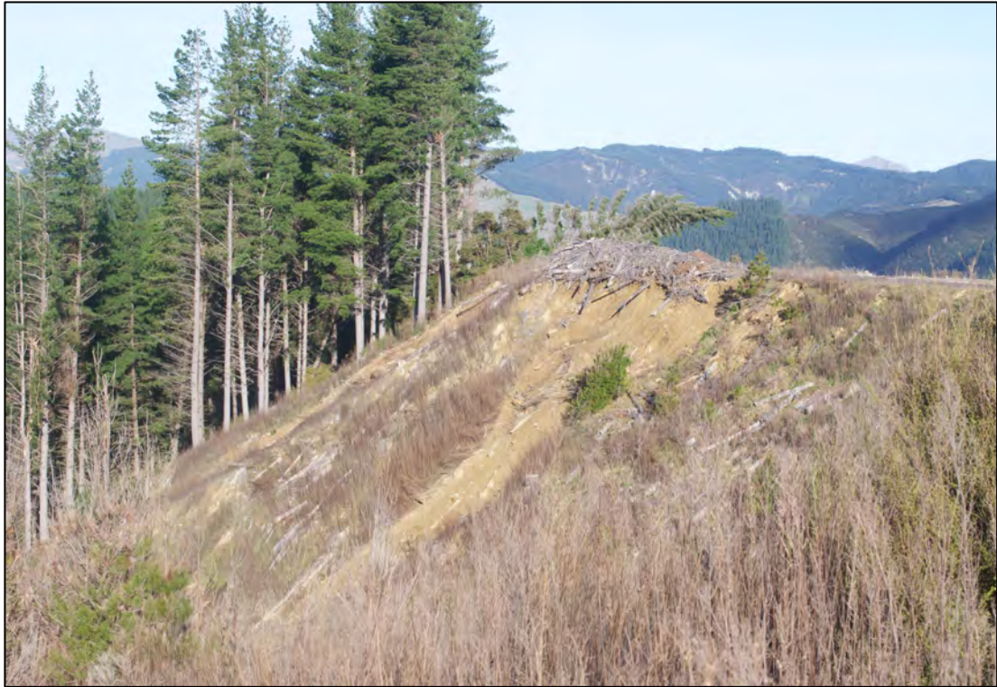
Figure Twenty. Image 1D1A1019 showing skid Site Two from Woolshed Road showing the failure on the eastern side of the skid and the logging debris perched on the edge.
