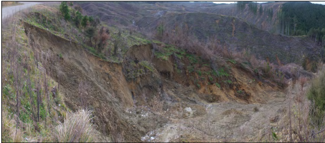
Figure Eighteen. Large slope failure around 200m south east of Site One resulting from water directed over the eastern side of the road. The image is a stitched composite of photographs 1D1A7834 to 1D1A7840.
