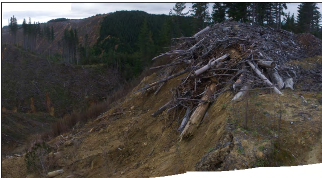
Figure Twenty One. Composite image (Images 1D1A7844 to 1D1A7847) showing the log pile overhanging the edge of the skid. A tension crack and part of the drainage channel is evident in the foreground.
