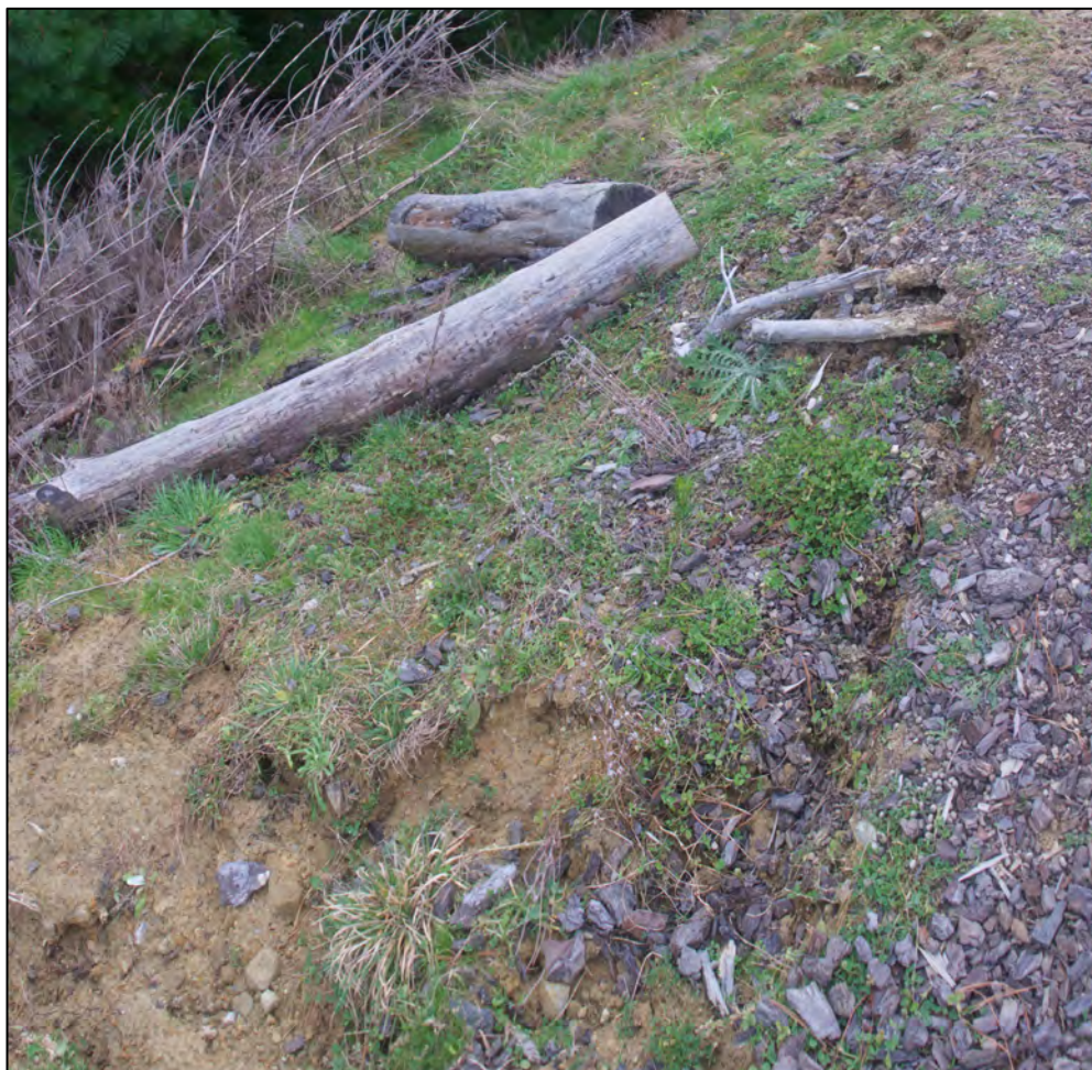
Figure Twenty Nine. Composite of Images 1D1A7880 and 1D1A7881 view showing a tension crack at the edge of the gravel pad on the eastern side of Site three. Note the presence of woody material caught up in the gravel pad and the tension crack leading to a slope failure. Such cracks act like a channel directing water onto the side cast.
