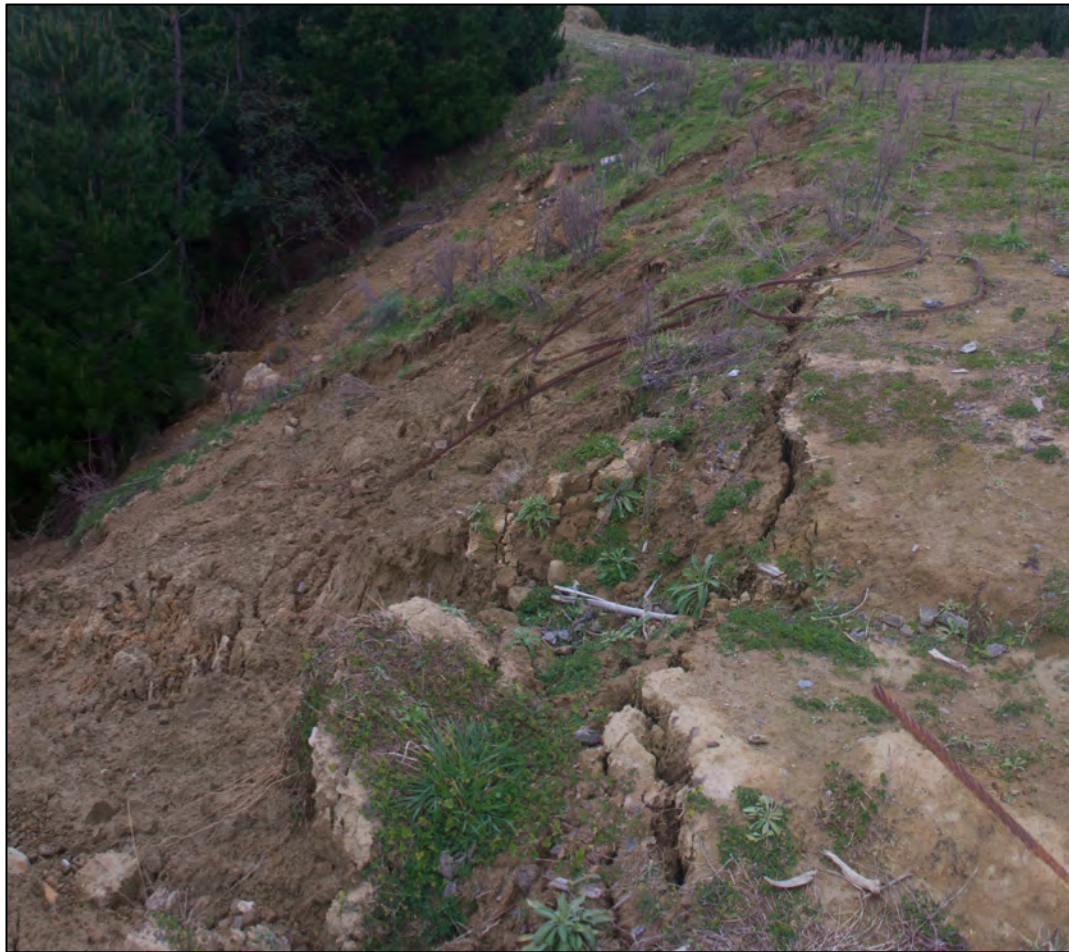
Figure Thirty One. View of the same area as in Figure Thirty showing the drain cut through to side cast material on the south side of the skid. Note the large tension crack cutting through the slope edge.
