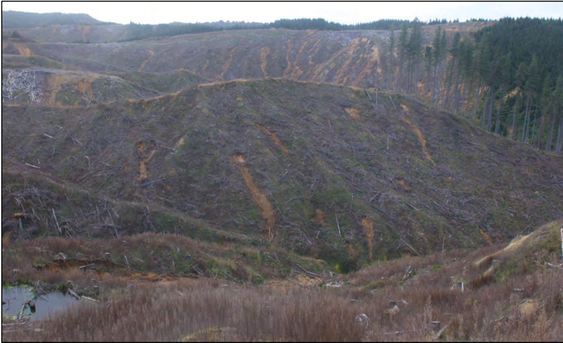
Figure Nine Image 1D1A7810 View looking east from eastern side of Site One showing a headscarp for a significant debris flow immediately below the water storage dam (bottom left), relatively small slips originating on the middle part of the slope (middle ground), significant failure of skid site 13 (Top left), and slips from adjacent to roadways (top).
