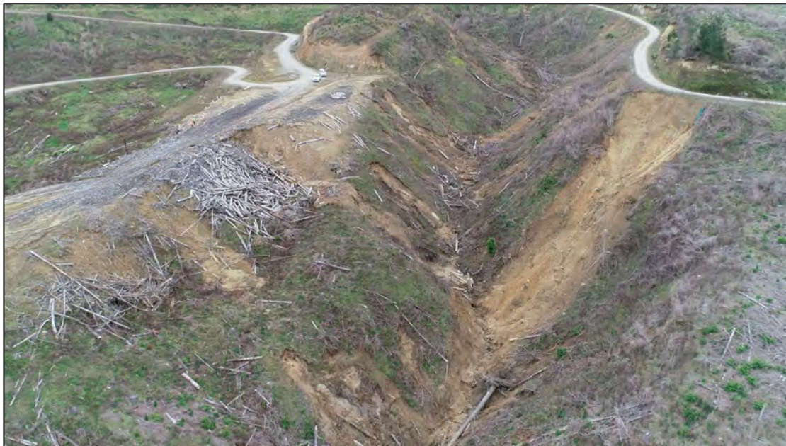
Figure Fifty Eight. A closer view of Site Eleven on the left and Bush Road highlighting the level of failures from Site Eleven and the bench below the perched material. On the far left the bench as caught the logging debris and has acted as an effective berm but in the middle ground the berm has not been an effective barrier and the slope failure has reached the valley floor. The major slope failure from the culvert and sock is on the right.
