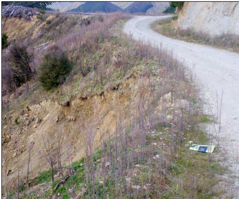
Figure Seventeen. View of headscarp of failure south of Site One on Woolshed Road. In the foreground some material has been placed to form a berm but where this berm is cut out water has been directed onto unstable side cast material leading to failure. On the opposite side of the water course has not been maintained and is full of vegetation and as a consequence water would have flowed across the road contributing to the failure. Site Two is visible in the background.
