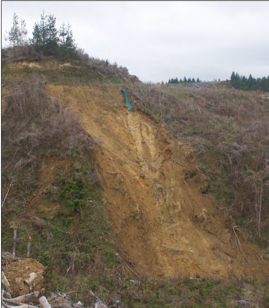
Figure Forty Six. Image 1D1A7965 showing a short section of sock from a culvert on Bush Road discharging water onto the top of side cast material on the slope resulting in the material failing.
