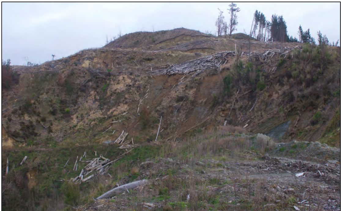
Figure Eight Image 1D1A7809. View looking west towards Duncan Road (top) and Bevan Road showing slope failure from log pile below Duncan Road to Bevan Road with logs blocking the lower Road.
