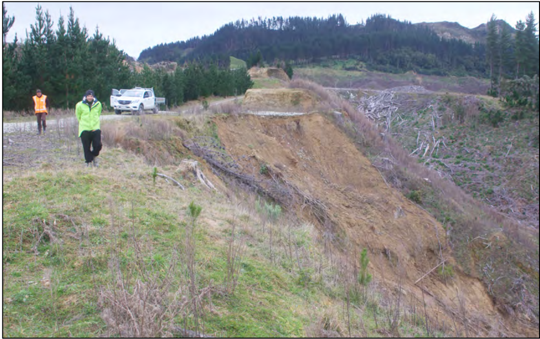
Figure twenty Six. Image 1D1A7858. View of eastern side of Site Three showing failure number 2 (background and failure 1 (obscured middle ground) with person standing at low point where water drains onto side cast material that has failed.
