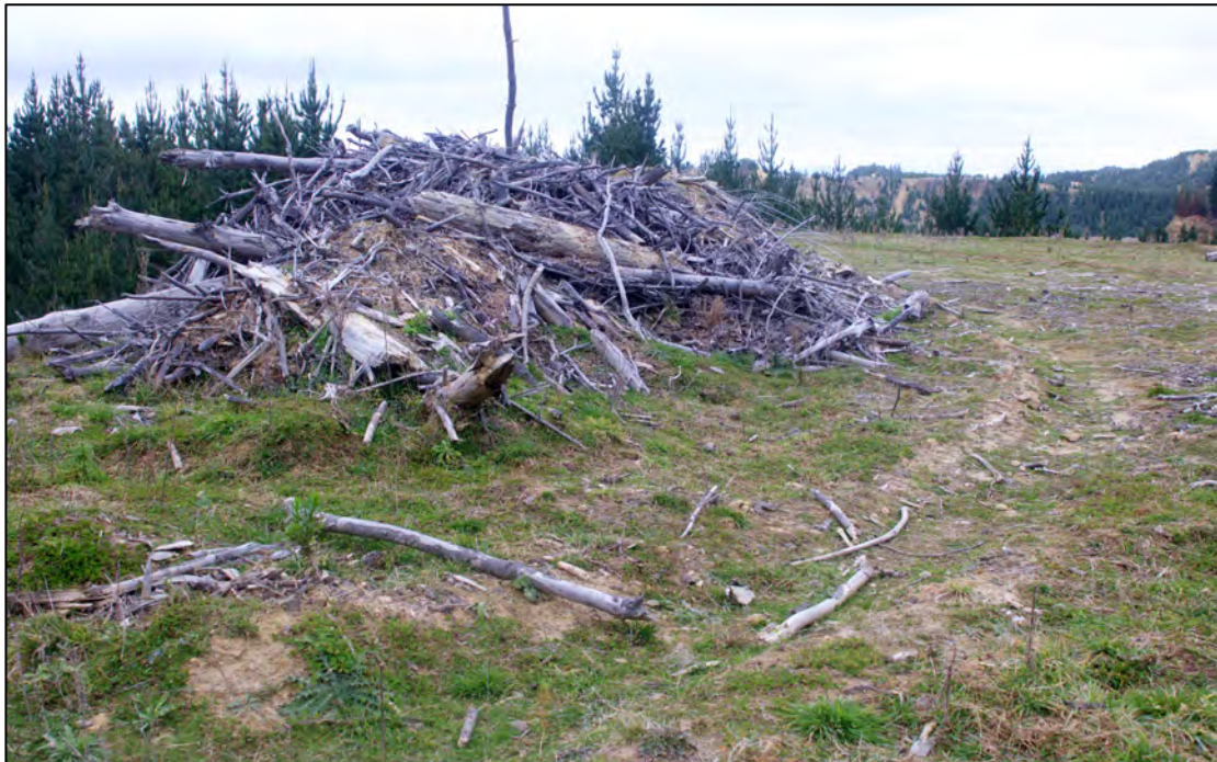
Figure Twenty Five. View of the logging debris pile perched on the eastern side edge of the skid at site 3 with a drain directing water onto side cast material.
