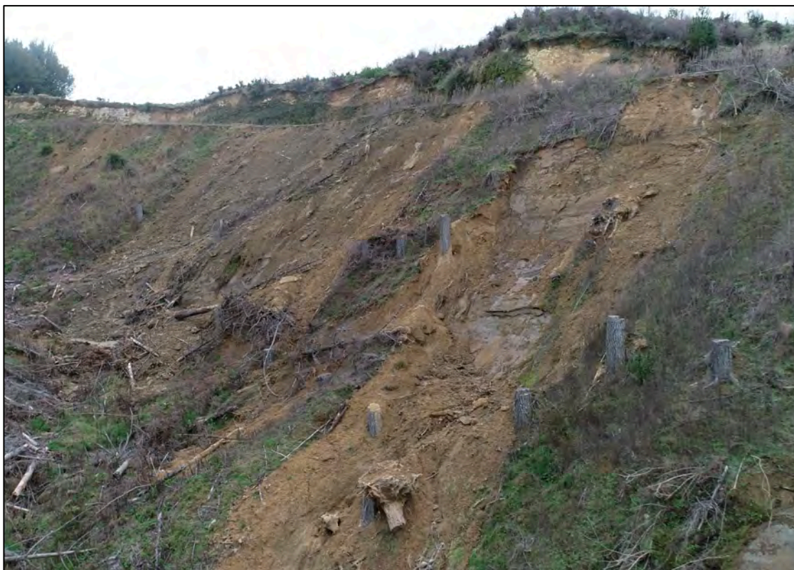
Figure Sixty. Close up view of the slope failure from Bush Road showing that this has occurred in side cast material as indicated by the soil caught up behind the trunks of the stumps at top middle.
