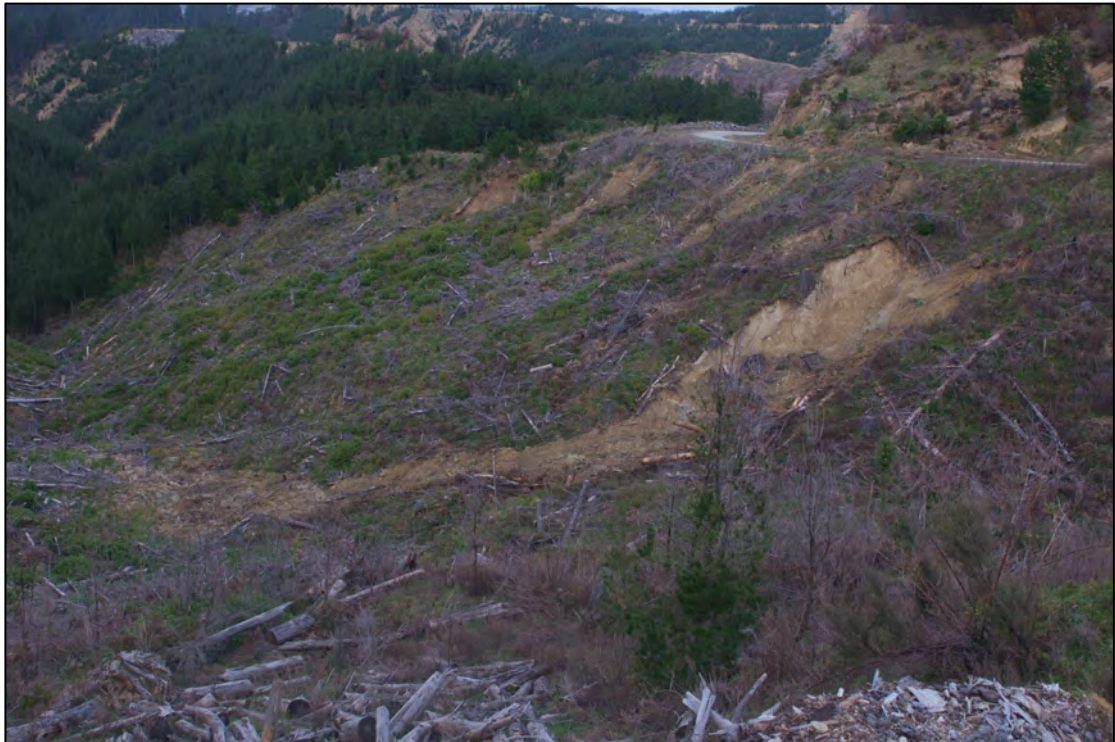
Figure Seven Image 1D1A7808. View looking south east along Woolshed road from the edge of the woody debris pile on the northern side of Site One showing multiple failures originating at road level with one large slip in the foreground.
