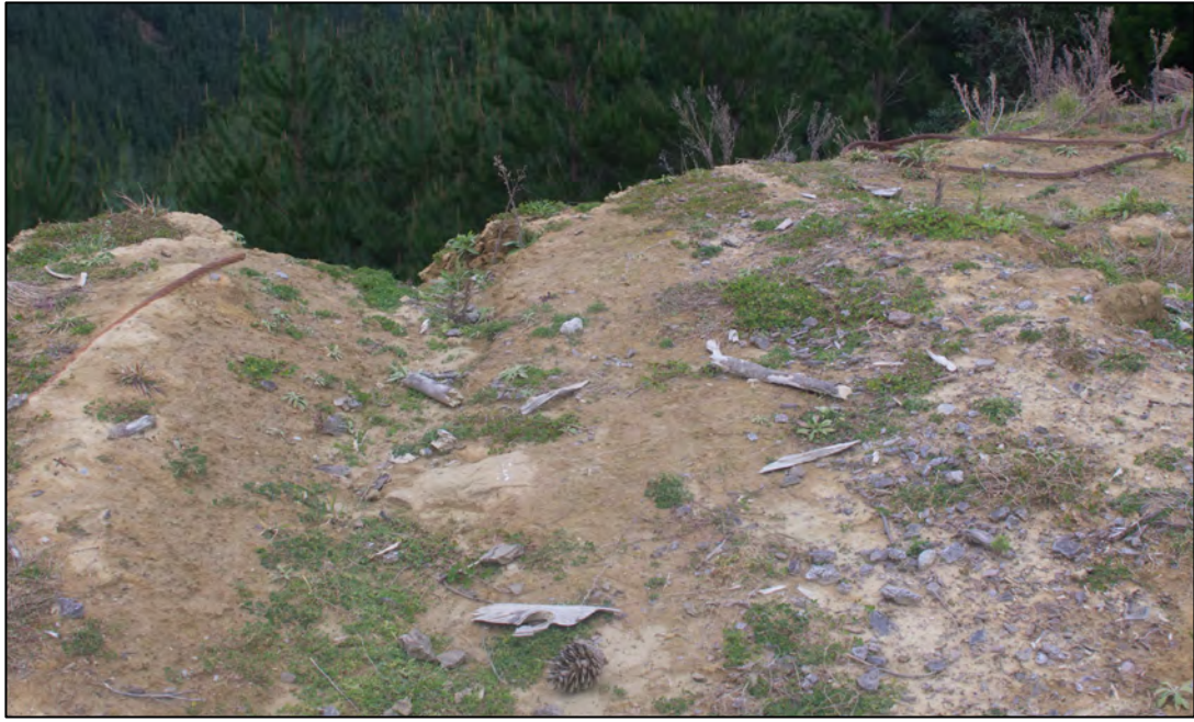
Figure Thirty. View of a drain cut through to side cast material on the south side of the skid. Note the poor house-keeping with wires left lying on the edge.
