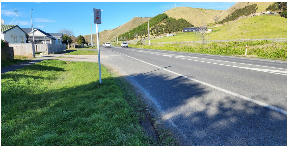
Figure 49 Example of a bus stop with poor facilities and no accessibility for mobility impaired people
