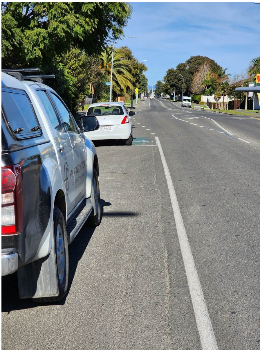
Figure 15 Example of an On-road cycle Lane occupied by a ute and ending in a parked car
