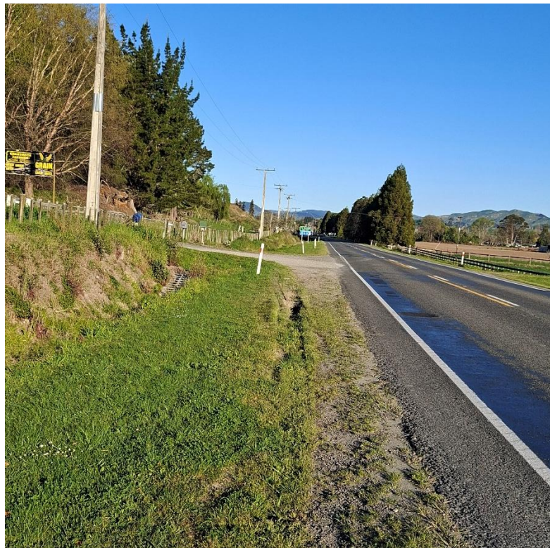
Photo facing east (heading towards Te Karaka). Tyre marks showing where cars and trucks pull left, before turning right into our second driveway / trade entrance. This side is much flatter on the camber. This is what we will lose once the roadworks are done. Note the dashed yellow no overtaking line which starts here and goes to the Te Karaka turn off.
