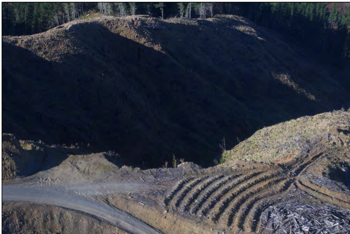
Figure Nineteen. View of stowage of spoil on skid site 47.
