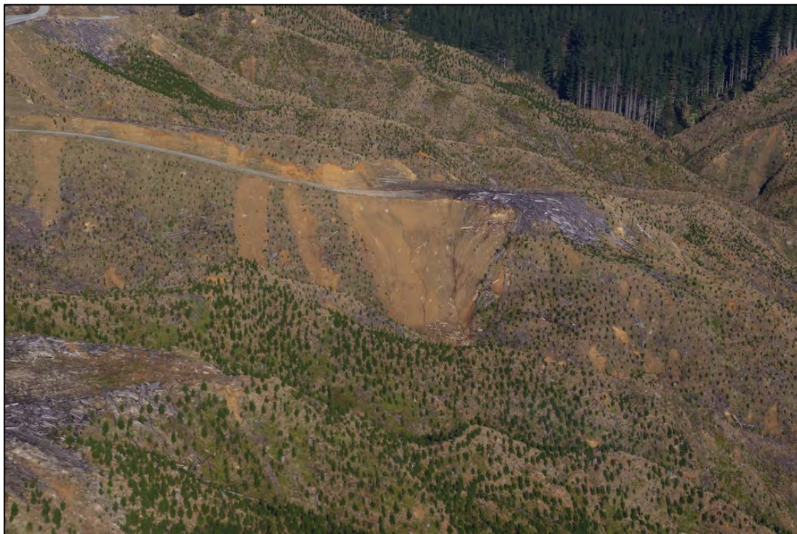
Figure Three Image 009A8790 looking west towards skid 8 (foreground) and skid 9 (middle ground). Both skid sites show skid edge failures which are significant at skid 9. The roadway to skid 9 also shows failure of sidecast material.
