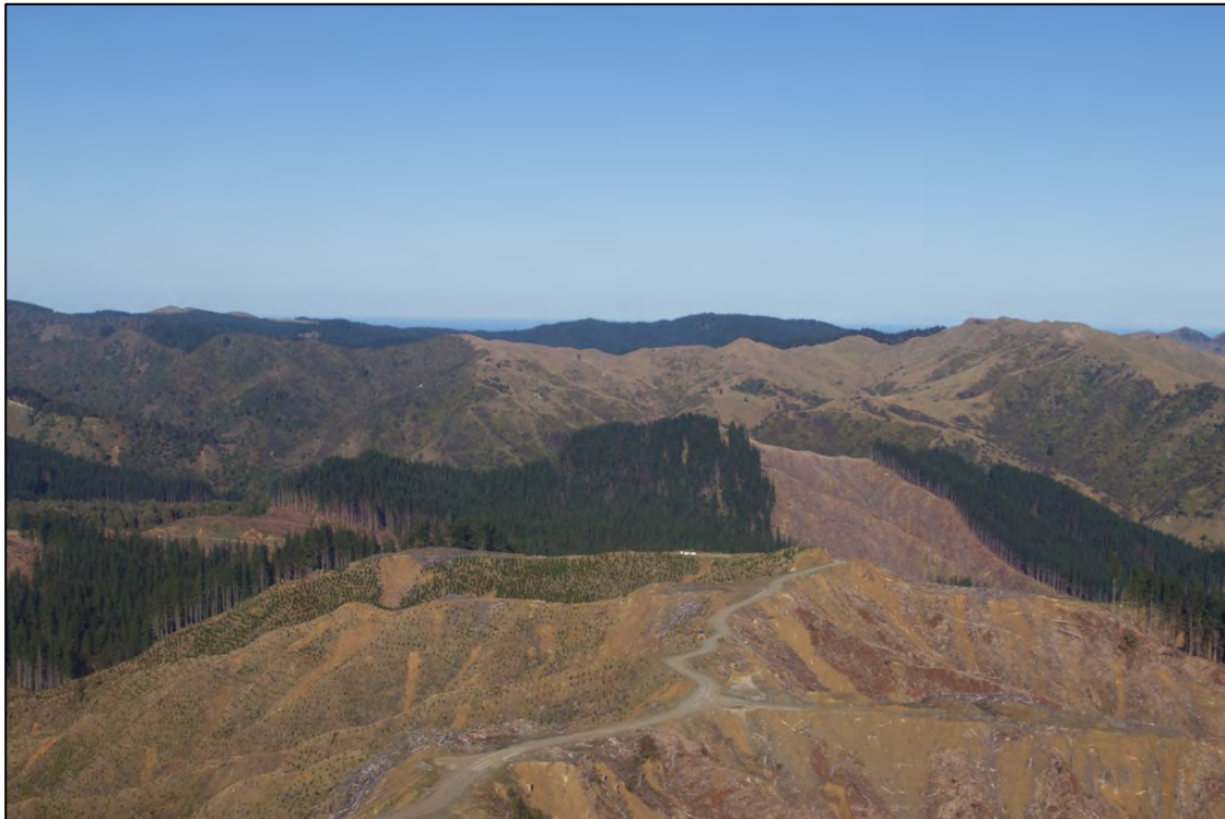
Figure Seven. View looking southwest towards skid 15 and beyond showing road edge failures, skid failures and failures from rough tracks on spurs.
