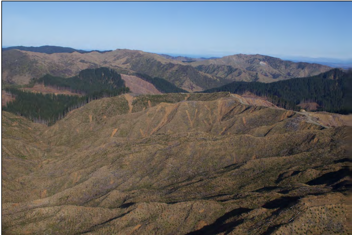
Figure Four. 009A8792 looking west towards skids 10, 11, 13, 14 and 15, showing slope failures from roadways (right), rough tracks (middle) and skid site (background left). A number a smaller mid slope failures are also evident.
