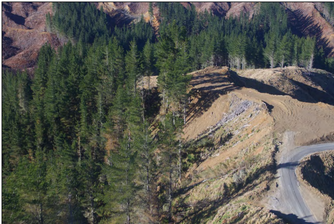
Figure Eighteen. View of skid 41 showing failures in side cast material.
