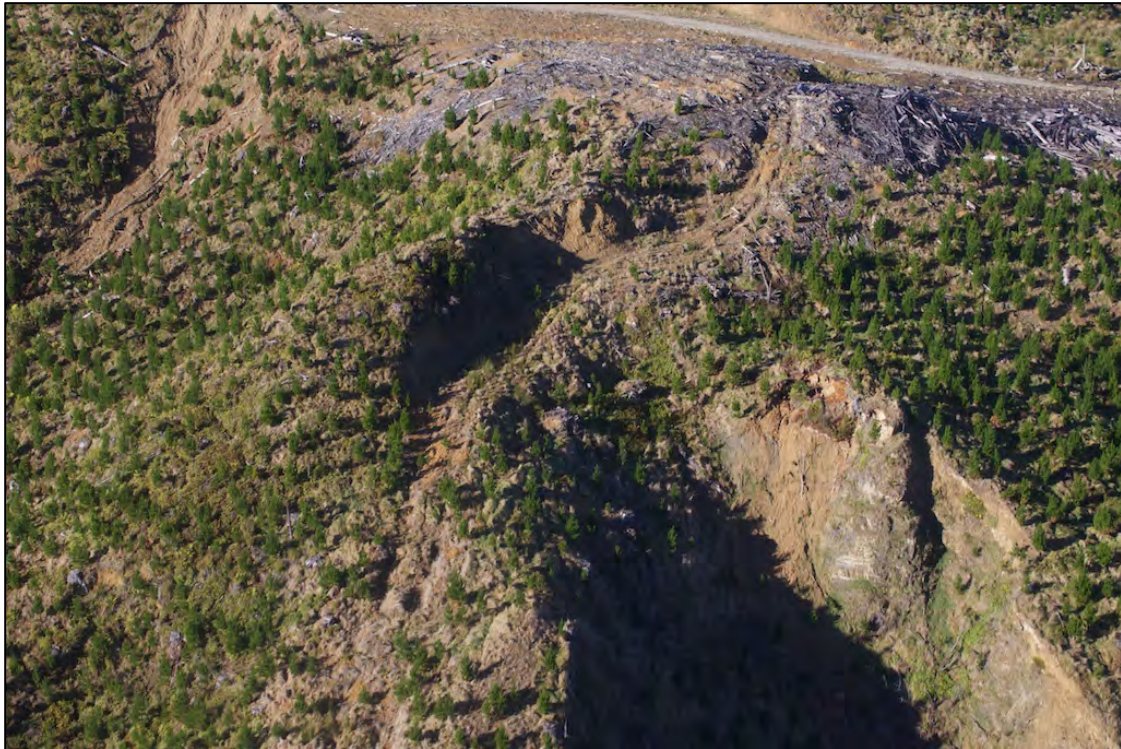
Figure Twelve. View of skid site 4 showing slumping from rough track cut through skid. Slope failure visible top left from roadway.
