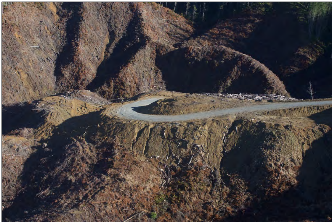
Figure Seventeen. View looking towards south showing rilling on sidecast material.
