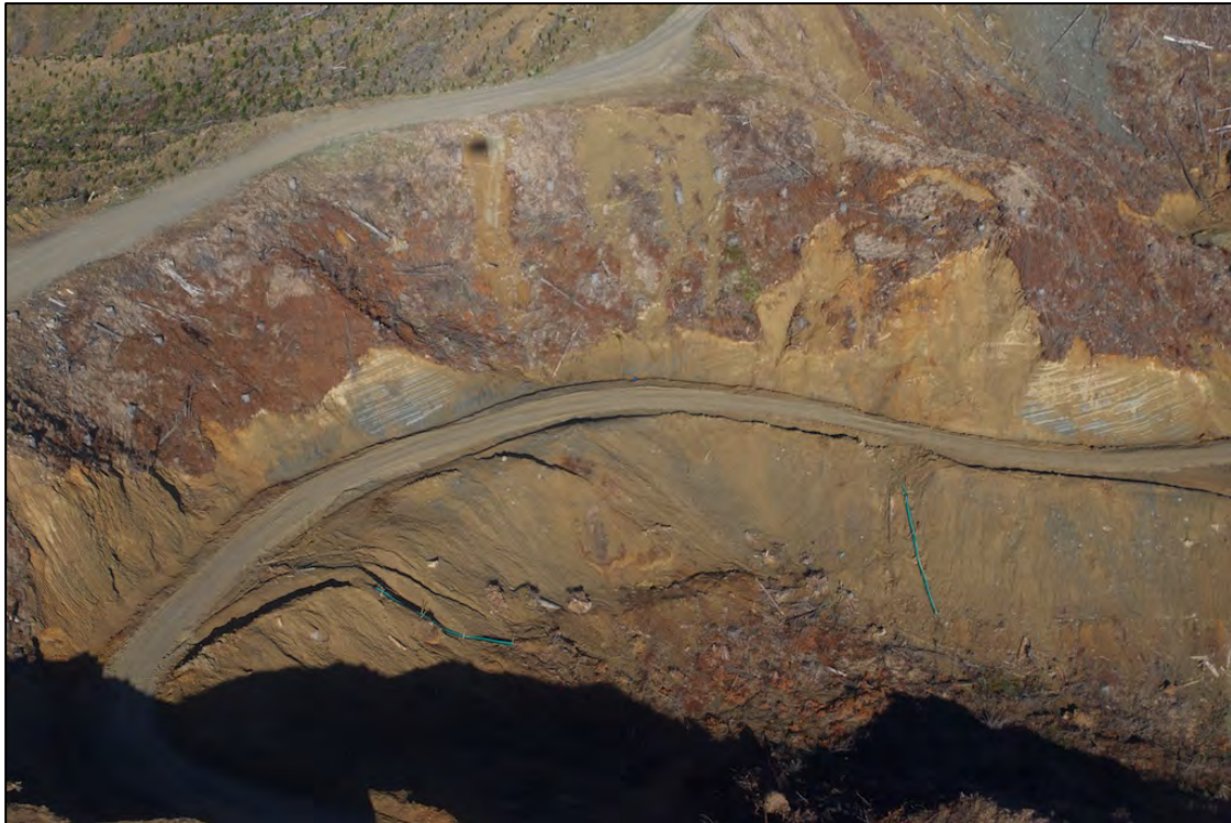
Figure Six View of Image 009A8795 looking south towards skid 11 showing flumes directing water onto sidecast material.
