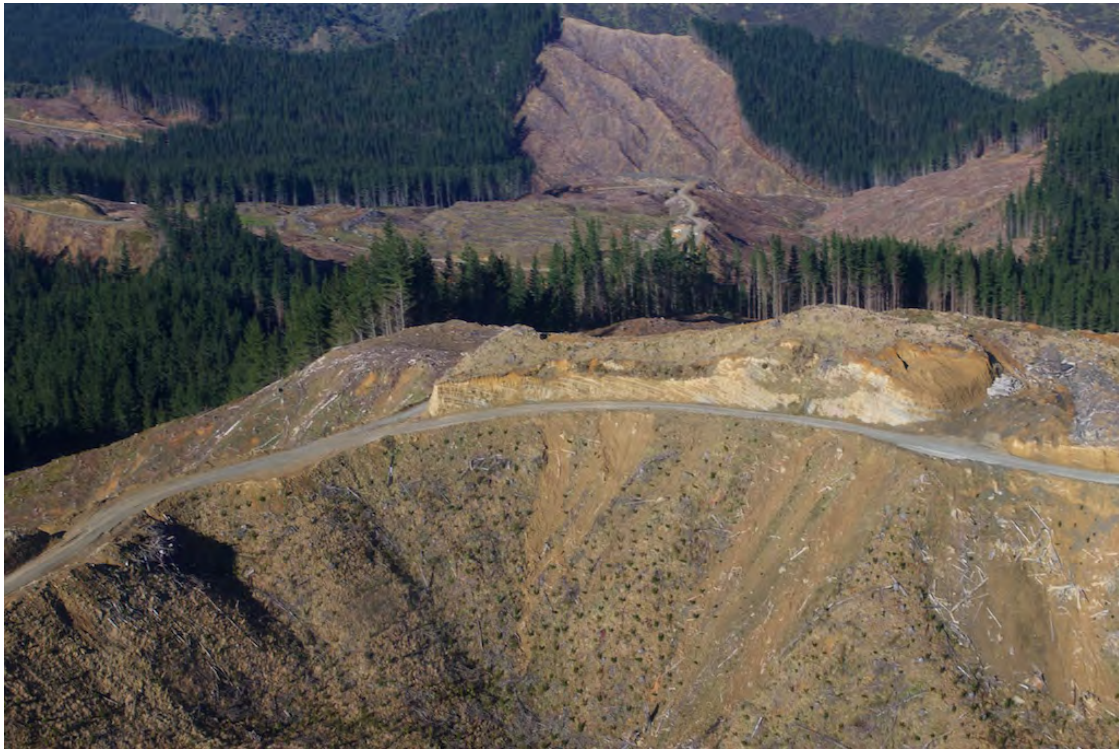
Figure Twenty. View of skid site 41 showing failures in side cast material from roadway.
