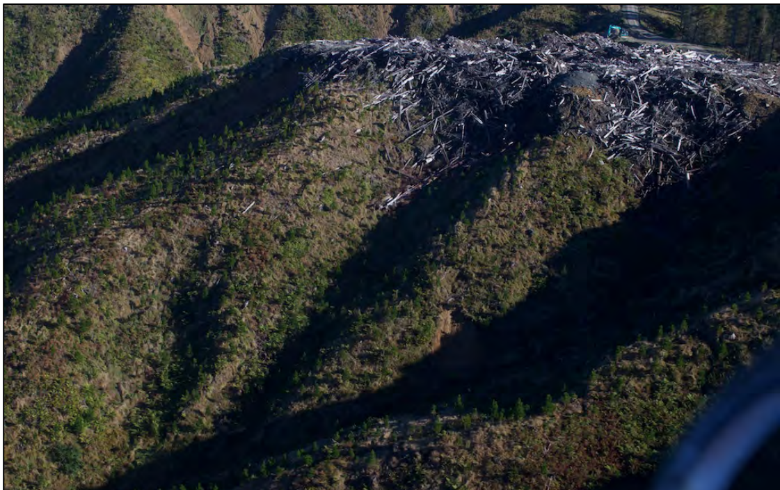
Figure Eleven. Image 009A8808 View of skid site 2? with woody material stowed on the edge of the skid with a collapse on the far right resulting in a debris flow and toe failure downstream.
