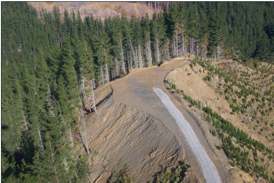
Figure Thirteen. View of new skid site showing extensive side casting with some slumping.
