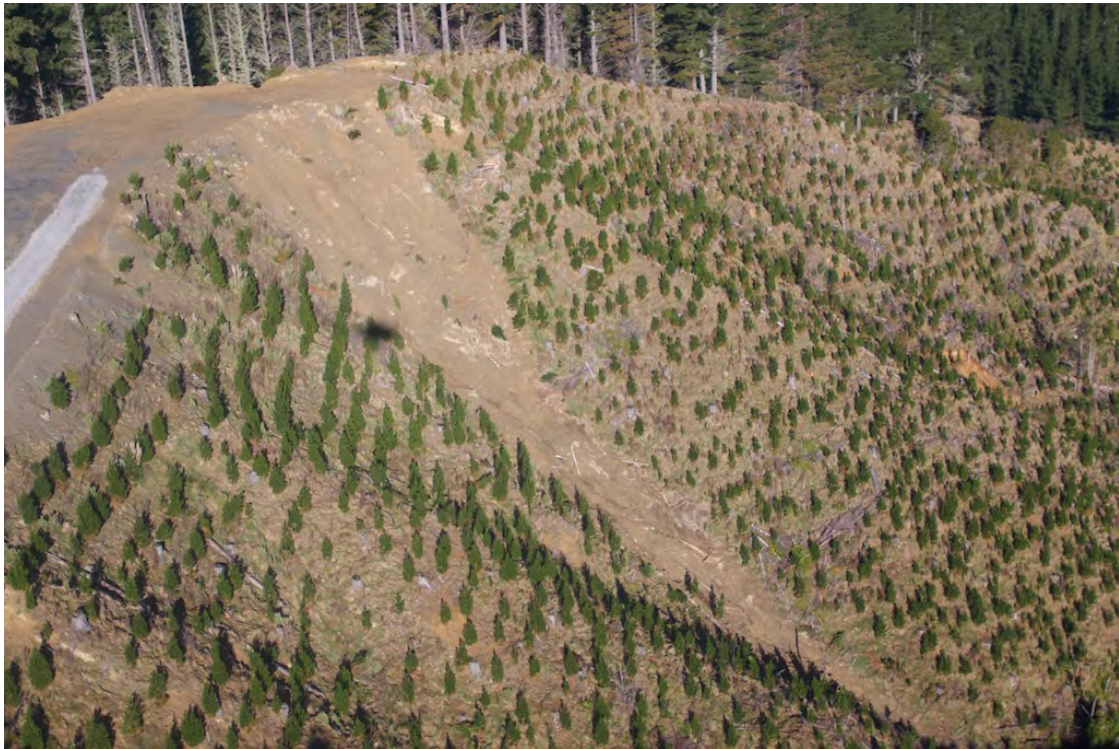
Figure Fourteen. View of new skid site (as in Figure Thirteen) showing failure on right hand side.
