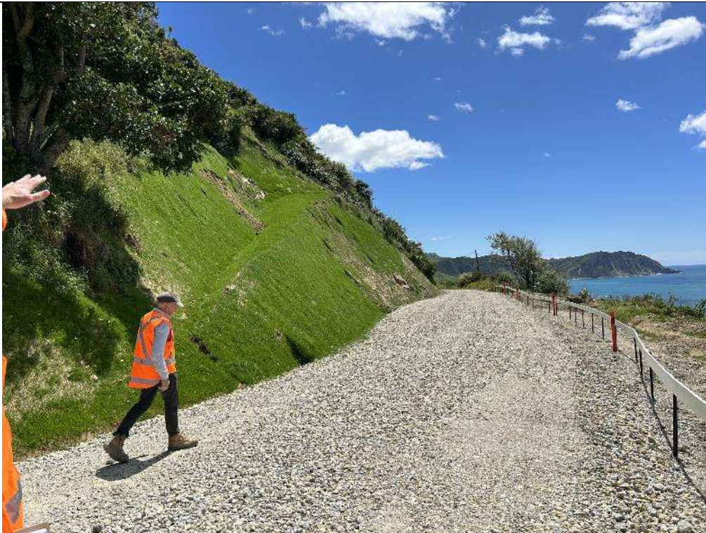
Photo 5: Large V drain and cut slope constructed and hydroseeded, shallow slope failures evident on steep faces. Road is 1.5m to 2.0m away from seaward cliff crest.
