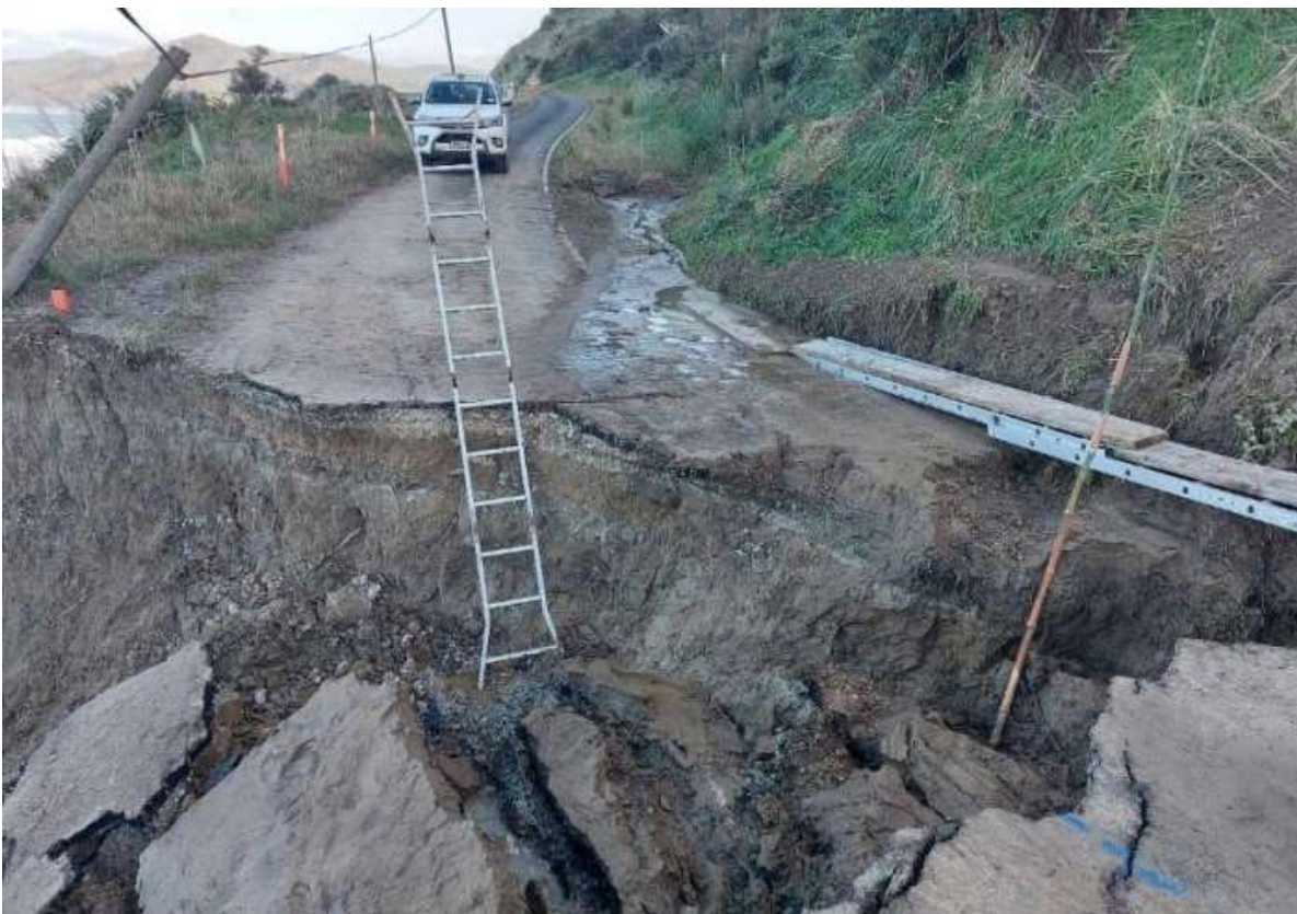
Photo 3: Photo taken by LDE showing the dropout at Waihou Road (temporary foot access created by locals)
