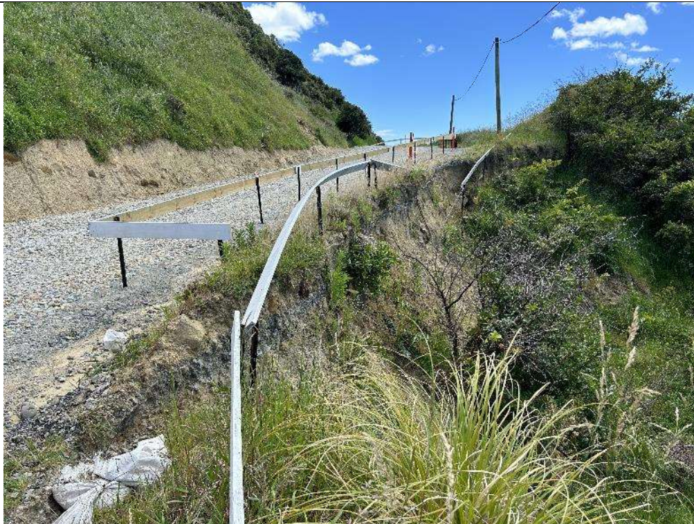
Photo 3: Sight rail reinstated above historic slip site (outside landslide feature extent discussed in this report)
