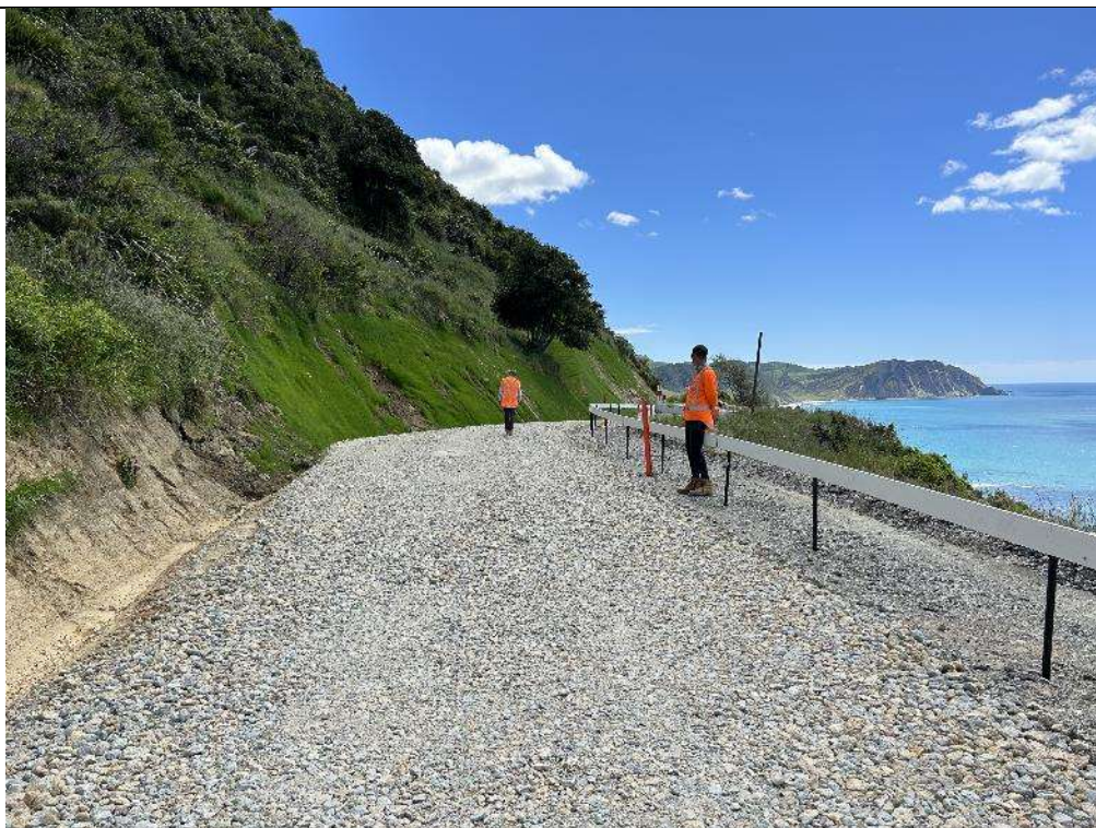
Photo 4: Road surface reinstated, road moved away from seaward cliffs, example of typical cut slope angles in the background recently hydroseeded.
