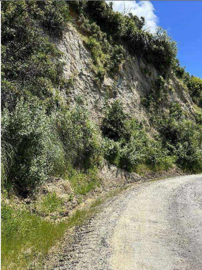
Photo 10: Cut slopes within similar material standing steeply just north of the site
