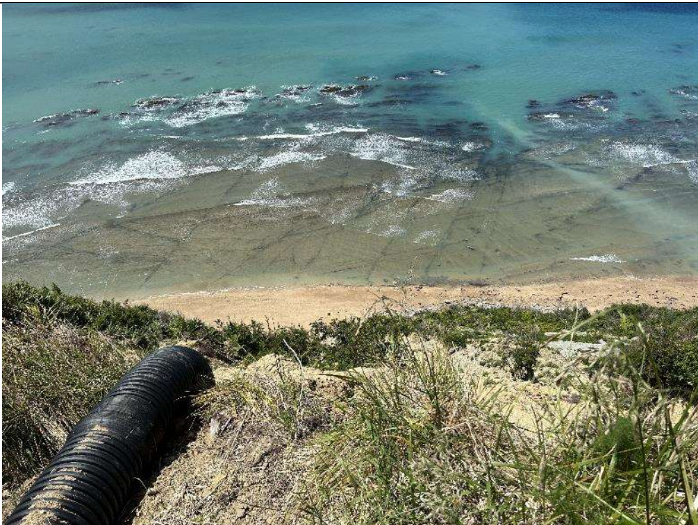
Photo 6: New culvert outlet with rigid flume over cliff edge.
