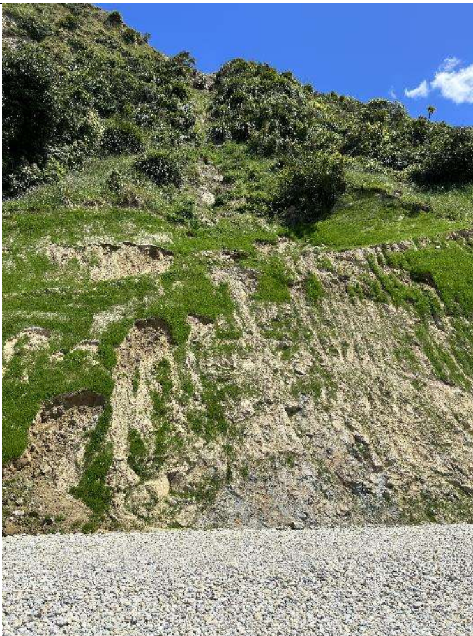
Photo 8: View towards source of debris flow, now directed by V-drain. Cut slope in extremely weathered sandstone/mudstone with surficial failures evident.
