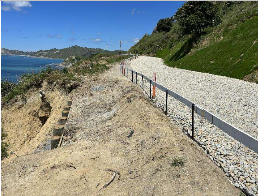
Photo 9: Road reinstated at drop out location, timber retaining wall at toe of reinstatement. Old culvert outlet visible in background, culvert is de-comissioned with no water outletting anymore.
