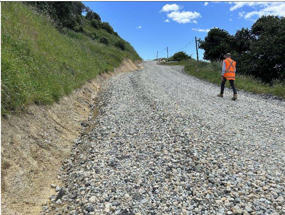
Photo 2: Road surface reinstated, minor excavation into landward slopes to form drainage channel
