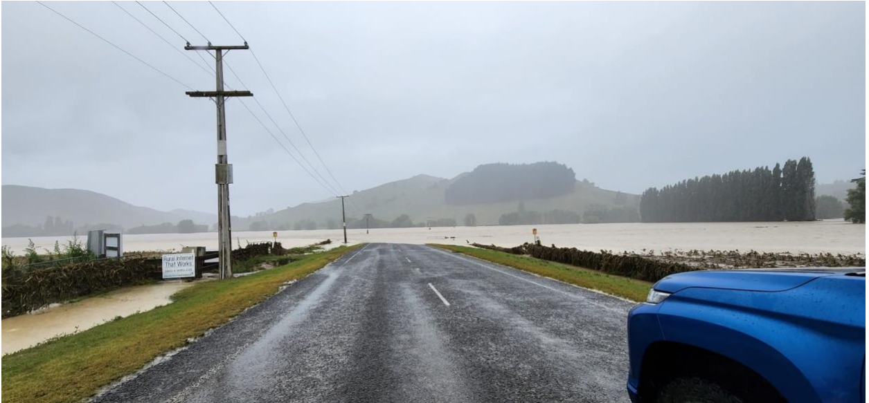
7. Whatatutu Road cut by floodwater. Cyclone Gabrielle, retreating water
