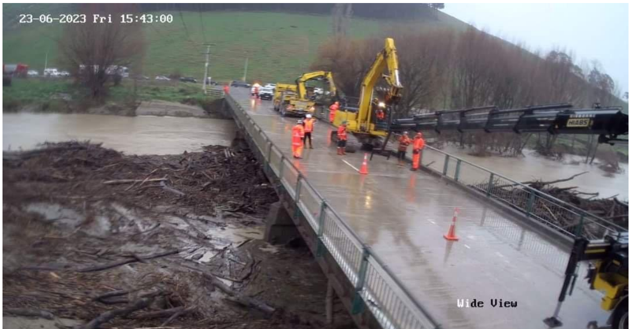
5. Contractors clearing wood debris from the Whatatutu Road bridge, 23 June 2023
