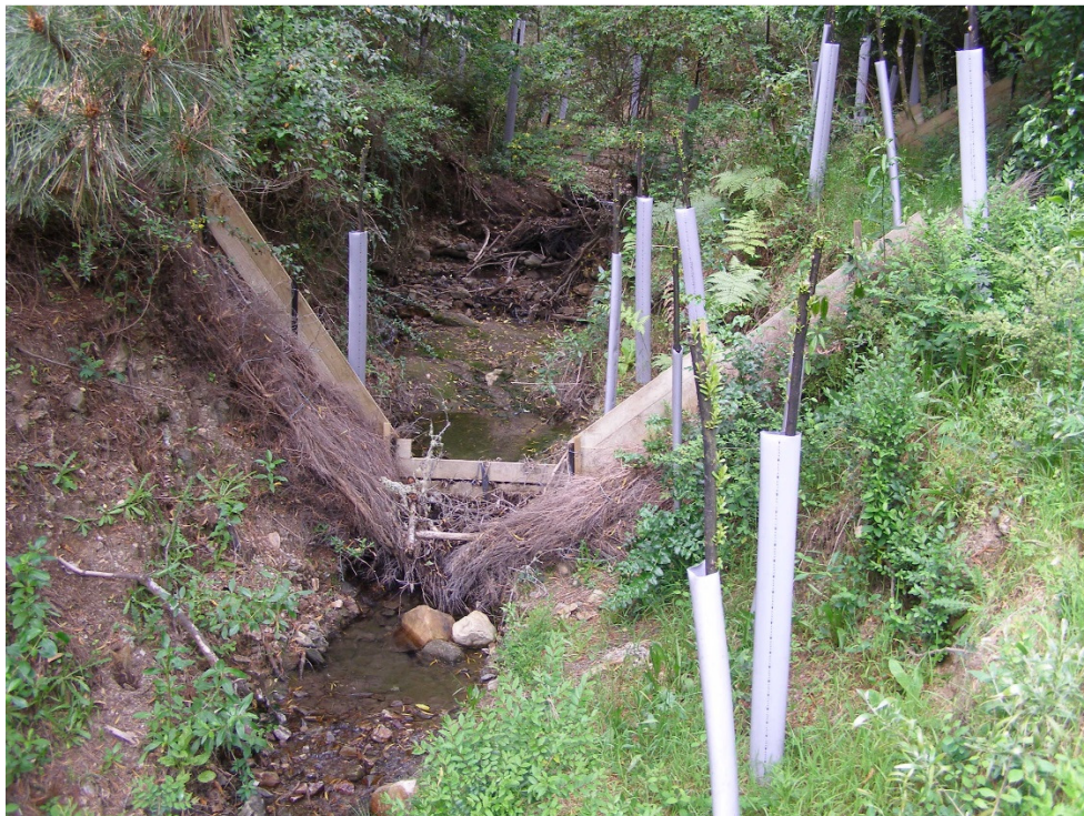
Fig. 4: Dam No. 5; Photo: D Peacock, 17 th October 2017.
