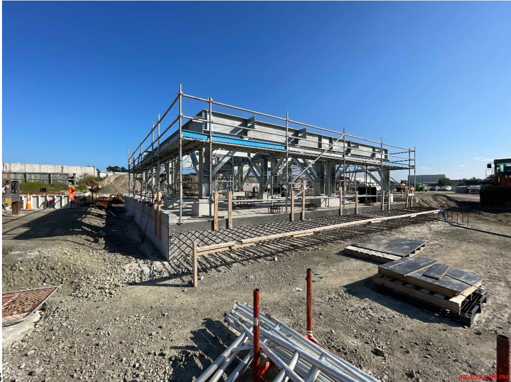
Scaffold around lamella clarifier frame being constructed.
