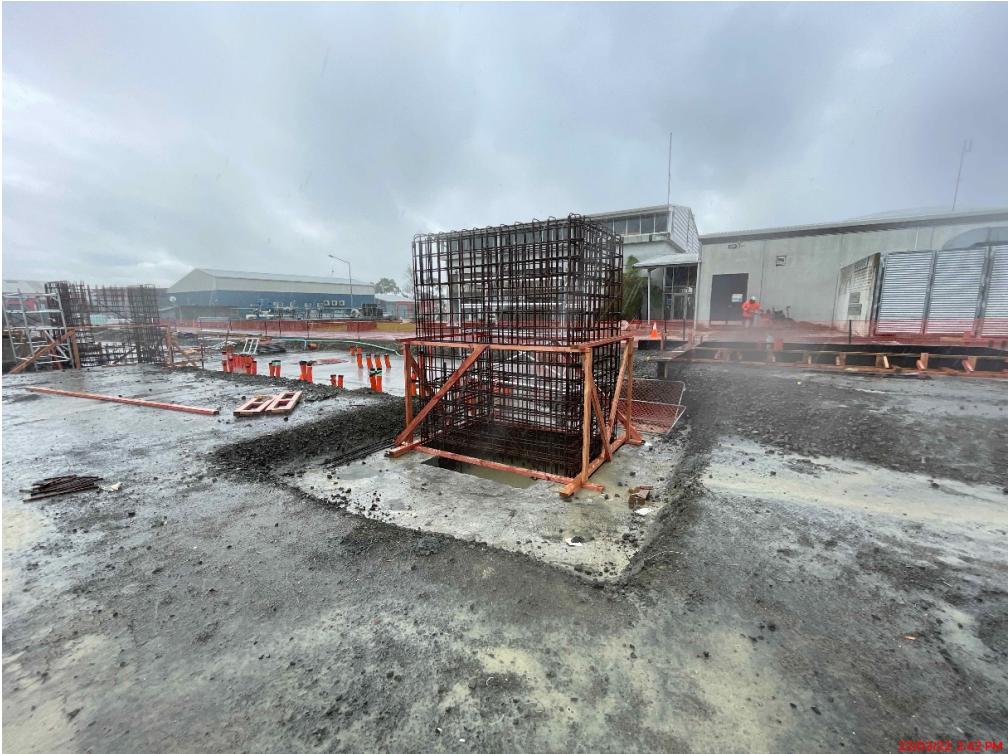
Reinforcing construction of UV treatment chambers.
