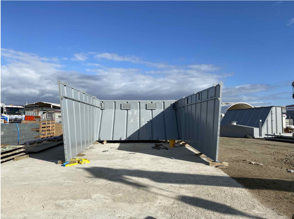
Pre-assembly of lamella clarifier upper hopper walls.
