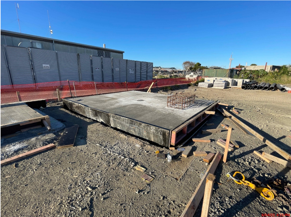
Pump shed slab poured.
