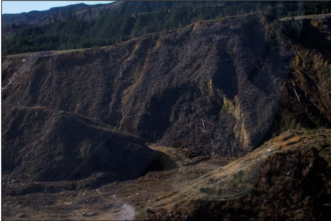
Figure Twenty. View of slash on slope at skid site on Bottom Road (left) with failure from skid site (partially obscured) on far right. Note volume of logs on valley floor and slips from the roadway in the middle ground.
