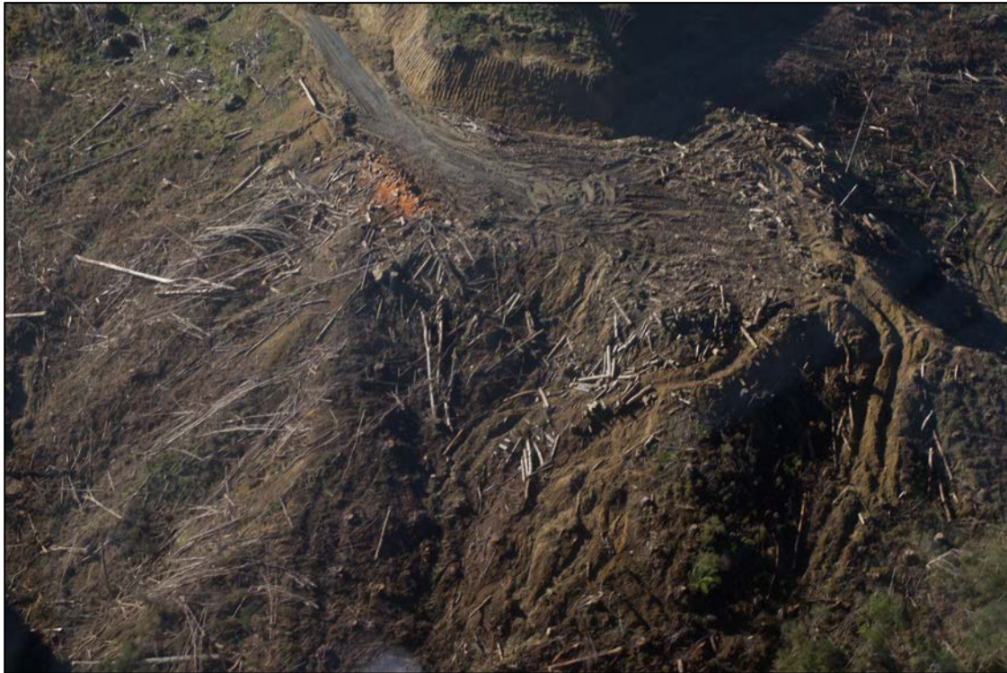
Figure Four. View looking east showing a skid site looking east showing a slope failure from a drainage channel cut at the edge of the skid site and generally messy housekeeping.
