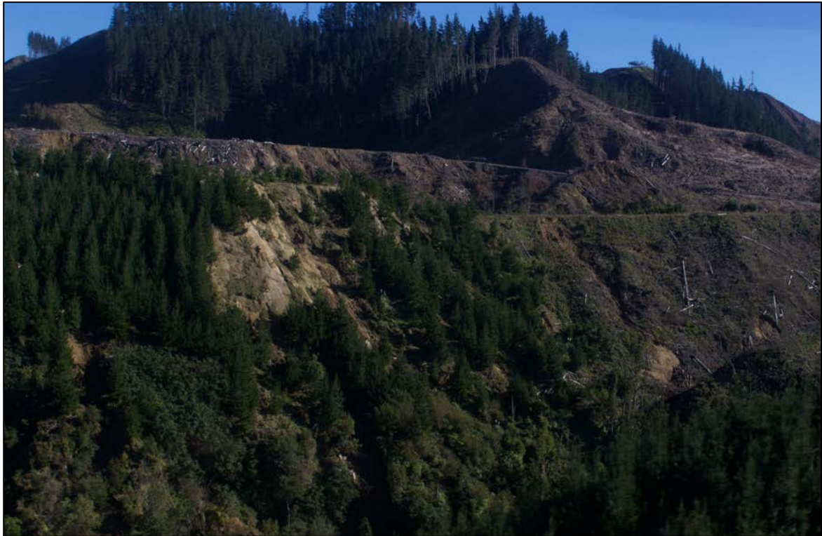
Figure Eleven. View looking north into the western end of the early harvest area in Wakarua Forest. At the far left a slope failure from the roadway has generated a debris flow which has migrated through 5+ year old pines towards the valley floor. Additional failures down to the rock base have also occurred from what appears to be a bench or rough track while on the right there is a slope failure from the edge of the roadway.
