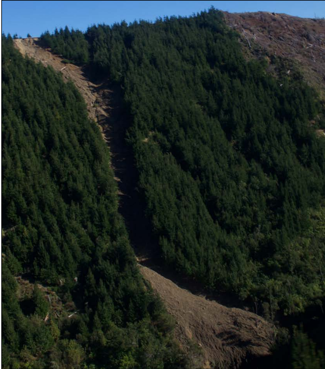
Figure Seventeen. View looking west of major debris flow from Goat Road.
