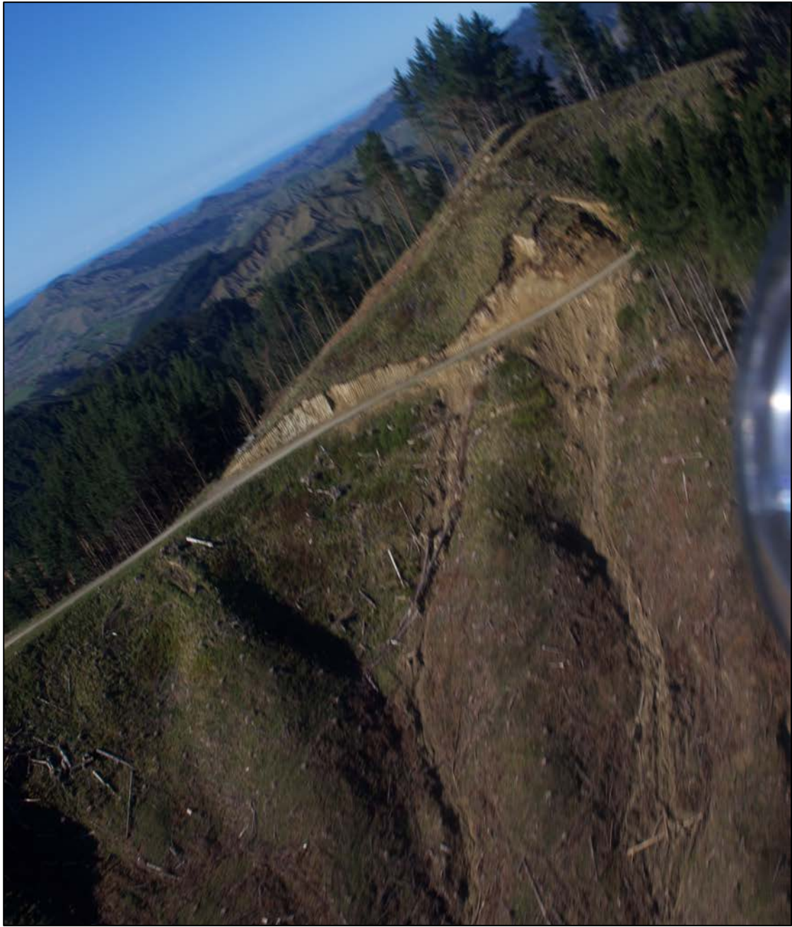
Figure Seven. View looking east showing two failures in side cast material originating from a roadway.
