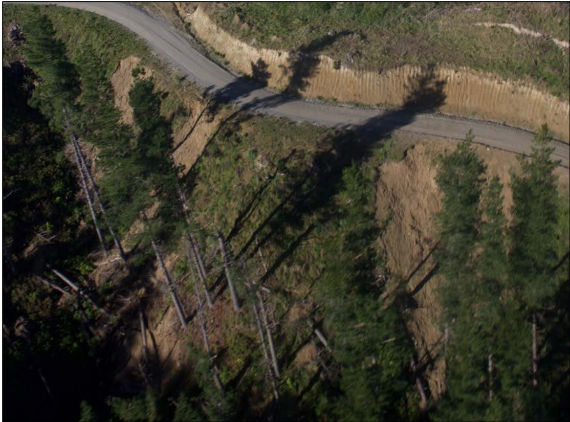
Figure Eight. View looking east towards several slope failures originating from a roadway.
