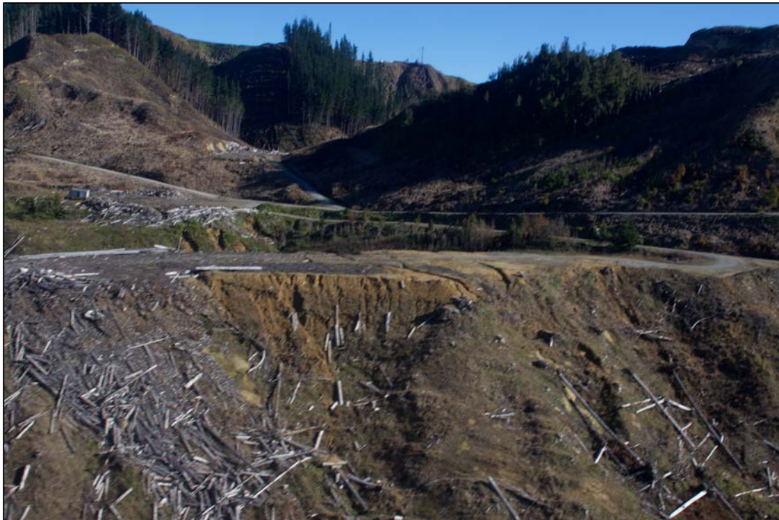
Figure Fourteen. View looking northwest towards a skid site on a spur off Bottom Road showing significant logging debris on the slopes and pronounced rilling in sidecast material.
