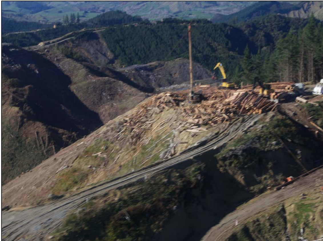
Figure Six. View of operational log hauler operation (blurred) showing two significant failures from the edge of the site.
