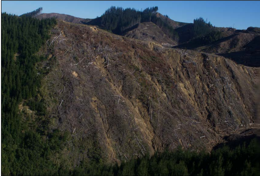
Figure Eighteen. View of slope failures on Goat road north of Figure Seventeen. On the right is a major failure where the edge of a skid site has failed, while on the left “mid slope” failures appear to connect to the valley floor and could be toe failures. On the right are “midslopes” clearly connected to the valley floor and thus most likely toe failures.
