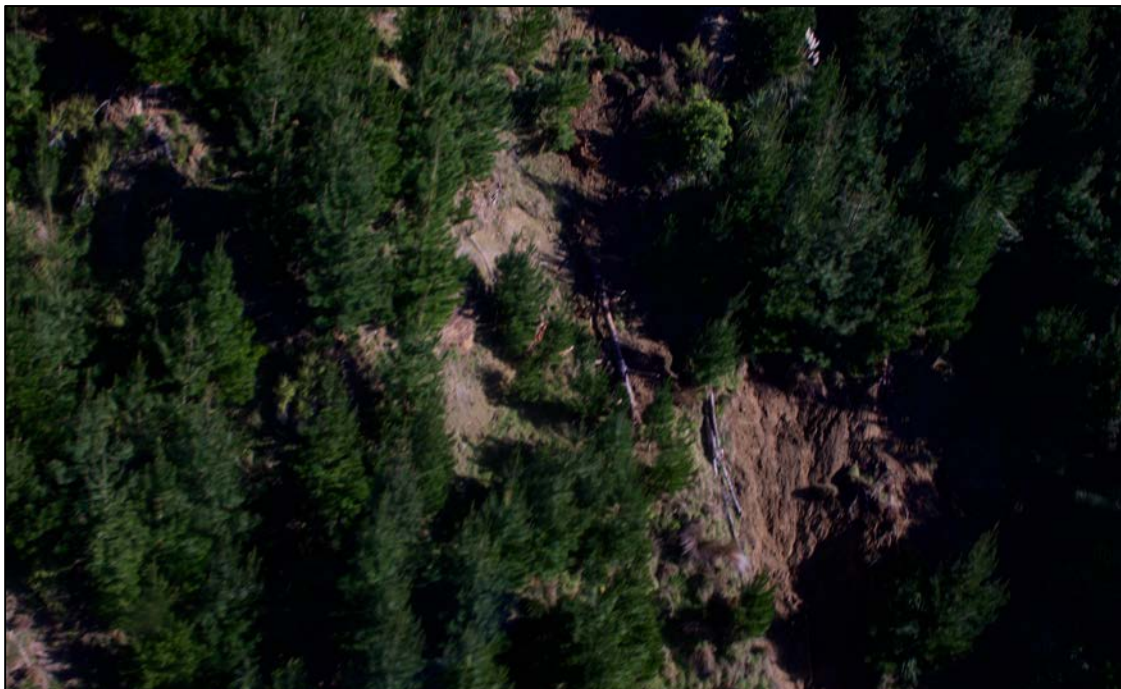
Figure Twelve. Detail view of the failure shown in Figure Eleven showing the path of the debris flow middle left and a subsequent failure on the right resulting from toe failure.
