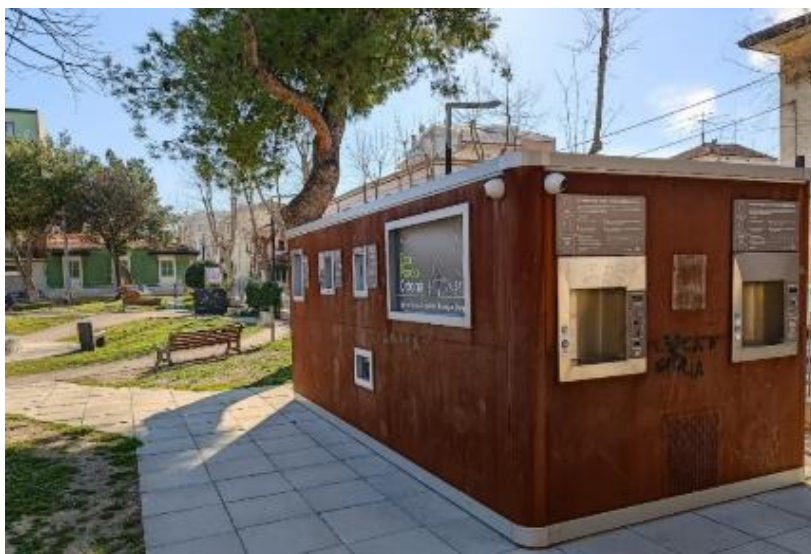
Figure 13 Ecologic Island in a playground in the city centre
