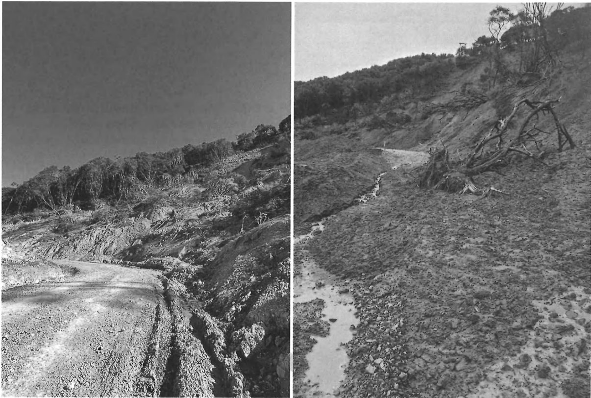
Figure 4-3: Slip across Anaura Road looking south, left image taken 28/08/23, right taken 25/09/23
