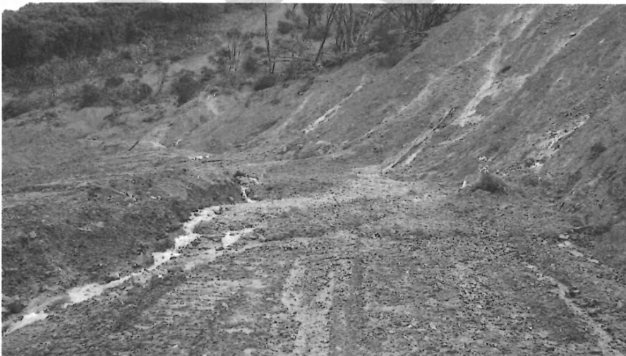
Figure 4-2: Photo of slip site after/during rainfall, facing south. See channels of water flowing down hillside and down Anaura Road.
