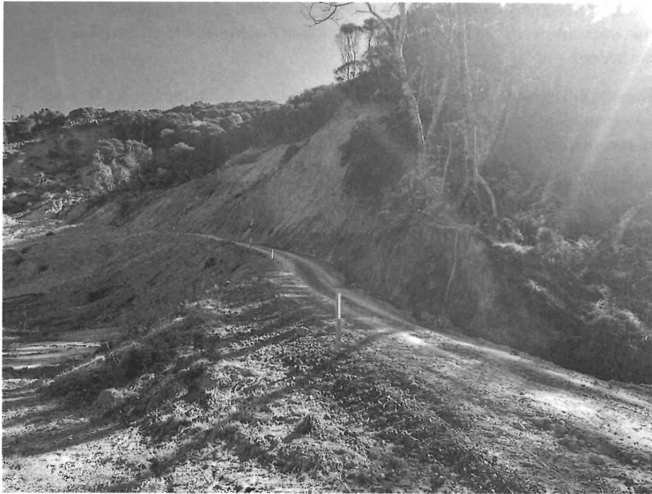
Figure 4-1: Northern Approach to Problem Area (facing south)
