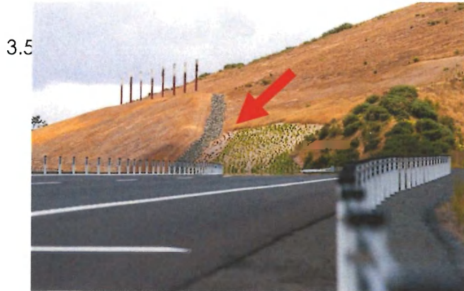
Figure 2: Cutoff drain example
