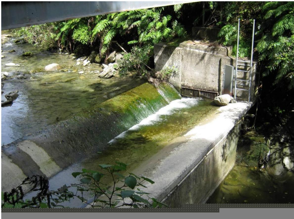
**Figure 2** Municipal water supply intake structure at Waterworks Bush
