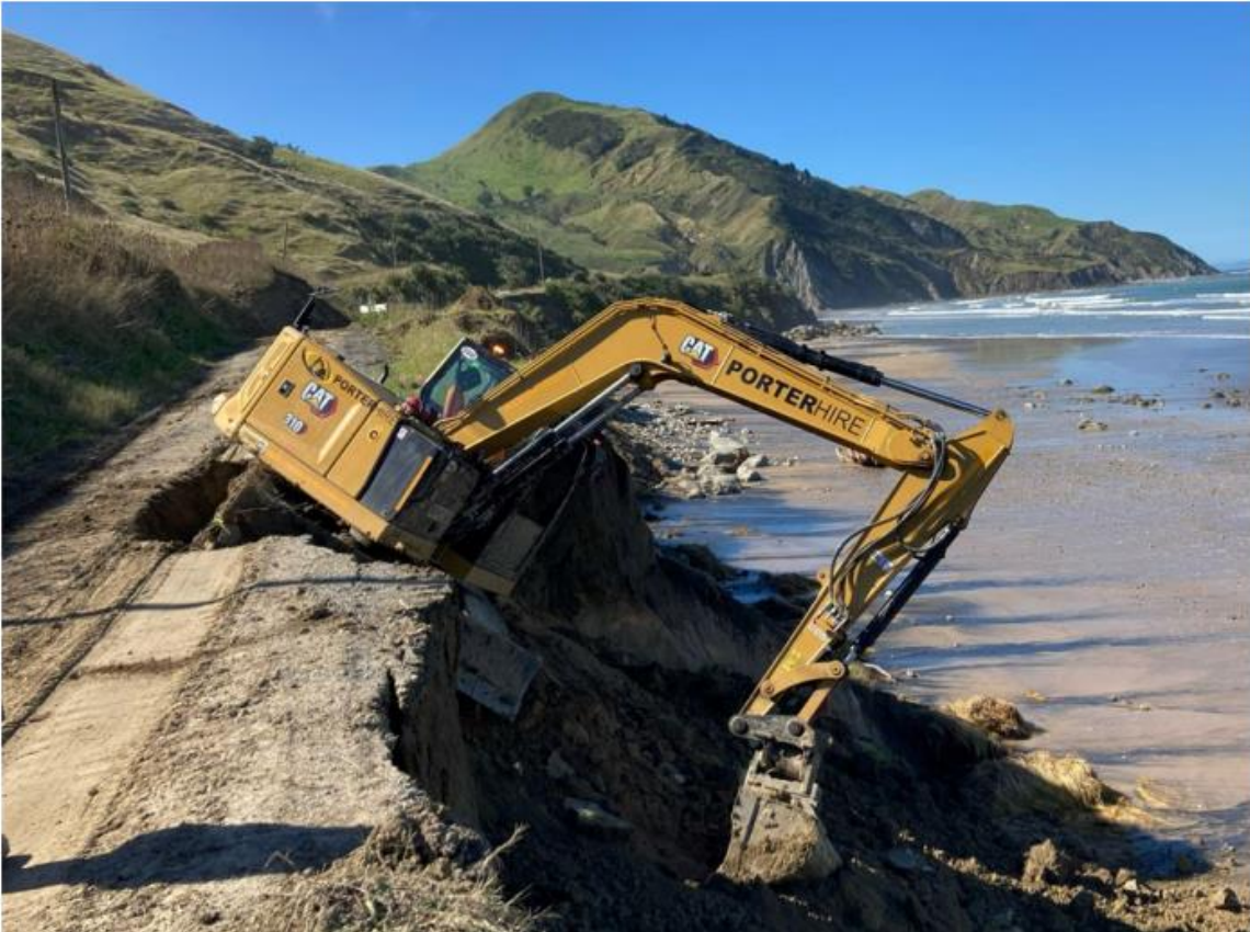
Below is a section of Kaiaua Road that has collapsed. This is due to a tomo (dissolved hole) under the road, created by the high sea hitting the sand dune face. The road collapsed under the weight of the digger.
