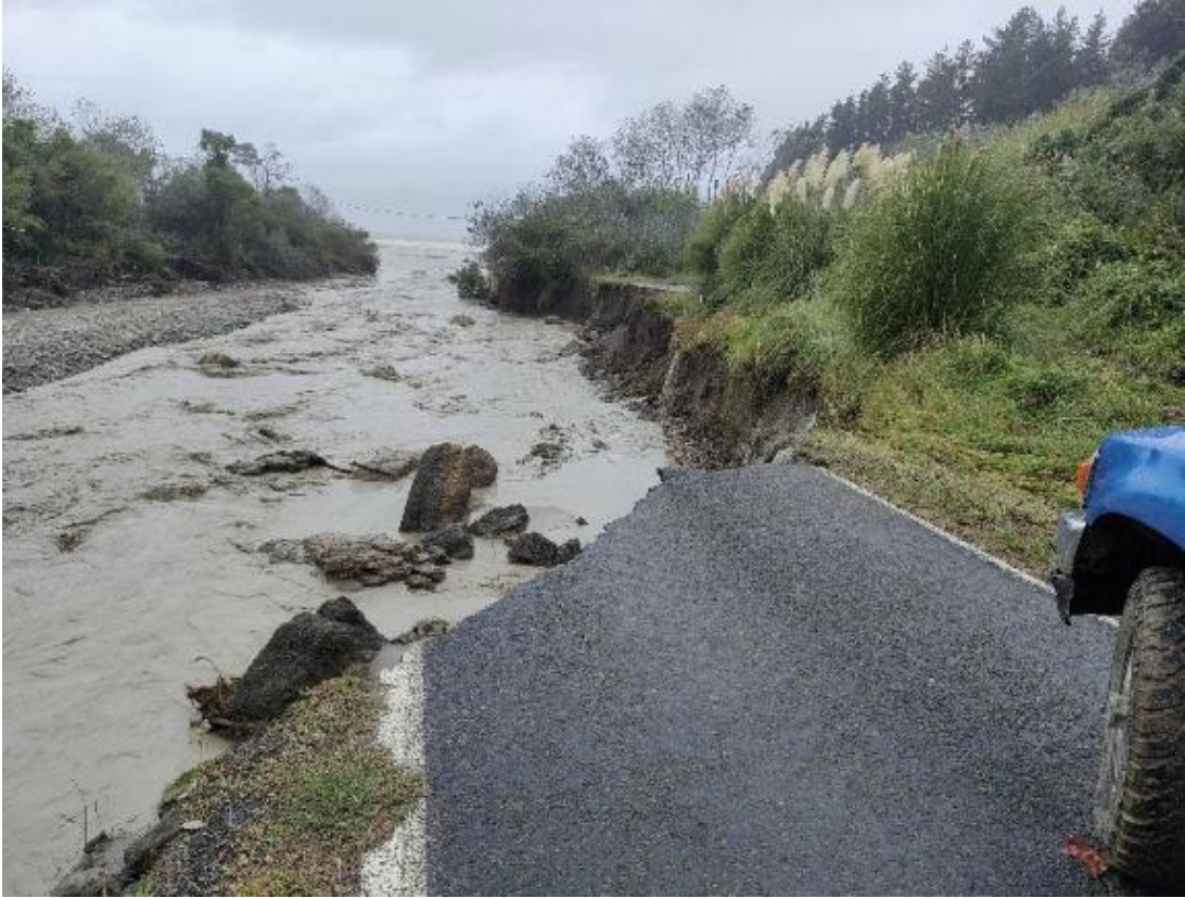
Below is a section of Kaiaua Road that has collapsed. This is due to a tomo (dissolved hole) under the road, created by the high sea hitting the sand dune face. The road collapsed under the weight of the digger.
