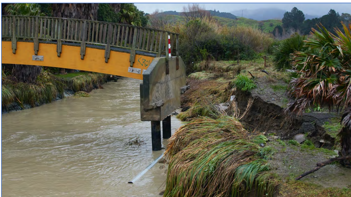
Figure Forty Nine. The washed out abutment of the footbridge at the mouth of Waiotu Stream.
