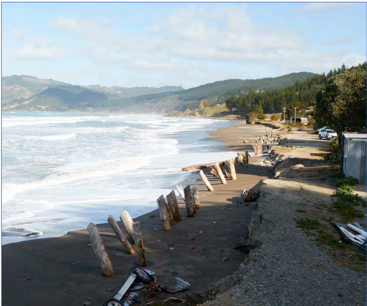
Figure Sixty Two. The extent of recent coastal erosion at the northern end of McIlroy Road marked by the pine logs that had been pushed into the sand as retaining posts.
