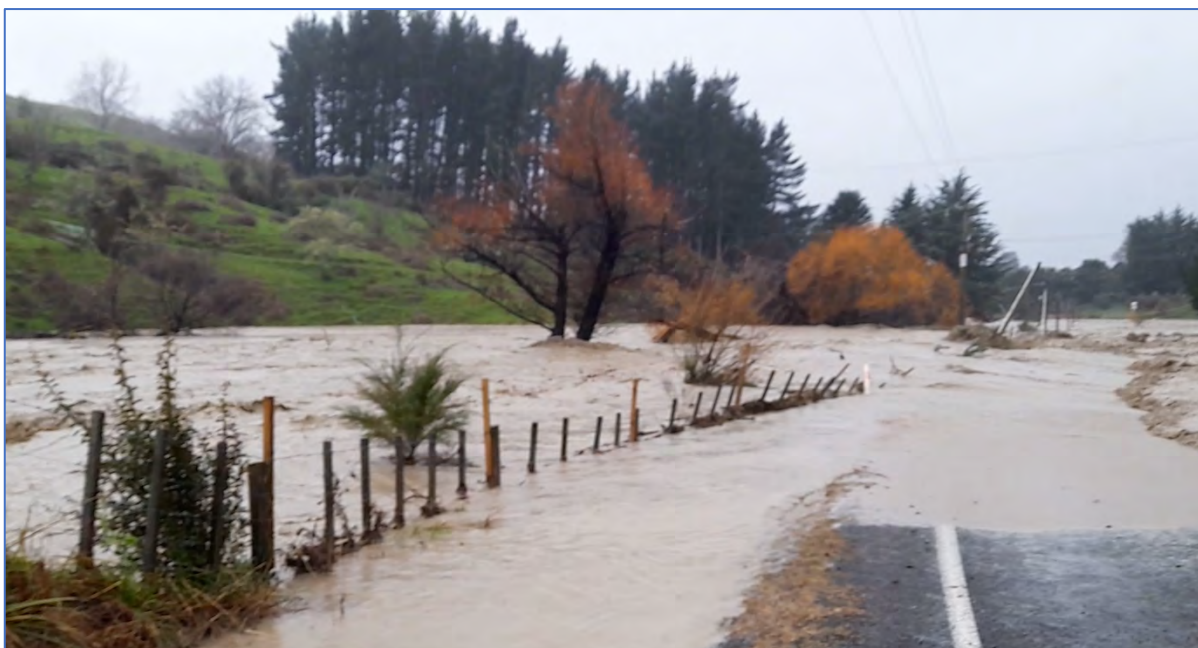
Figure Forty Two. Video still provided by Tianna Rongonui showing the flood spread and with the large willow in the river in the background. As can be seen the flood spread was considerable wider than the normal river banks at point and had occupied the entire flood plain.
