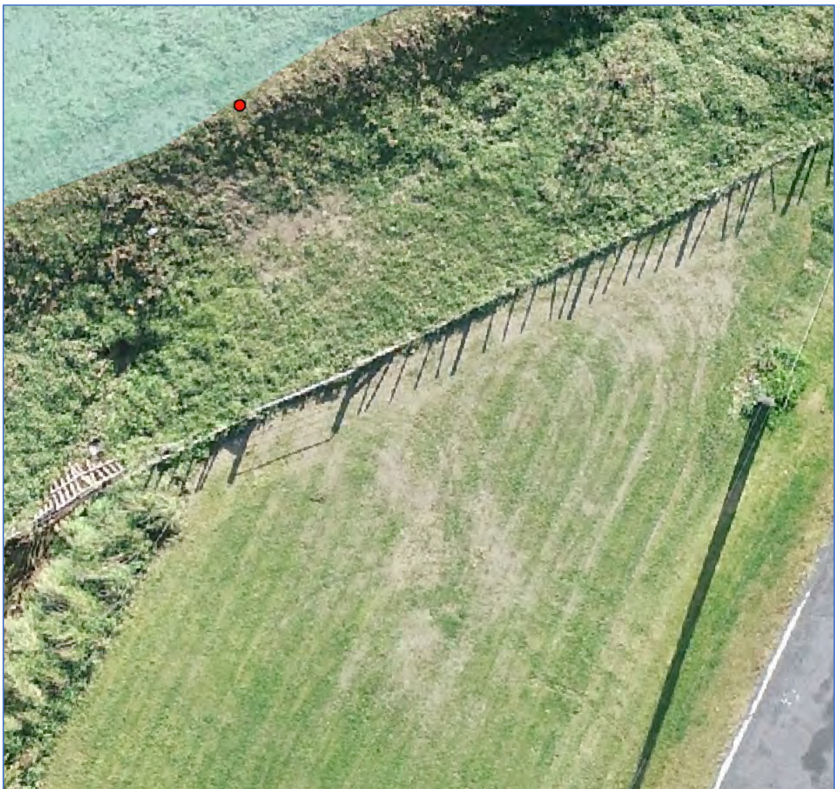
Figure Fifty Eight. View of the lower overtopping point showing the silt deposition extending out onto the low lying ground beyond. The imagery does not, however, suggest flood spread beyond 18m of the overtopping point.
