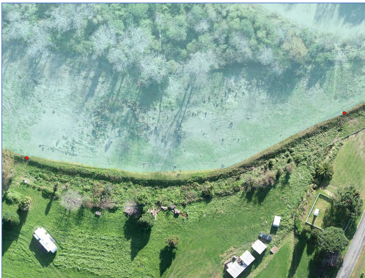
Figure Fifty Six. View of the lower true right bank of the Mangahauini showing the two overtopping points. The old road is shown at far right.
