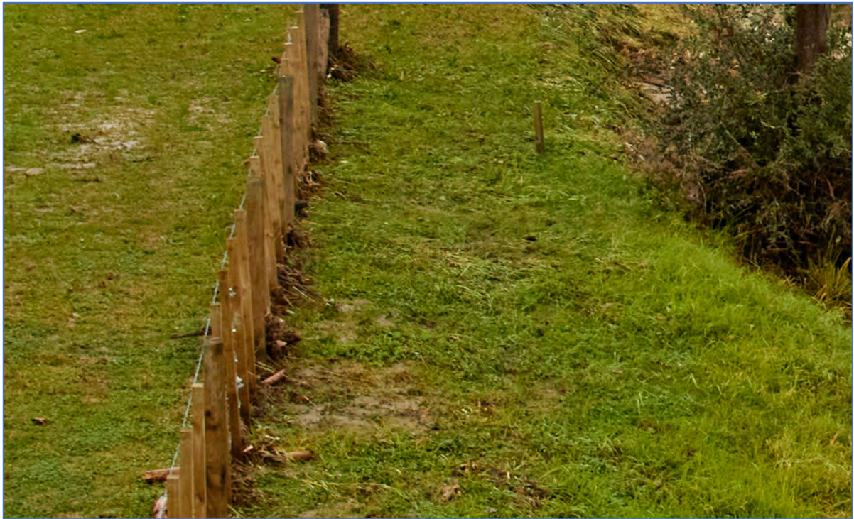
Figure Thirty Five. Fence at top of bank of Kaiawha Stream upstream of the SH 35 Bridge showing woody debris caught up in fence and mud deposited on the river side of the fence.
