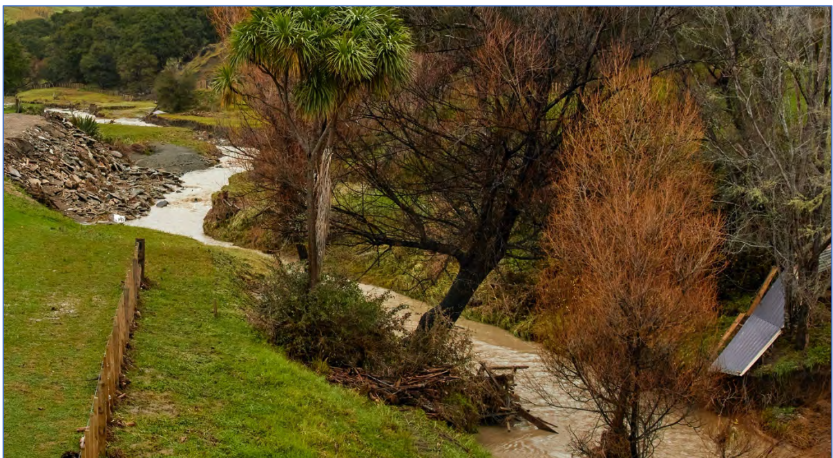
Figure Thirty Four. Kaiawha Stream upstream of the SH 35 Bridge showing the damaged debris fence and woody debris caught against the trees.
