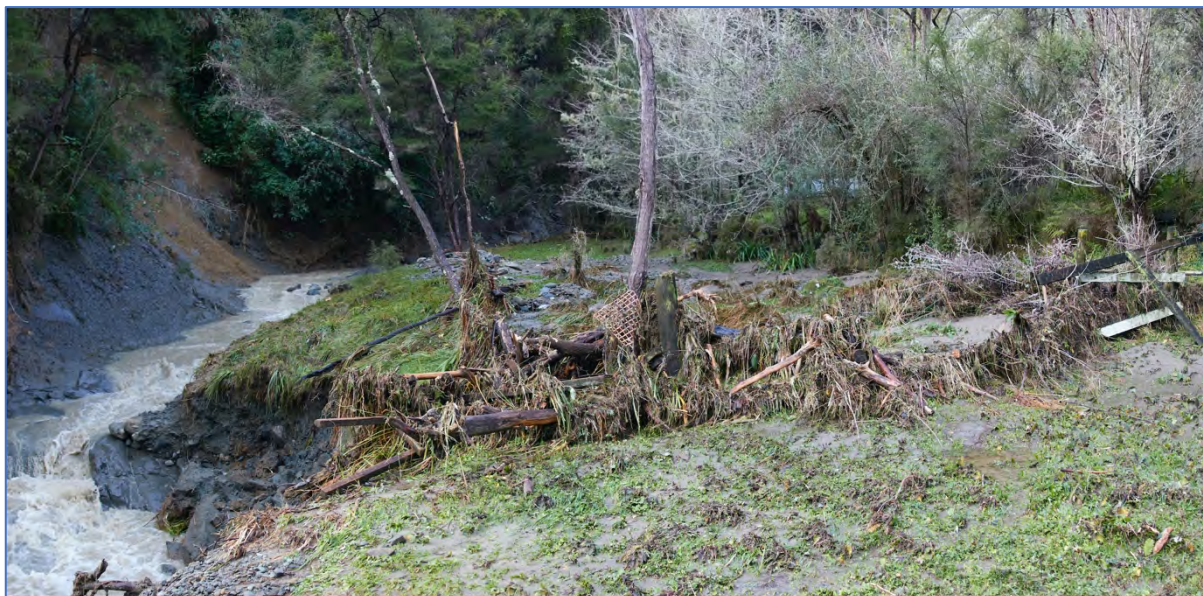
Figure Thirty Seven. Photograph upstream of the ford on Kaiawha Road showing the extent of flooding upstream of the ford on the Kaiawha Road.
