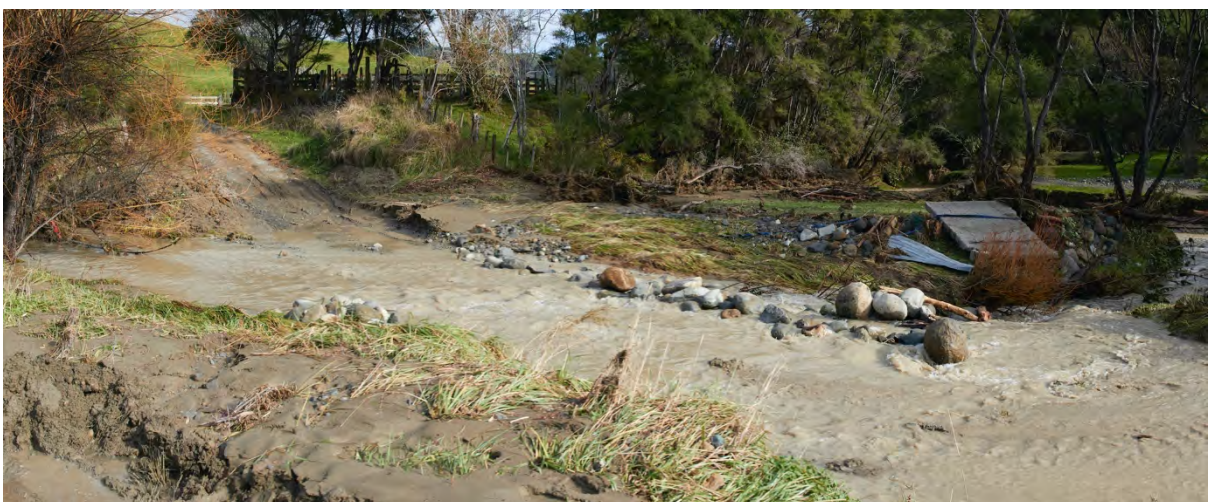
Figure Thirty Six. Photograph of the ford 650m upstream of the bridge on State Highway 35 showing the depth of silt deposition (bottom left), the height of the flood spread based on the debris layer and the mobilised boulders on the ford path.
