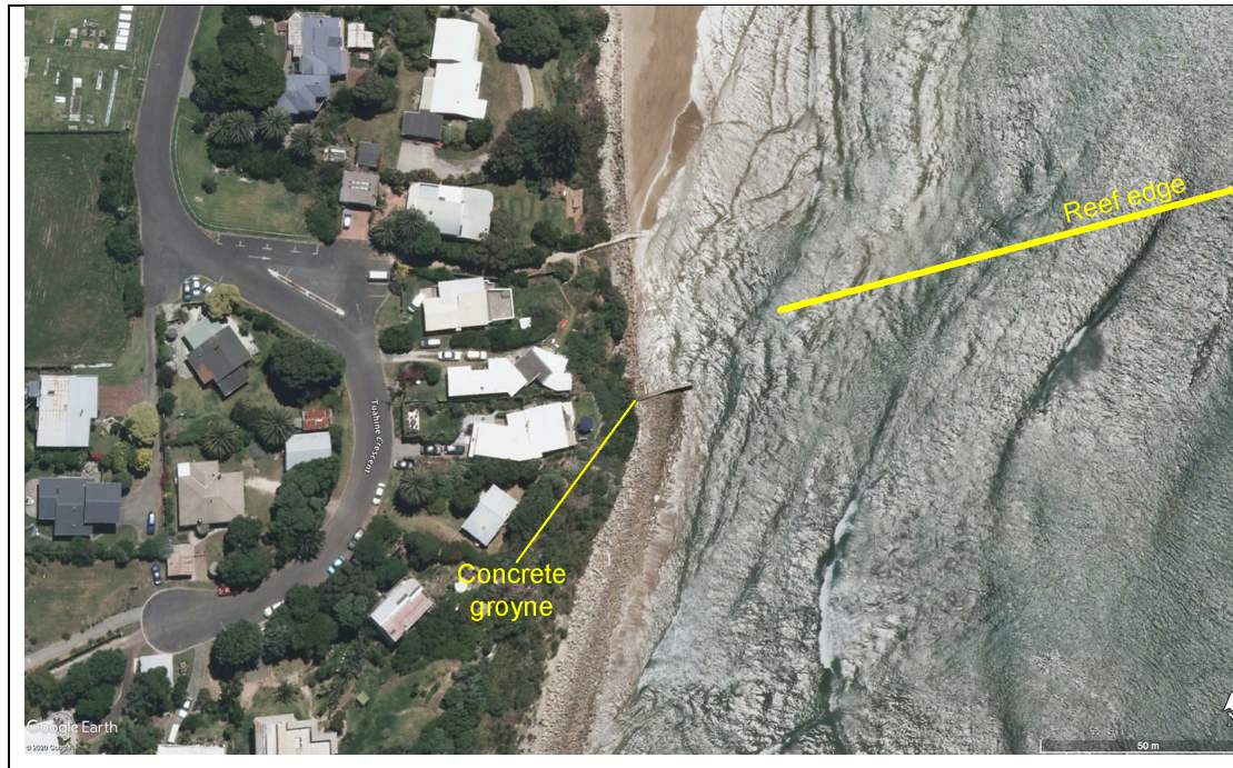
Figure 1 – Google Earth image of Tuahine Crescent showing the pattern of incident and reflected waves interacting with the bathymetry and shoreline structures. The existing concrete groyne is labelled, and a rock revetment seawall is present along the length of the shoreline shown. A rocky reef occurs south of the reef edge marked on the image, with sand dominating north of the line. The boundary appears to be a fault, with the southern side upthrown relative to the north.
