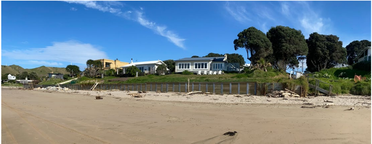
IMAGES OF REINSTATED SEAWALL 22-26 PARE STREET (August 2022)
